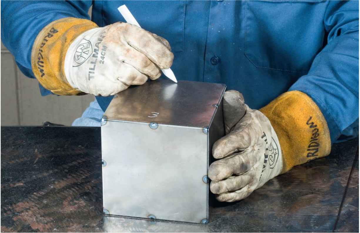
Use a marking tool to indicate the location of tacks, welds, and features such as drilled holes.
