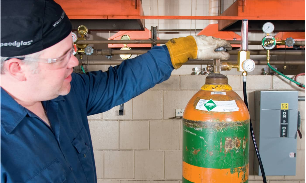
Open cylinder valves slowly to avoid damaging regulators and flow meters.
