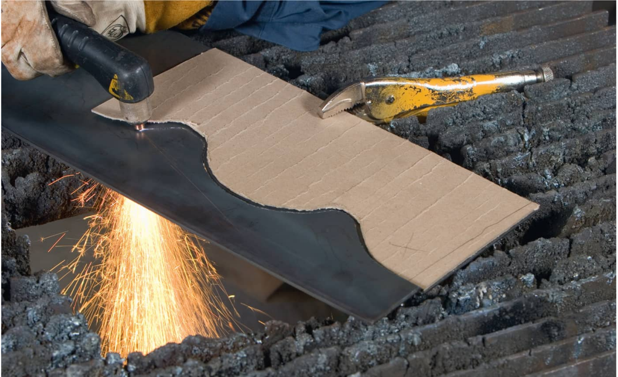
Cardboard or plywood templates work well for plasma cutting odd shapes.
