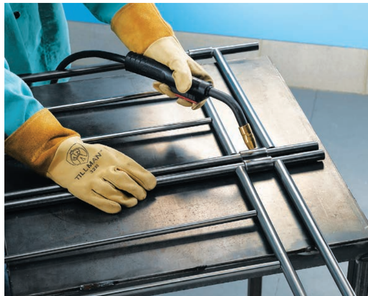
Align the hinge barrels and weld them together.
