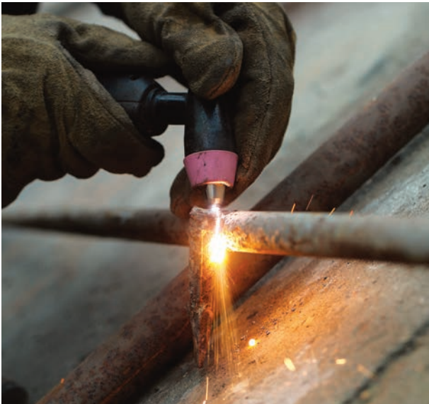
Cutting pipes is a cinch with an electric plasma cutter.
