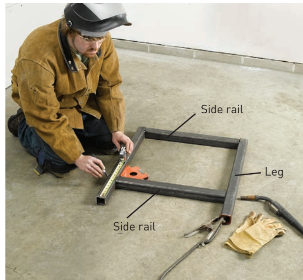
Align the side rails in between legs. The side rail part is 6" up from the leg bottom. You will make two of these side frames and then add front rails in between the sides for the front and back of the table base.
