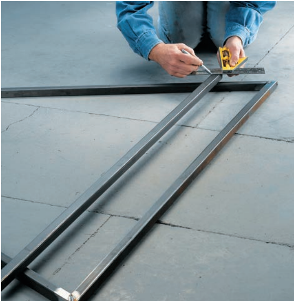
Mark the roof crossbar for cutting.
