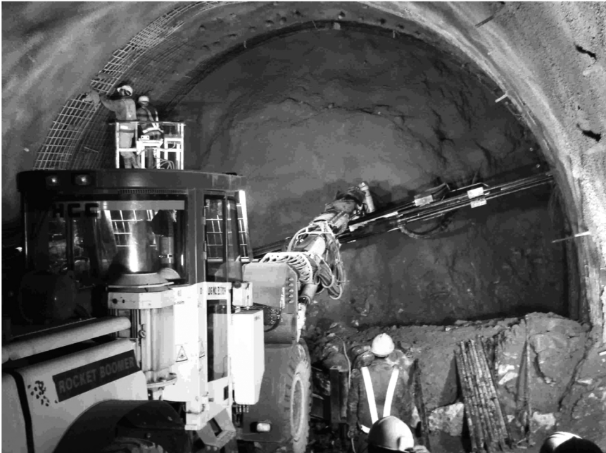
Figure A.6.2.4 Drilling for Rock bolt
