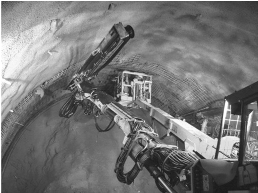
Figure A.6.2.3 Shotcrete and Lattice girder Support 11
