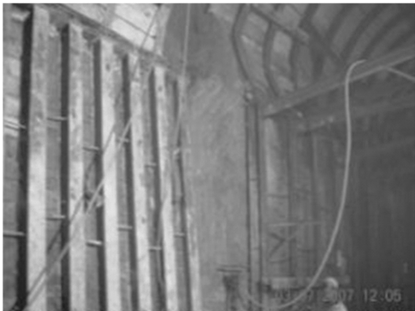
Figure 7.5 Tunnel Support failure due to swelling soil.
