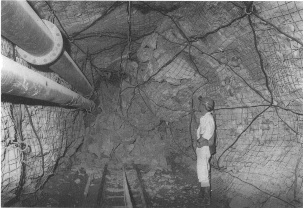
Figure 4. Wire mesh and wire rope lacing behaviour
