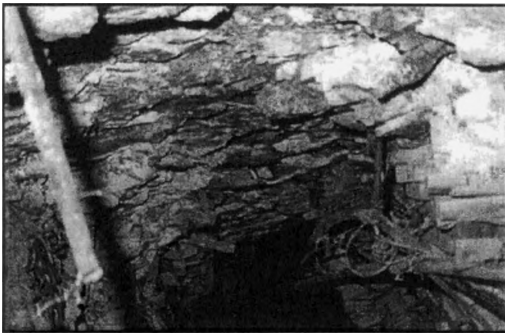
Figure 7 Stability problems in the WDL East Gold Mine strike gully
