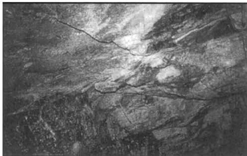
Figure 11 Example of low cohesion environment caused by heavily serpentinised rock.
