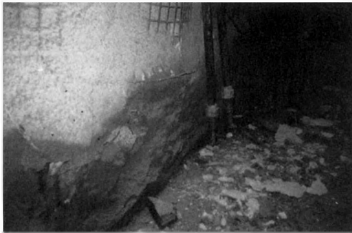
Figures 6 (above) and 7 (below). Ongoing deformation causing localised spalling of plain shotcrete off the mesh.
