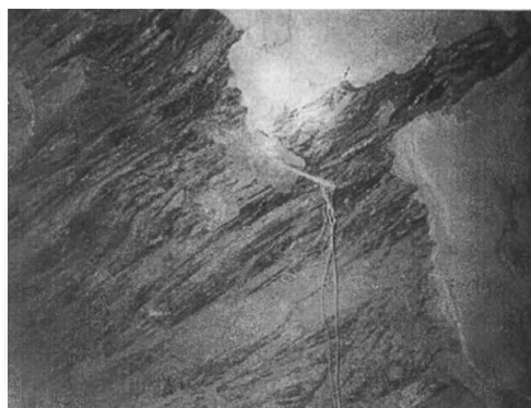
Figure 10. Shotcrete layer fell off from the lower wall after damage by mucking units, showing layer separation.
