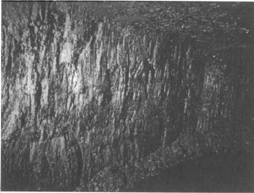
Figure 13 Coal pillar condition soon after cutting.
