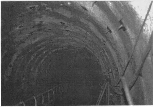
Figure 9. The roadway reinforced by bolt injection.
