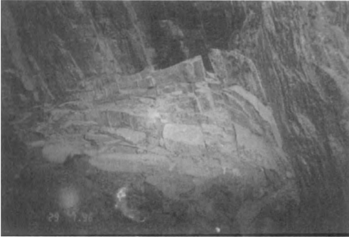
Figure 1: Stress induced fracturing above the backs of an old haulage drive, 320 Level.
