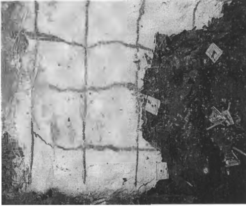
Figure 1. Damage to the leading edge of the Mineguard membrane after a development firing.
