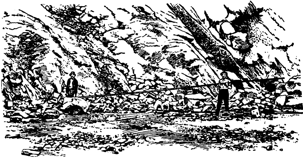
Fig. 159.—Loading the holes in a quarry where snakeholing is practiced.
