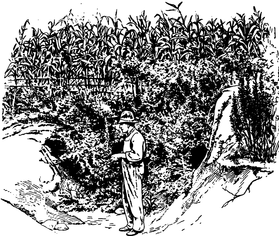
Fig. 134.—Showing a log and brush dam built across a gully to form an anchorage for the moved soil. A woven wire fence with the top set level with the ground is also good.
