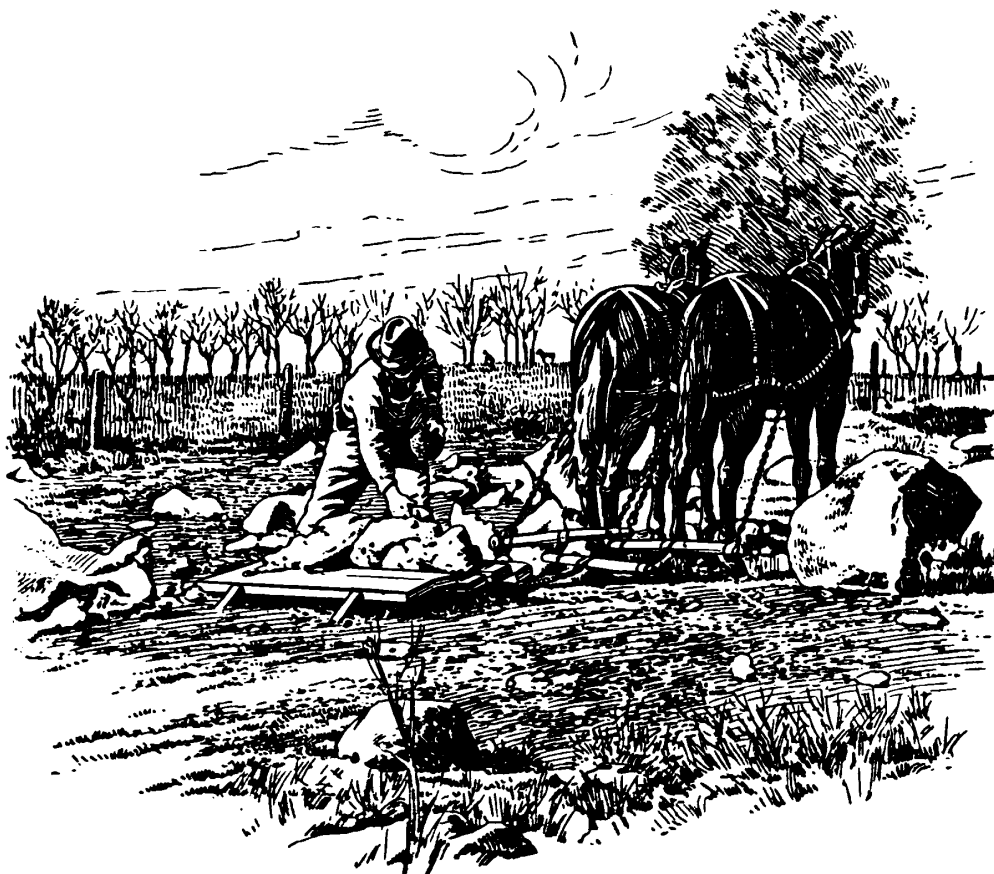
Fig. 118.—Stone boat suitable for hauling boulder fragments for short distances.
