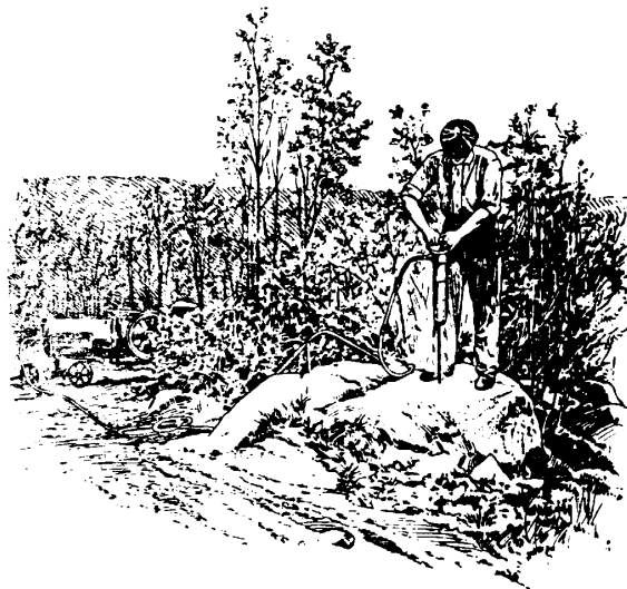
Fig. 77.—Portable compressor supplying air to hammer drill.
