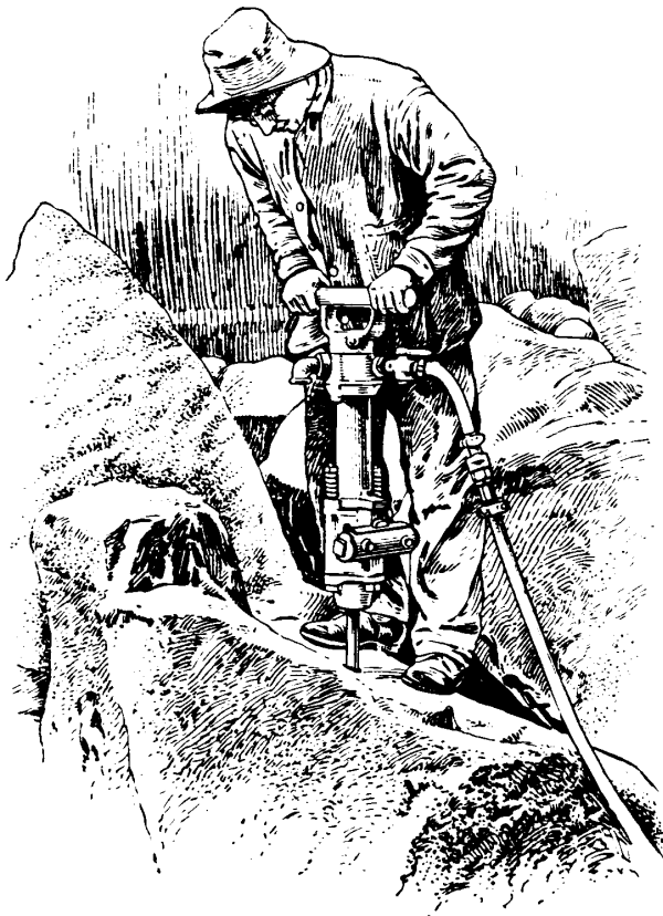
Fig. 72.—Hammer drill on road work.
