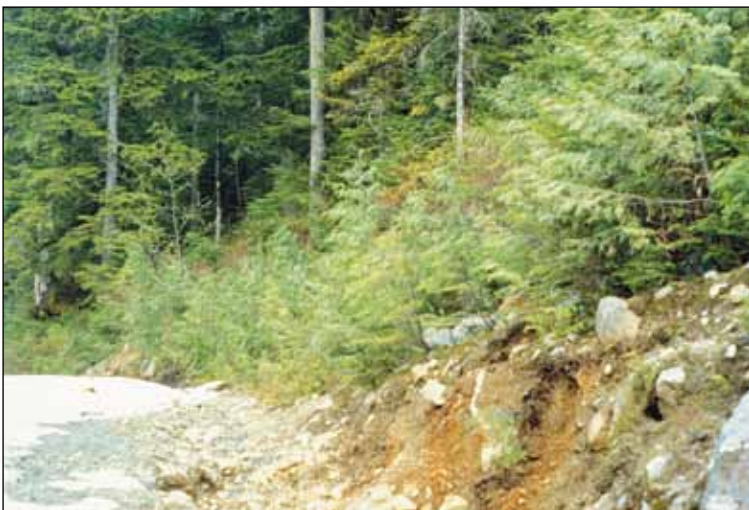
FIGURE 66 Dense natural regeneration of redcedar on the exposed mineral soil of a roadcut.
