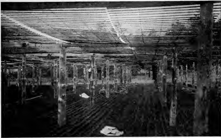
FIG. 70. — High cover formed of posts and scantlings covered with mats woven from narrow slats and wire.
