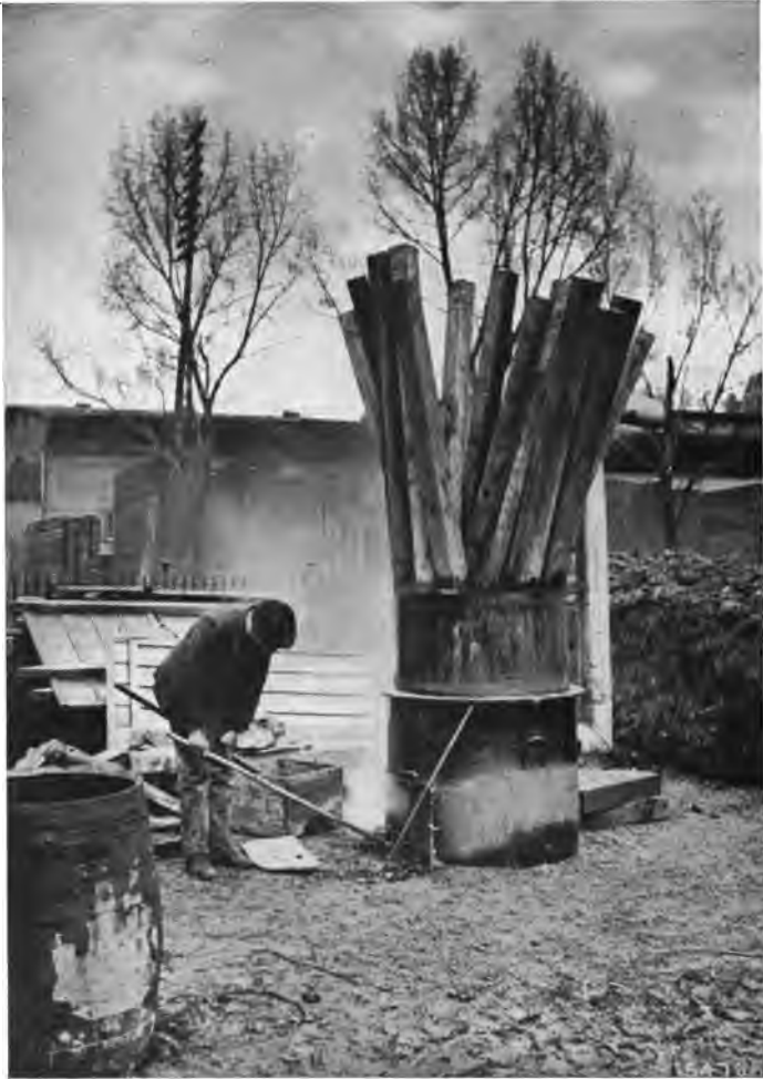
FIG. 44. — A POST TREATING PLANT, MONTGOMERY CO., MARYLAND.
