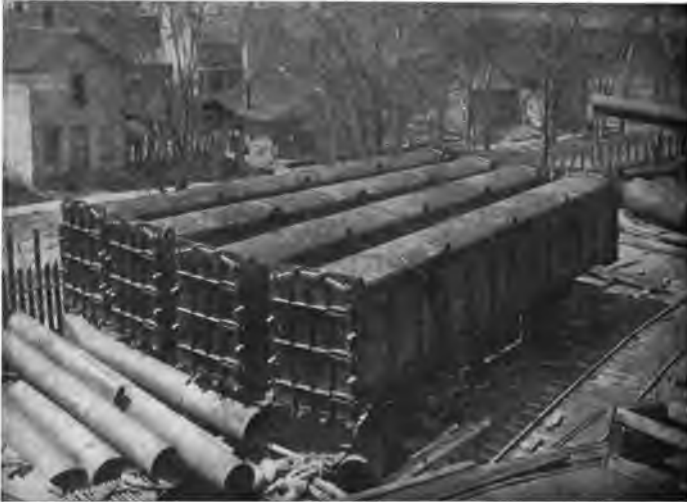
FIG. 39. — RETORTS USED IN THE WOOD DISTILLATION INDUSTRY.
