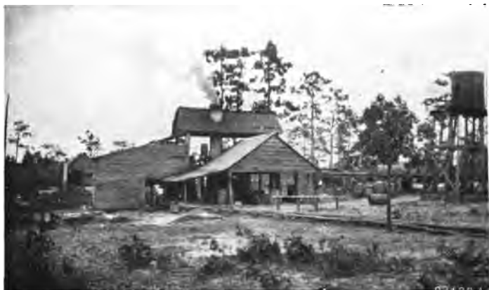
FIG. 38. — A TURPENTINE STILL ON THE FLORIDA NATIONAL FOREST.
