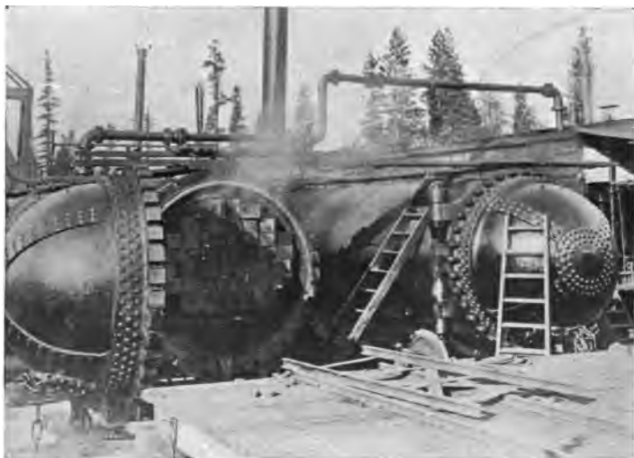
FIG. 43. — HIGH-PRESSURE CYLINDERS USED IN TREATING TIES, OAKLAND, CALIFORNIA.
