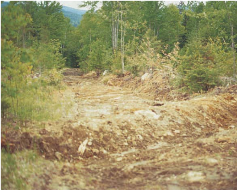
Water bars move water out of the trail onto the forest floor.
