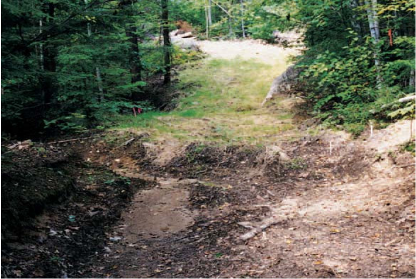
A trail closed-out with water bar and seeding.
