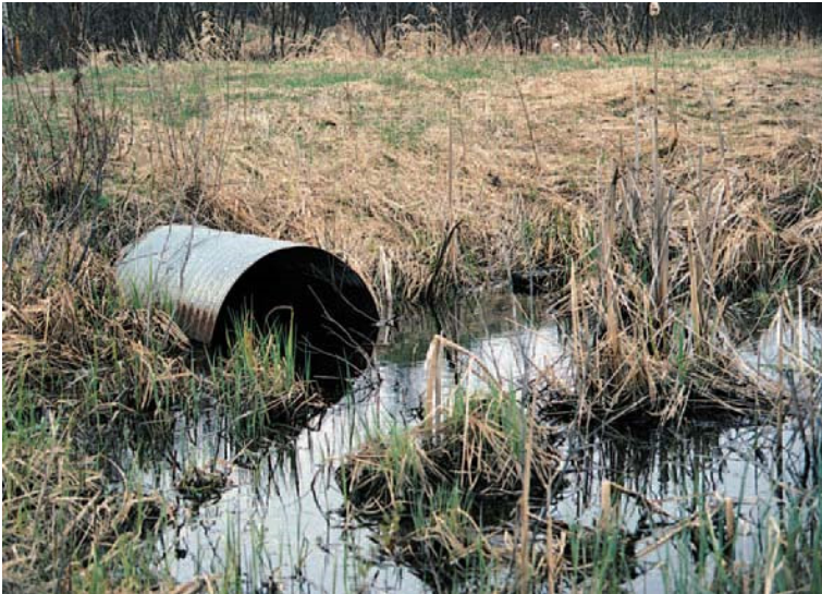
Wetland culverts allow for cross drainage if the road fill does not.
