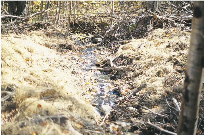
Closeout of a temporary stream crossing.
