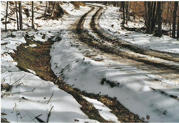
Properly sized ditches capture and slow down runoff.
