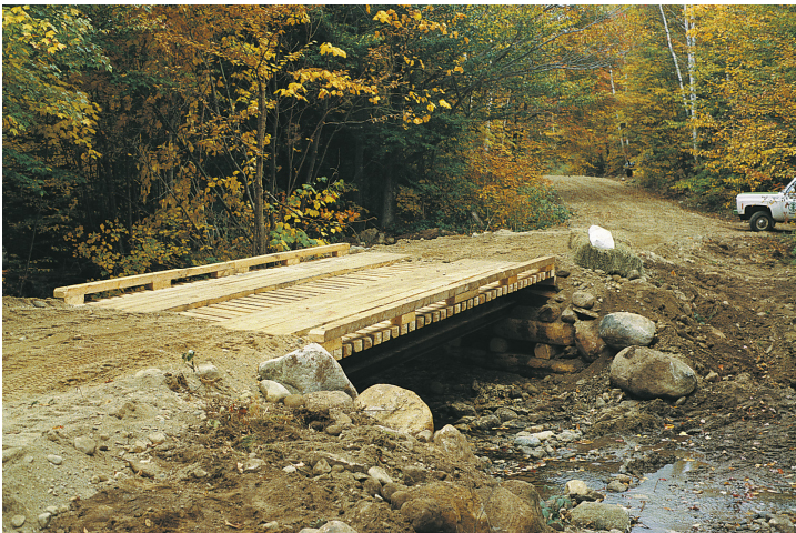
A permanent bridge.
