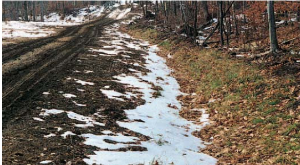
Revegetated road ditches carry water without eroding.
