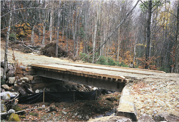
A permanent bridge on a truck road.
