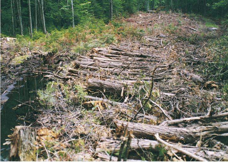
Log corduroy used for a skid trail across a wet area.
