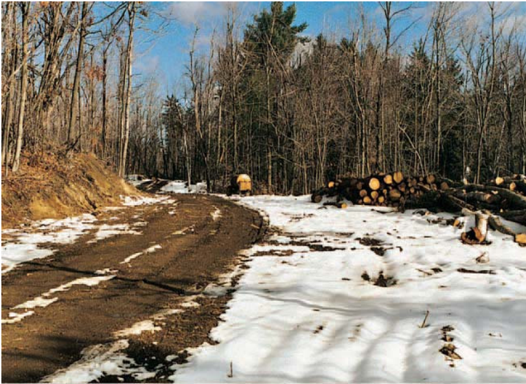
A well-maintained, well-drained landing.
