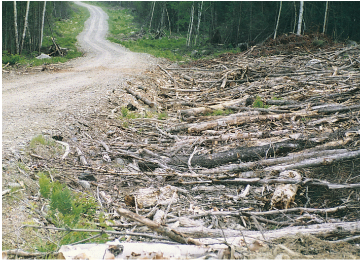
Slash and logging debris can help stabilize exposed soil on log landings.
