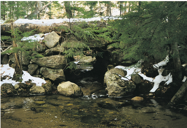
An old stone culvert still functioning.
