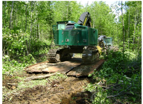
A temporary bridge.
