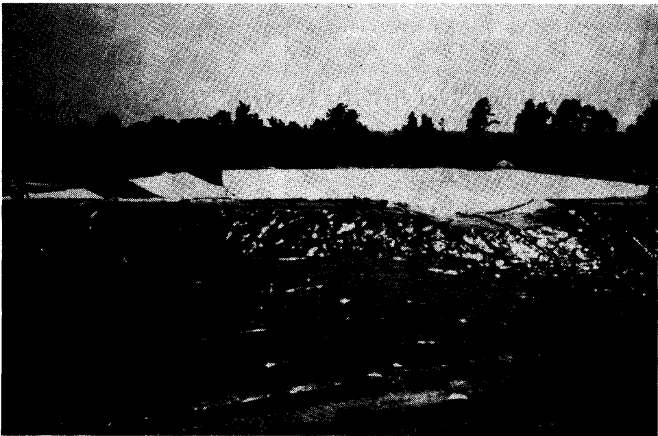
FIGURE 9.21 Application of geotextile for protection.
