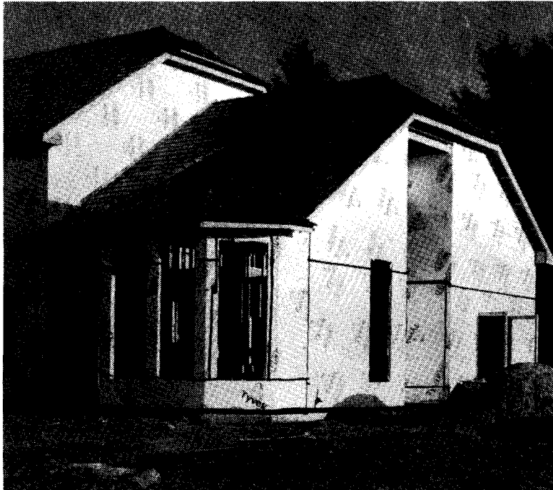
FIGURE 6.31 Tyvek® spunbond material for house insulation (courtesy of DuPont).
