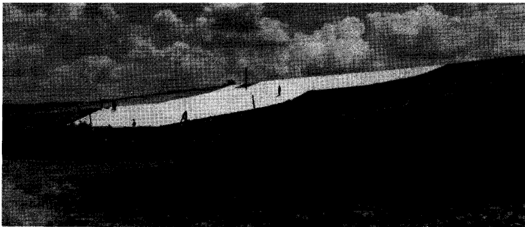
FIGURE 9.17 Geotextile used to stabilize a steep highway embankment (courtesy of Polyfelt).
