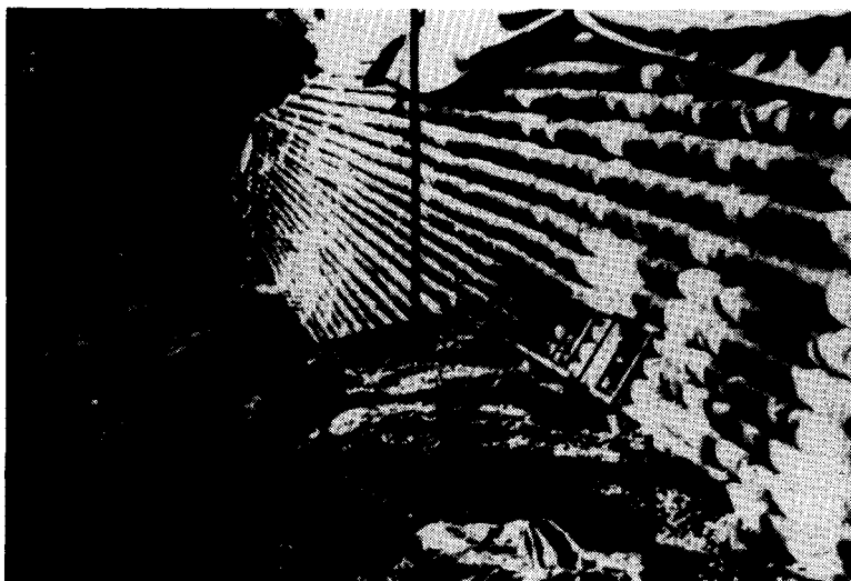
FIGURE 9.24 Geotextile reinforced wall (courtesy of Hoechst Celanese).
