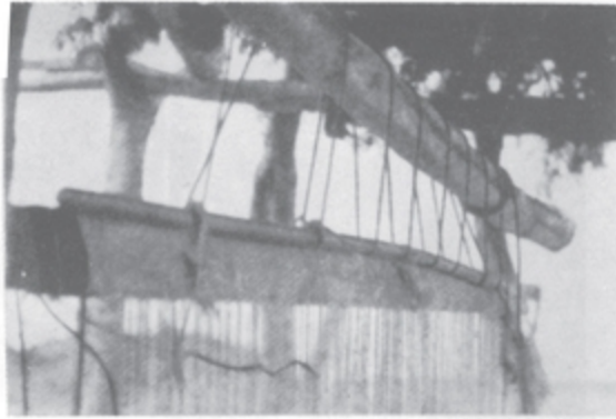
[a] Warp-beam with extra warp rolled under
