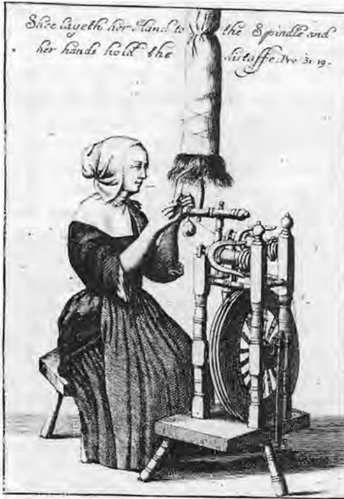
59 The two-handed spinning wheel illustrated by Thomas Firmin in 1681
