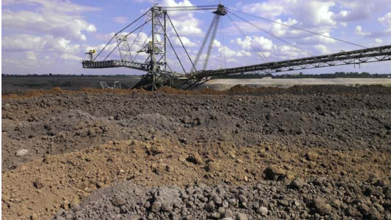
Picture 11.1 Backfilling of an open-pit mine.
