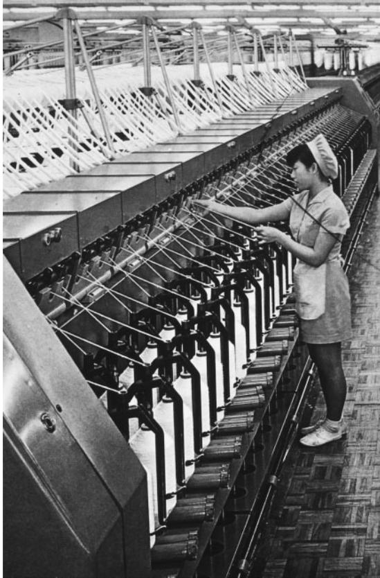
**FIGURE 5.24** Basic roving frame.
