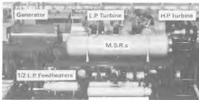
**Fig.12 Location of L.P. Feedheaters Sizewell N.P.S.**
