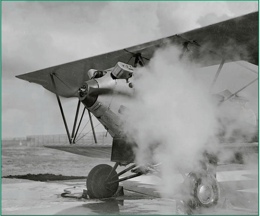
**George and William Besler developed the first working steam engine airplane in the early 1830s. In this photograph of the Beslers' plane, George Besler is nearly obscured in the pilot's seat by the steam issuing from the engine.**
