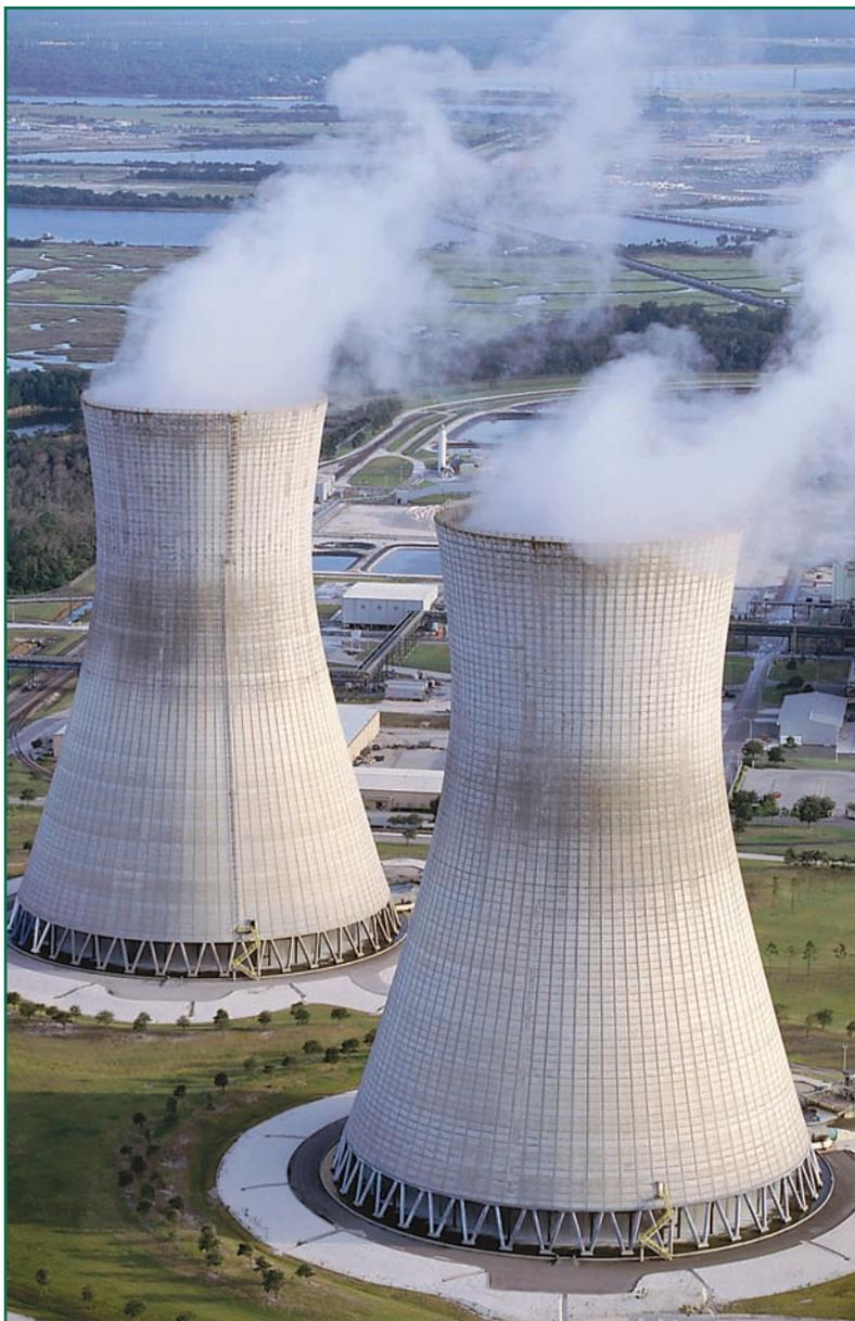
**It is steam, not smoke, that drifts from the cooling towers of nuclear power plants. The energy produced by nuclear fission makes the steam that drives the turbines to generate electricity.**
