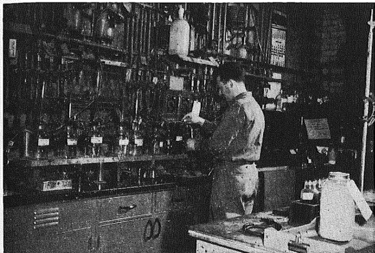
FIG. 2-3. Water-treating room at a large power plant features complete laboratory receiving sample lines from various parts of the plant. (Courtesy of Consolidated Edison Company of New York.)
