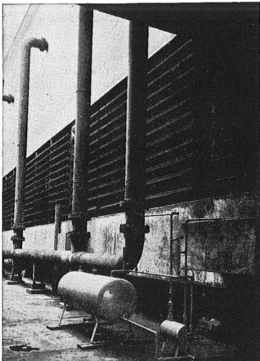
**FIG. 11-3.** Proportioning hydraulic feeder treating cooling tower recirculating water. (Courtesy of Water Service Laboratories.)
