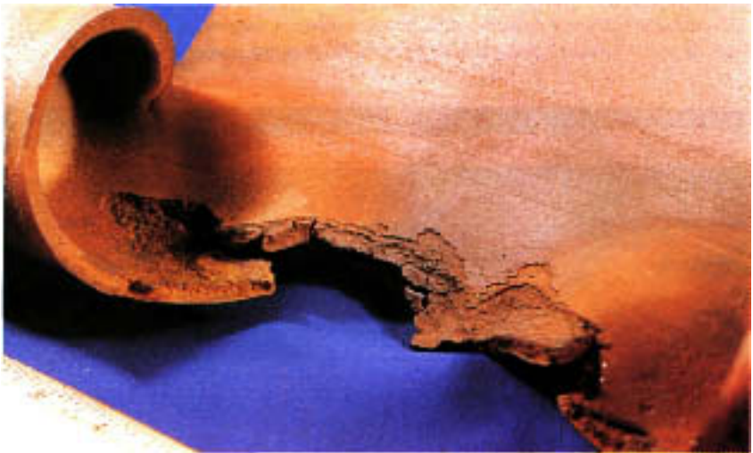
Figure 6.4 Metal loss at the origin of rupture.
