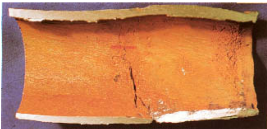
Figure 7.6 Transverse fissures near rolled end.
