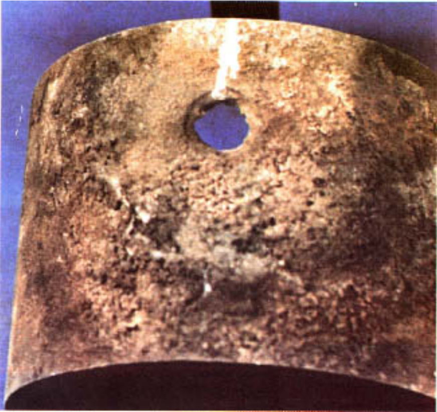
Figure 6.9 Perforation resulting from corrosion of internal surface.
