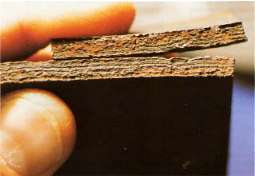
Figure 19.5 Edges of brittle rupture.
