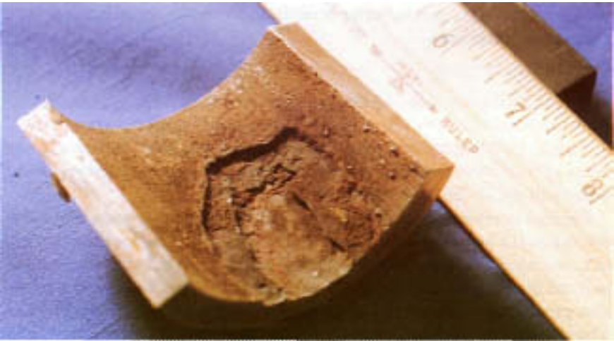
Figure 4.6 Region of caustic gouging along internal surface.
