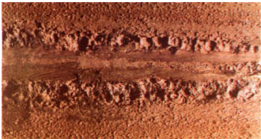
Figure 6.6 Appearance of deposits covering groove.
