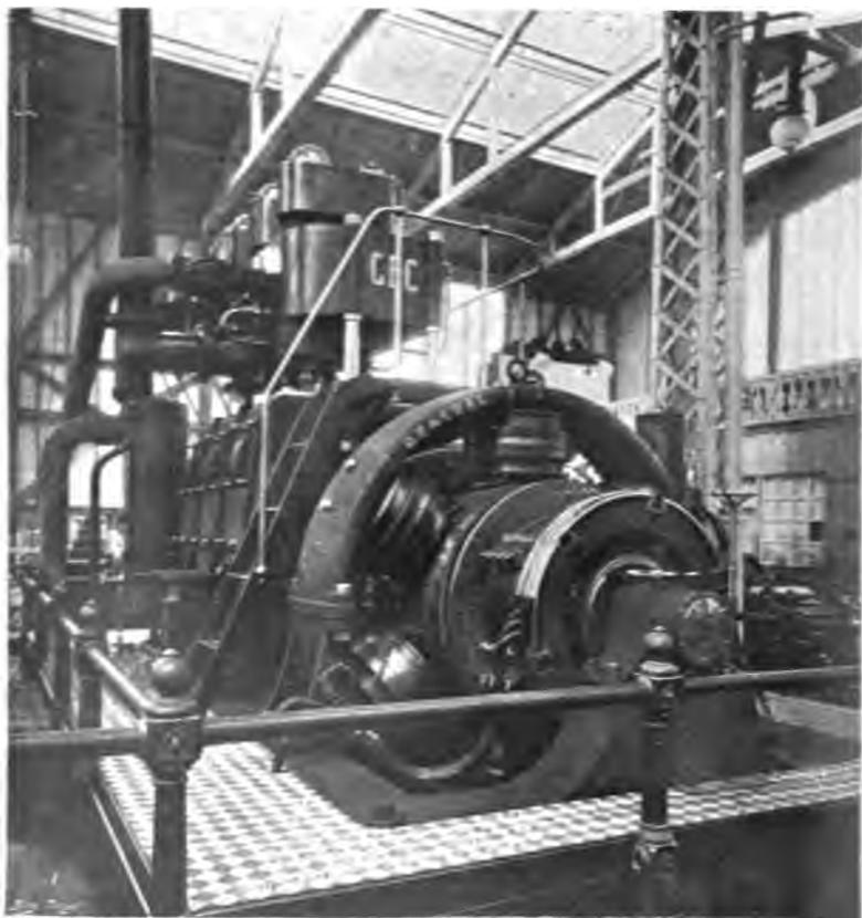
FIG. 139.—360 I.H.P. "TEACHE" ENGINE, BY MESSRS. DAVEY, PAAMAN & CO., COLCHESTER, DRIVING DYNAMO BY THE GENERAL ELECTRIC CO.
