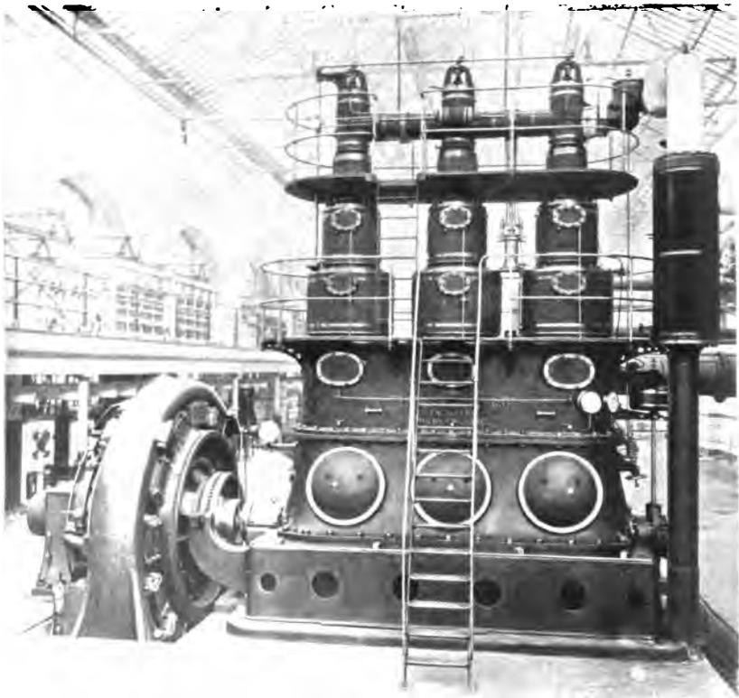
FIG. 136.—1,075 H.P. "WILLANS" HIGH SPEED ENGINE DIRECT CONNECTED TO DYNAMO.
