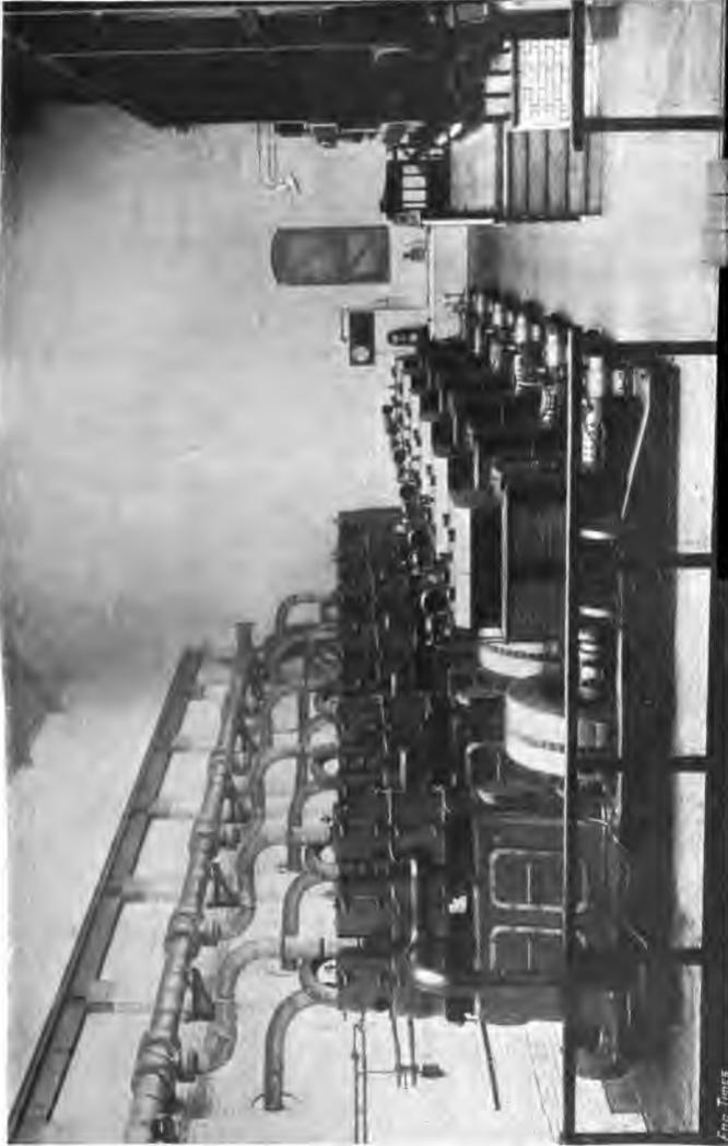
FIG. 9.—VIEW SHOWING SIX SETS OF THREE-CRANK TANDEM COMPOUND "BELLISS" ENGINES AND DYNAMOS INSTALLED AT THE WATERLOO AND CITY ELECTRIC RAILWAY GENERATING STATION.
