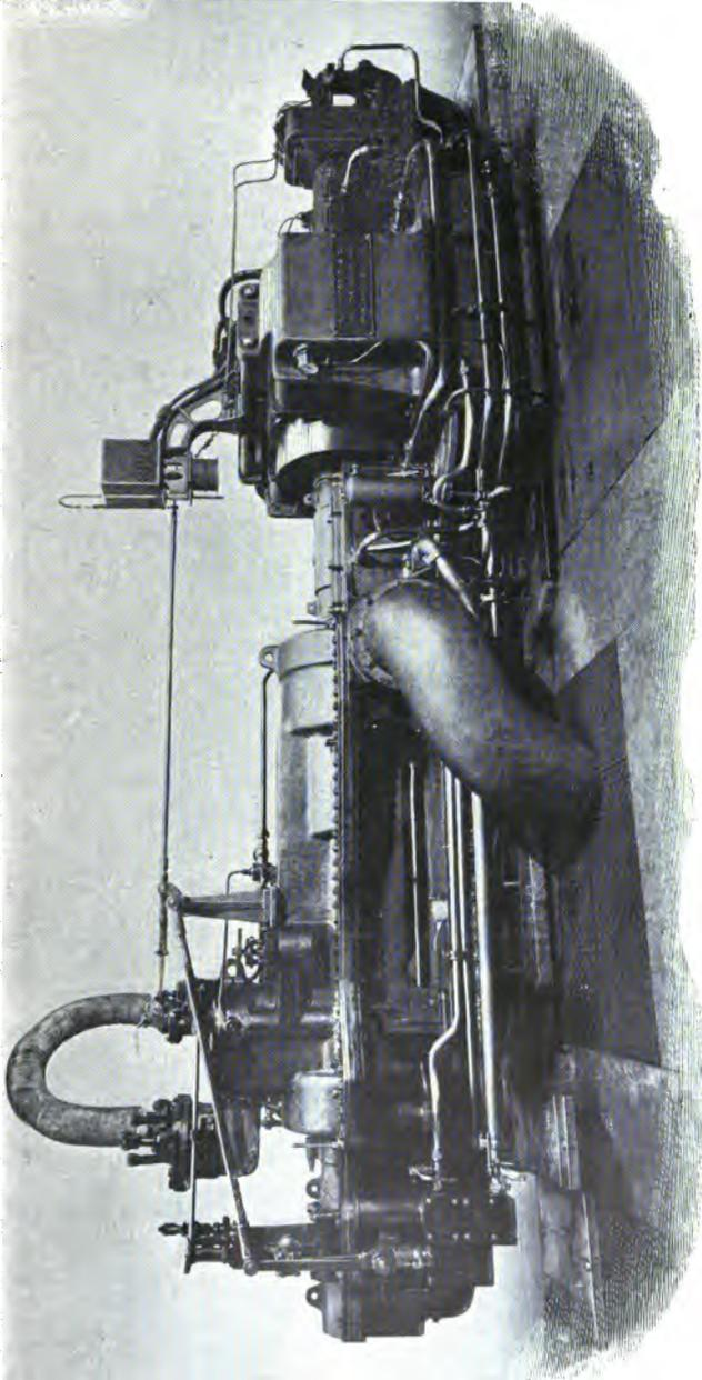
FIG. 130.—PARSONS' STEAM TURBINE DRIVING A 500 K.W. ALTERNATOR.
