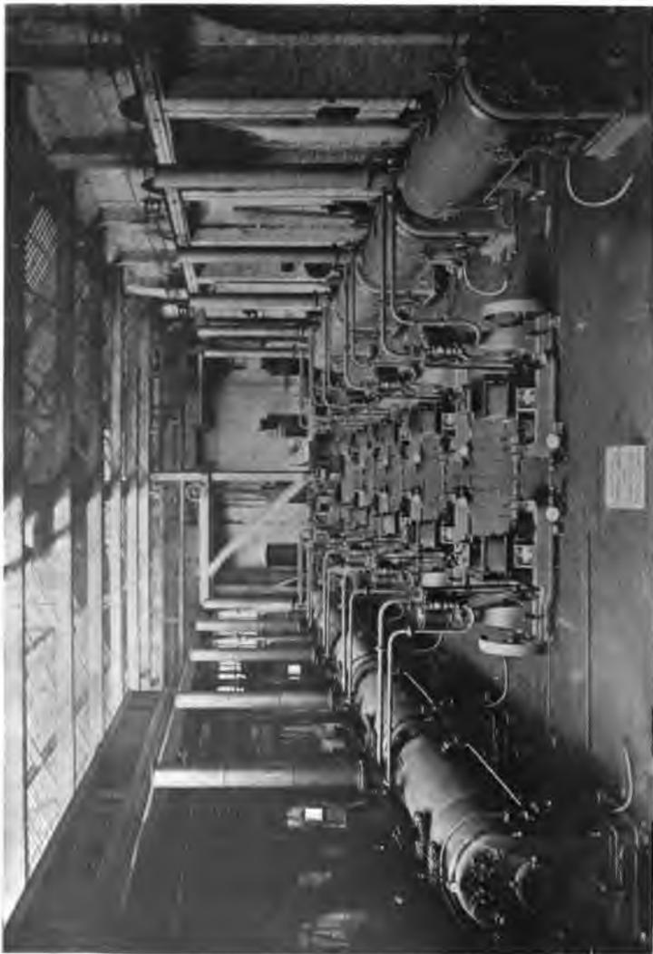
FIG. 27.—GROUP OF TEN "ROBEY" ENGINES. "TYNE" DYNAMOS AND LOCOMOTIVE BOILERS, SUPPLIED TO THE WAR OFFICE.
