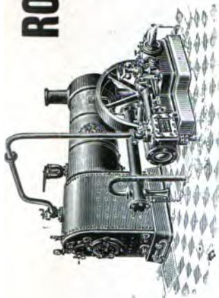
MEDIUM STROKE HORIZONTAL ENGINES, WITH SEPARATE LOCOMOTIVE BOILER.
