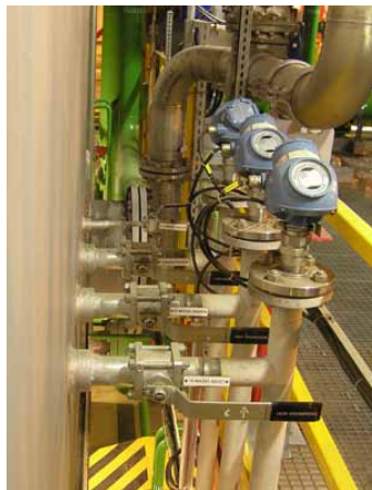
Figure 1. Three Rosemount 5301 Guided Wave Radars used for condenser level control.
