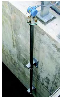
Guided Wave Radar Installed
