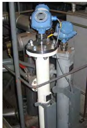
Figure 2. A second Rosemount 5301 replaces the electronic displacer.
