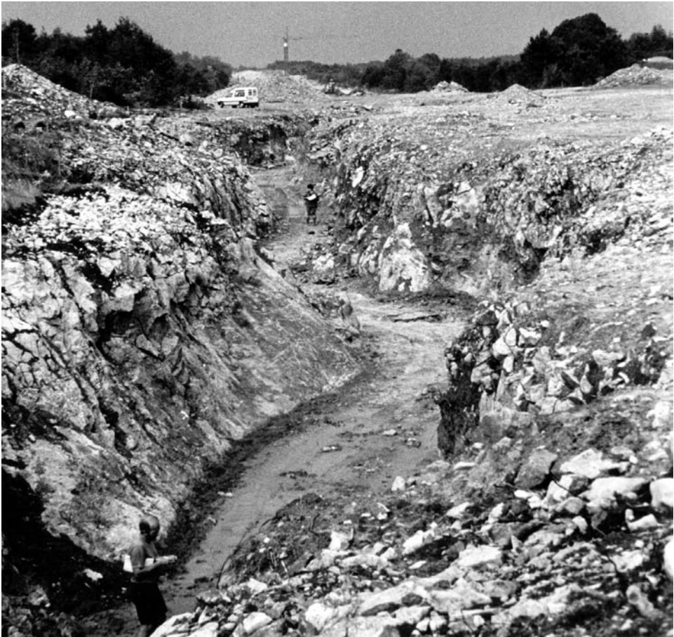
Figure 13.3.2. Large unroofed cave passage that lay parallel to the karst surface, near Divača, seen after its sediment has been removed in preparation for road construction.
