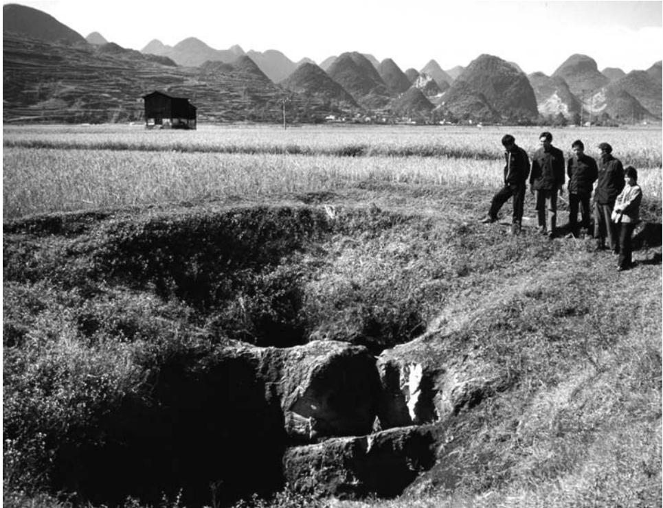
Figure 8.9. A subsidence sinkhole induced by water table decline as groundwater was pumped through the well house visible beyond, in the Shuicheng karst basin, China. The crest of a limestone pinnacle is exposed in the sinkhole only a metre below the original ground level. TW.
