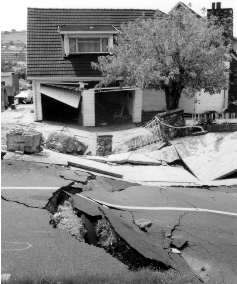
Figure 10.8. A house and road destroyed by sinkhole development in Centurion, South Africa, during a period of water table decline within the underlying dolomite aquifer; major costs will have to be borne, wholly or partly, by the home owner, his insurance company, the highways authority and perhaps by whoever was responsible for the groundwater abstraction. Photo: Fred Bell.
