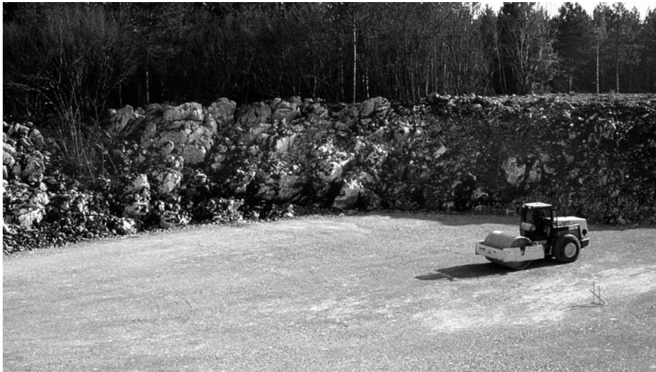
Figure 13.3.3. Compacting a graded fill placed inside a large sinkhole that had previously been filled with loose soil, near Divača.
