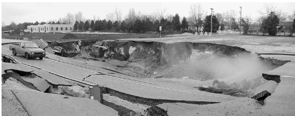
Figure 1.5. A major sinkhole collapse under an urban highway in Bowling Green, a city that stands entirely on the Sinkhole Plain of Kentucky; the fog is due to warm air rising from the breached cave early on a cold winter morning.
