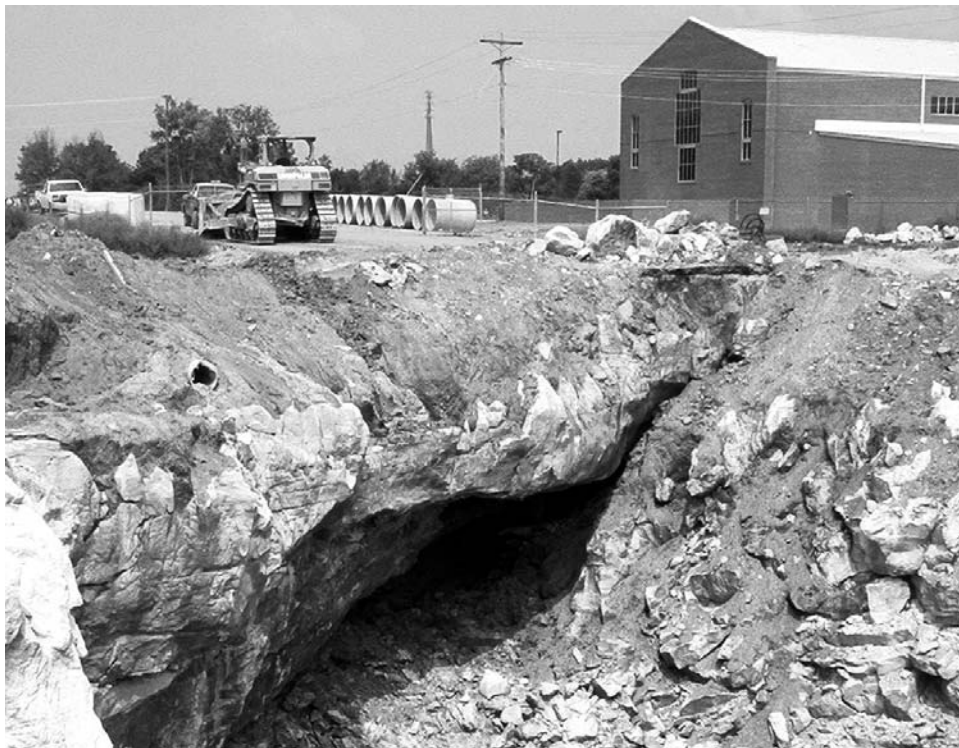
Figure 7.1. Fractured rock around the margin of the new collapse sinkhole that destroyed Dishman Lane in Bowling Green, Kentucky, in 2002.
