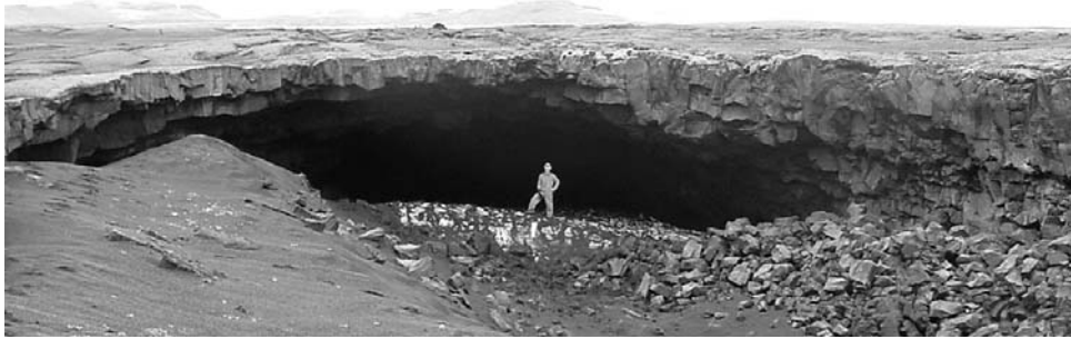
Figure 6.4. The entrance to the Flothellir lava tube in Iceland where a very thin roof has collapsed across a very wide span.
