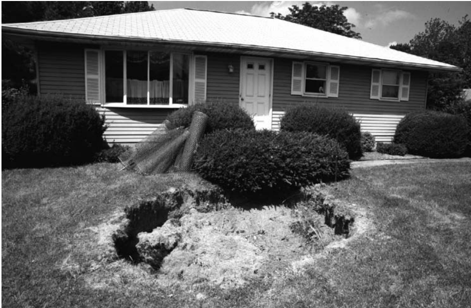
Figure 4.8. A dropout sinkhole in the front lawn of a house in Pennsylvania; the hole was originally 5 m deep but was filled with soil to prevent the sides flaring out, and the soil fill had compacted and settled by 0.7 m by the time this photo was taken. TW.
