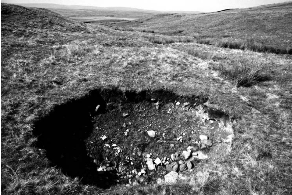
Figure 4.1. A typical small, fresh subsidence sinkhole formed in till overlying cavernous limestone in the Yorkshire Dales, U.K.; the new sinkhole is only about 3 m wide and 1 m deep, and it does not expose the limestone as rockhead is at a depth of about 3 m. TW.
