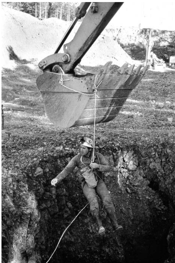
Figure 9.7. Direct exploration: an engineering geologist, who is also an experienced caver, abseils from an excavator bucket into a sinkhole that collapsed into an open cave during road construction in Slovenia.
