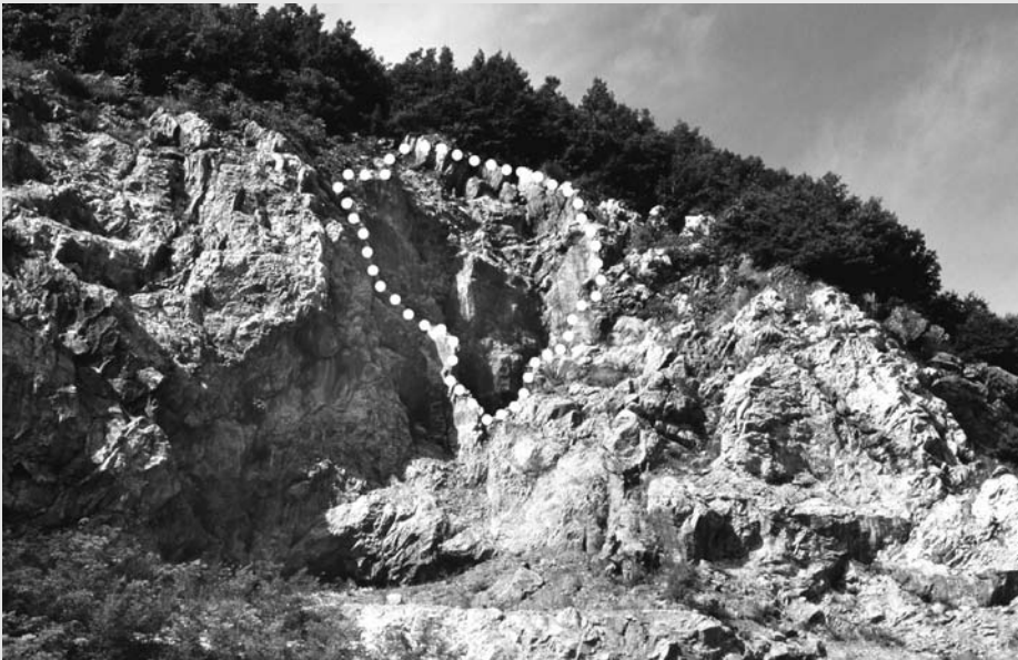
Figure 5.1.2. The upper bench of the Chunglim quarry, with the subsoil outcrop of the now-empty buried sinkhole picked out by the dotted line. Entrances to the mine workings are almost hidden behind the debris barriers piled up on the main bench at the foot of the picture.
