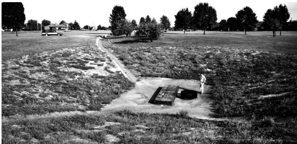
Figure 12.1. A shallow sinkhole in Bowling Green, Kentucky, engineered to take storm-water drainage from an urban area directly into an underlying limestone cave without eroding the soil cover.
