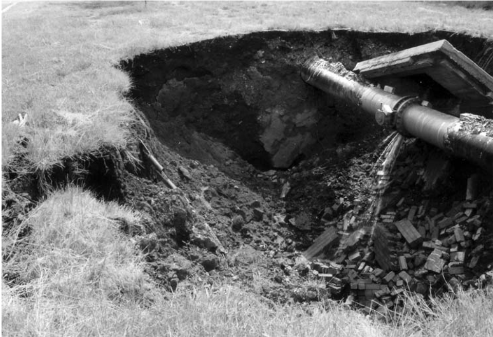
Figure 1.12. A small suffosion sinkhole that has opened up beneath a leaking pipeline in the soil-covered dolomite karst south of Pretoria, South Africa.
