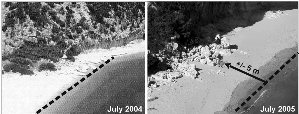
Fig. 9. Two photographs of Cala Luna taken in July before and after the extreme December flood, showing the increase in beach sediment in the northern section, confirmed by periodical monitoring measurements of the beach.
