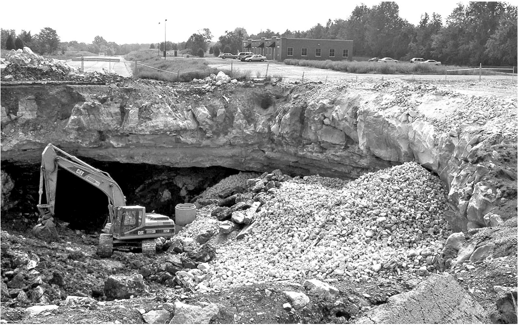
Fig. 3. The edge of the collapse doline that destroyed a road in Kentucky in 2002, viewed when remediation was under way; the broken edge shows the wide cave chamber spanned by a very thin roof, of which the upper half was a zone of soil-filled fissures between rockhead pinnacles.
