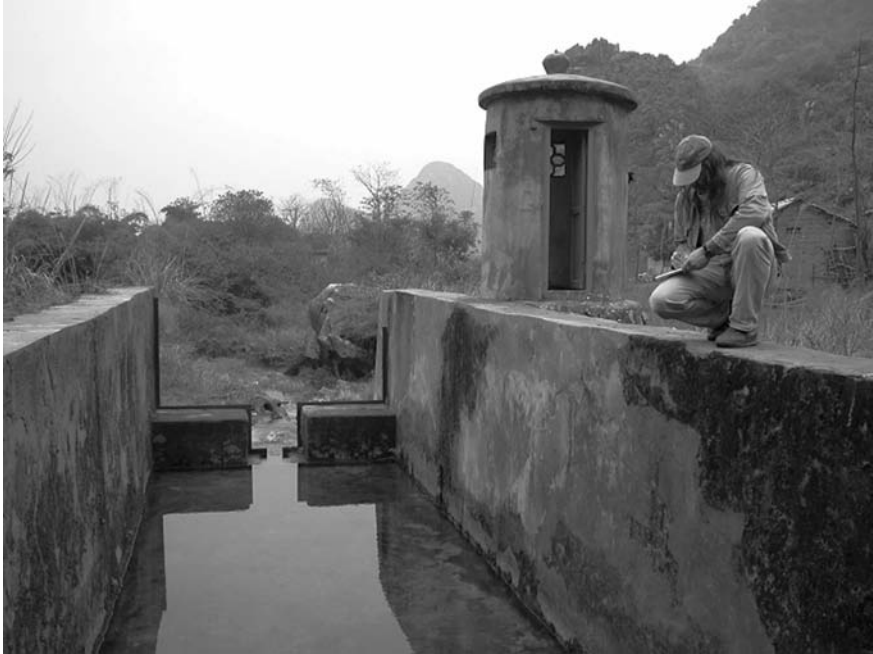
Figure 4.4. Weir for discharge measurement at Spring 31 of the Guilin Karst Experimental Site, near Yaji Village, Guangxi Autonomous Region, China. A pressure transducer makes continuous depth measurements upstream from the weir that are related to discharge using the appropriate relationships for the weir’s three sections. Use of a compound weir is useful in this case to capture a wide range of flows that results from the monsoon climate of southwest China. This photo was taken in February, typically late in the dry season prior to the onset of the Asian Summer Monsoon (photo Groves).
