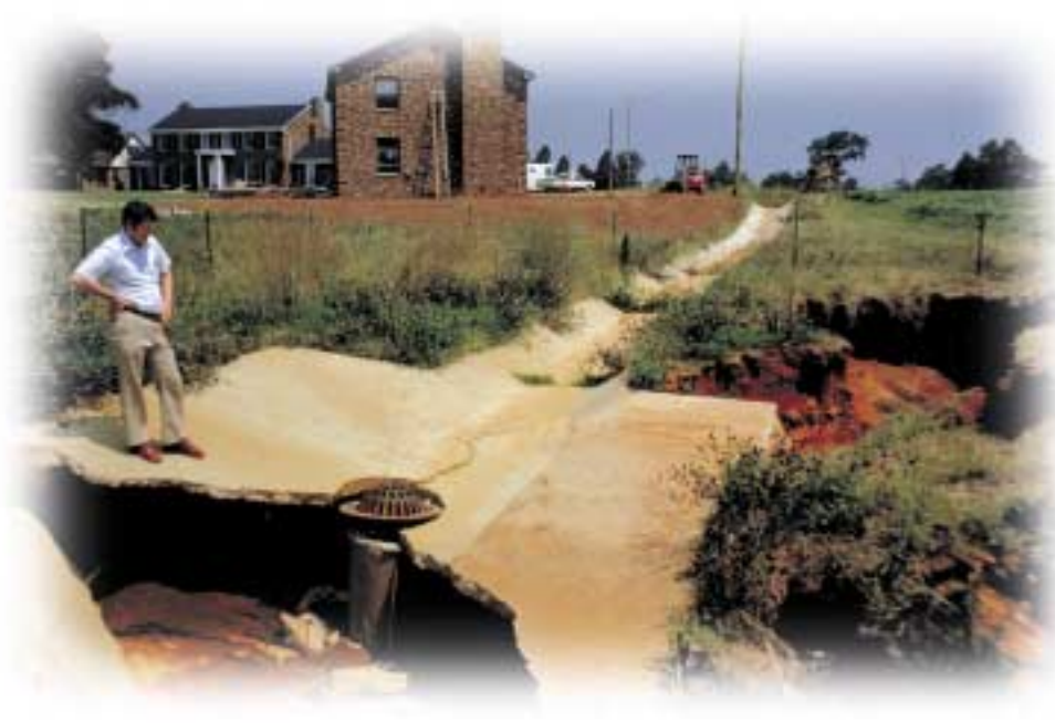
Fig. 30. Sinkhole collapse commonly results where the casings of drainage wells are not properly sealed to the bedrock.
