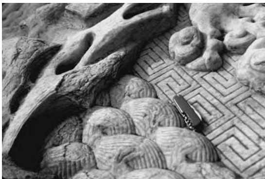
Figure 12.14 (Upper) Façade of a Mayan temple at Chichen Itza, Mexico. It is built of soft Tertiary limestone facings with trash stone filling behind, a common method worldwide. Note that weathering discolouration is distinctly less beneath projecting lintels that offer some protection from rain. The building was buried in second growth forest for ~800 year. (Lower) Detail of sulphation breaking up ornamental carving of the Ming dynasty on an outside staircase in the Winter Palace, Beijing, China.
