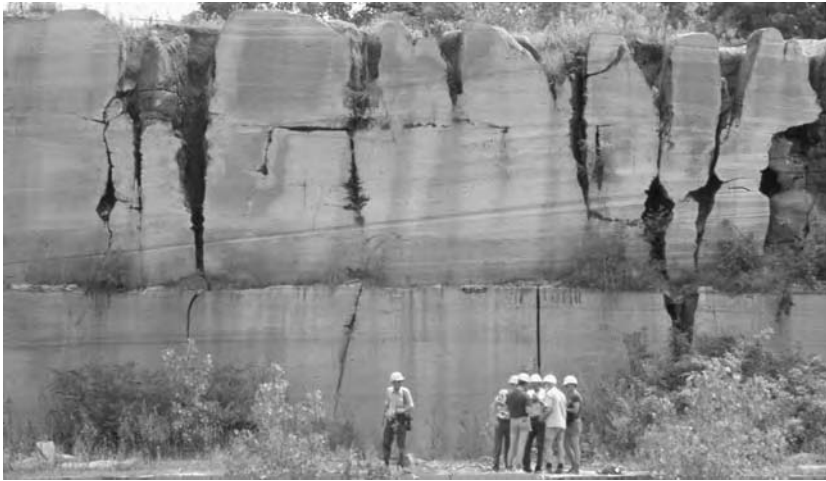
Figure 5.25 ‘Pinnacle and cutter’ relief exposed in a limestone quarry face in Kentucky. This illustrates the tapering closure of solutionally enlarged joints with depth in the epikarst.
