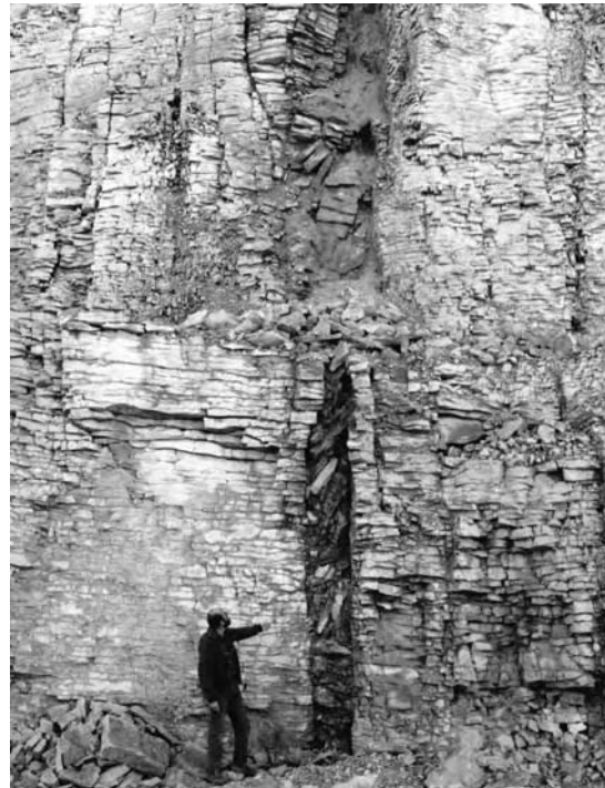
Figure 5.27 Very high fissure frequency exposed in a quarry face near Te Kuiti, New Zealand. The vertical feature to the right of the figure is a minor fault and is the kind of discontinuity that permits doline initiation by providing a preferred drainage path for infiltrating rainwater. Reproduced from Williams, P.W., Polygonal karst and palaeokarst of the King Country, North Island, New Zealand. Zeitschrift für Geomorphologie , Suppl. Vol 136, 45–67, Zeitschrift für Geomorphologie © 2004.
