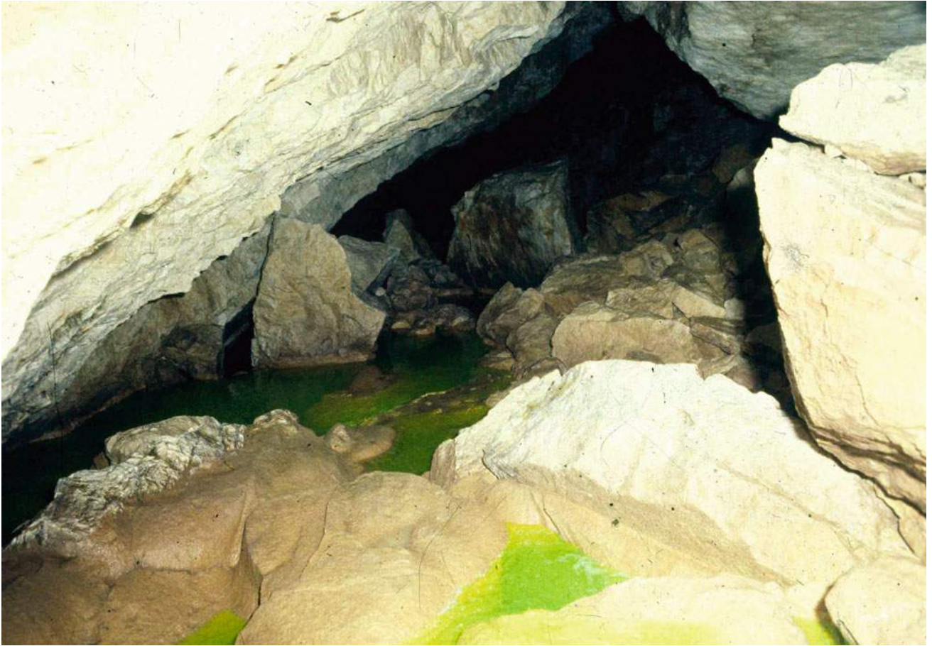
Fig. 6.6 Colour trace in the lower parts of the cavern in Učka Tunnel
