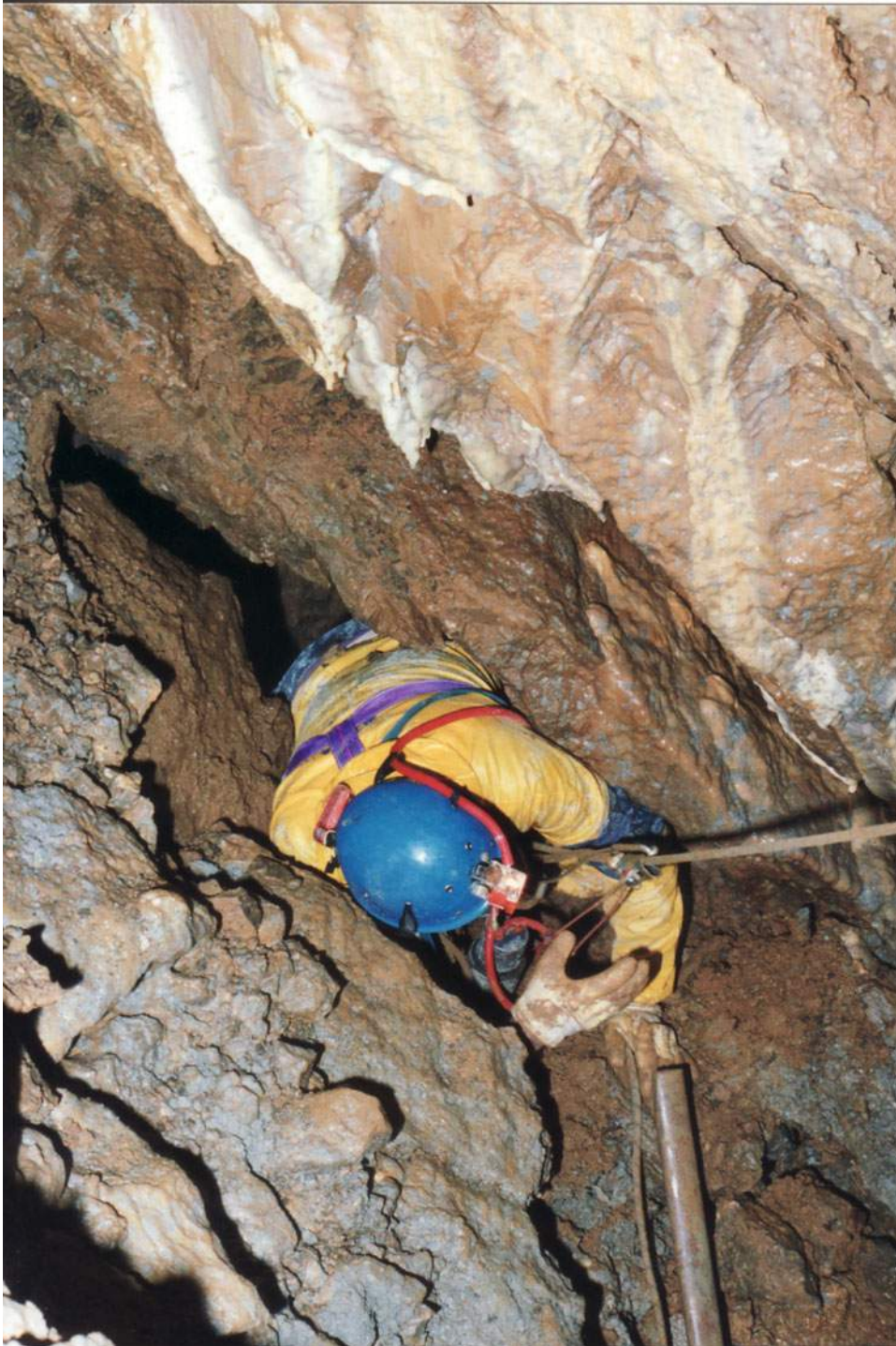
Fig. 6.40 Cavern at km 35 + 541 in Sleme Tunnel
