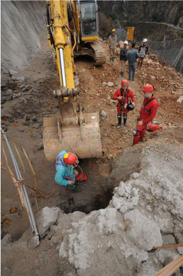
Fig. 8.44 Cavern at km 0 + 393 under pillar on U-2, Katarina viaduct
