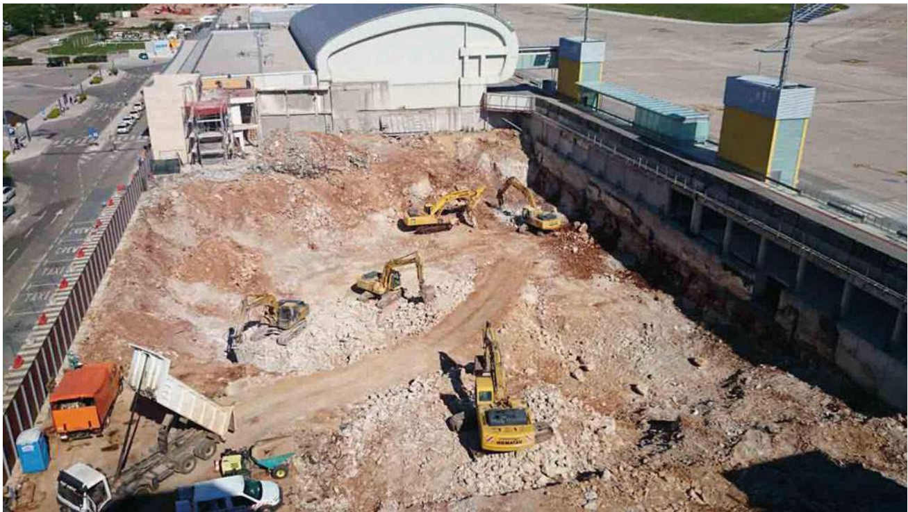
Fig. 9.1 Building “C” at Dubrovnik Airport
