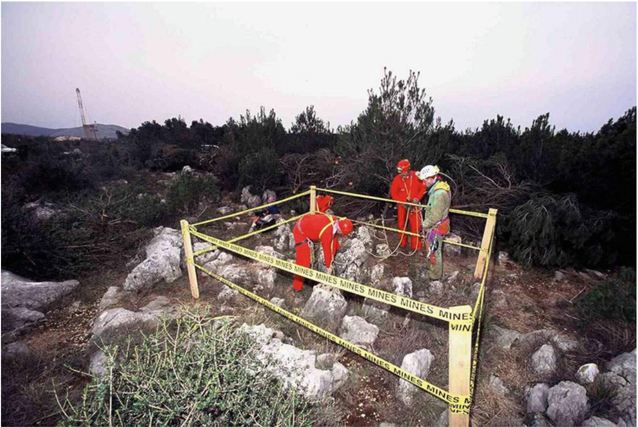
Fig. 8.14 Cave in the embankment at km 71 + 754—Martina Jama near Krka Bridge
