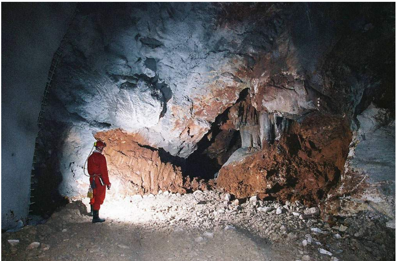
Fig. 7.66 Cavern at km 1 + 965 in Puljani Tunnel (view from tunnel to cavern)
