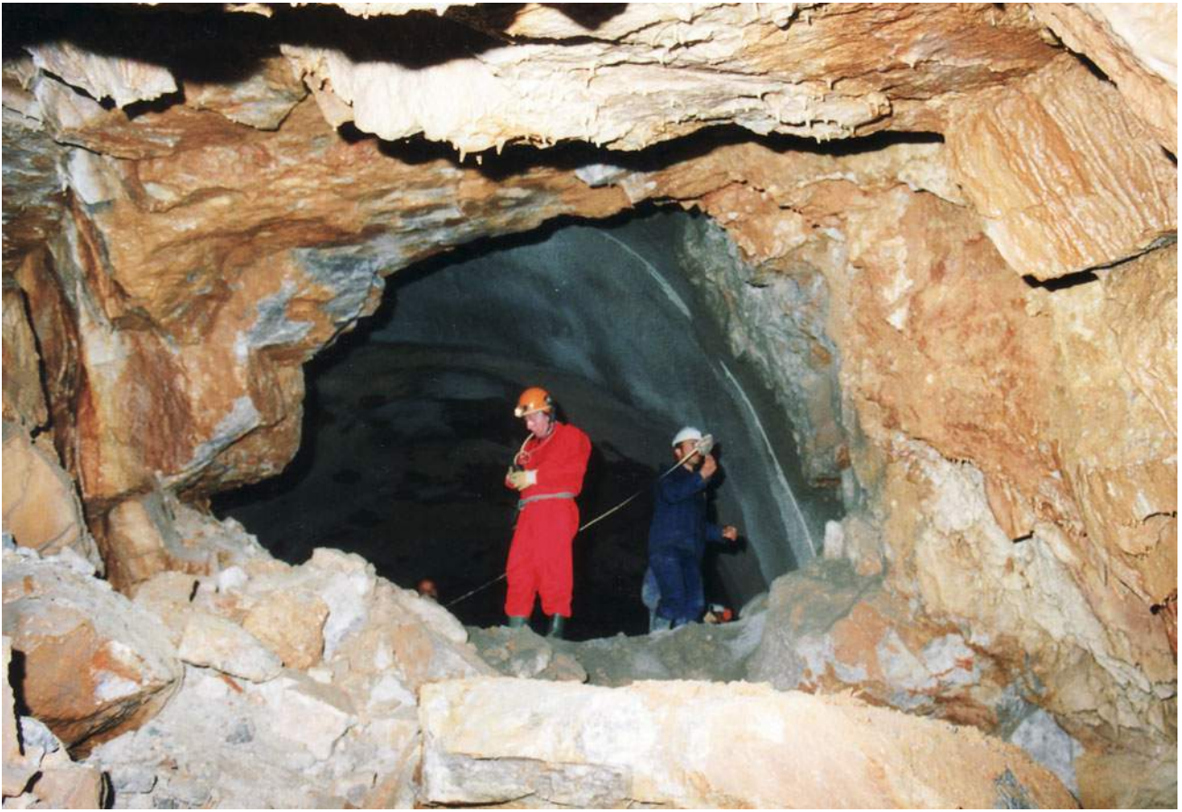
Fig. 6.60 Entrance of cavern at km 47 + 365 in Vršek Tunnel
