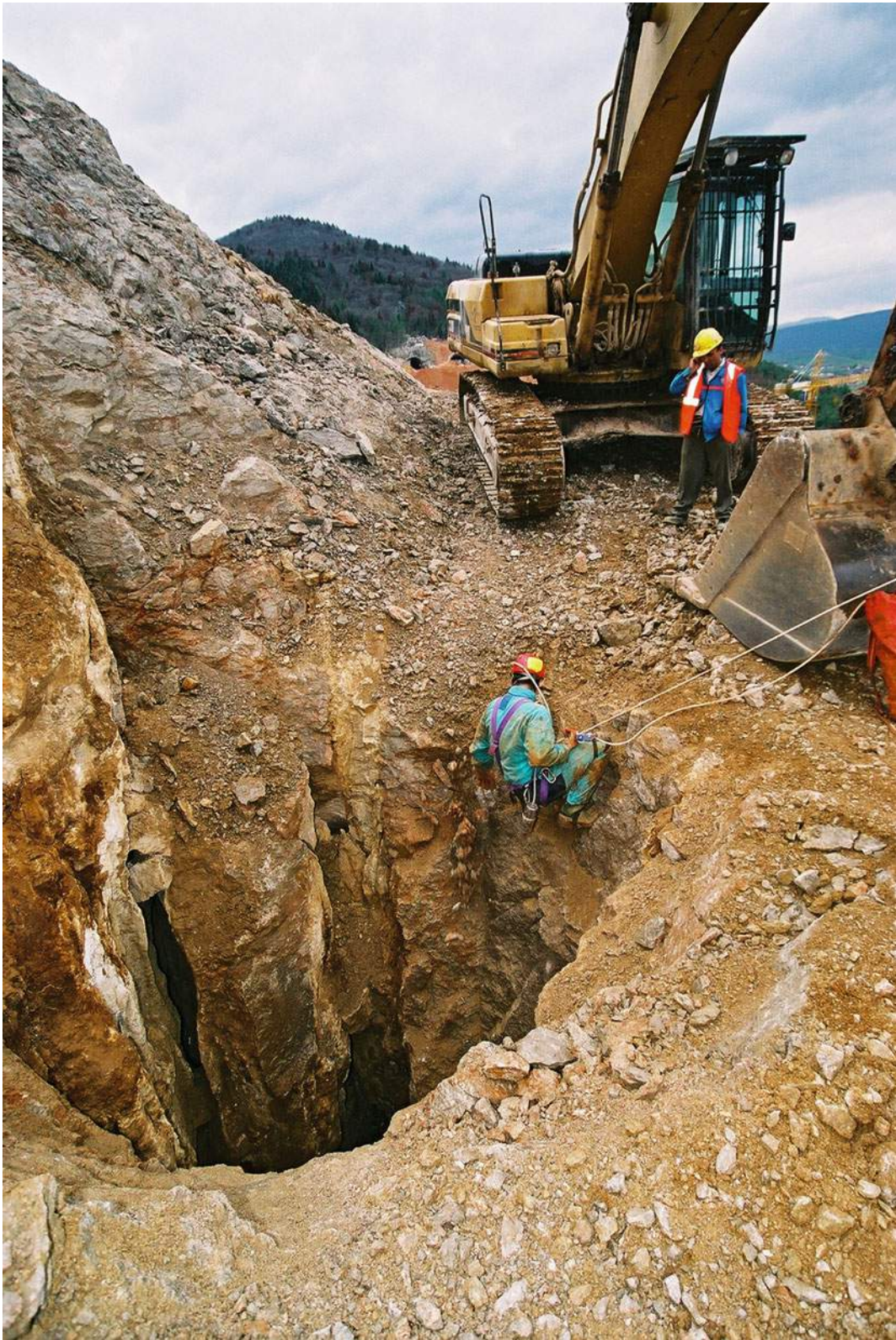
Fig. 8.12 Cavern at km 18 + 130 in Žuta Lokva junction
