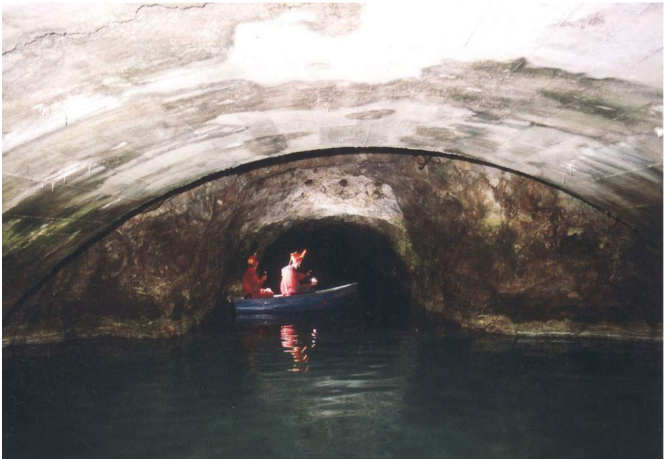
Fig. 5.27 Water-filled drainage tunnel during the inactive period of HPP Dubrovnik
