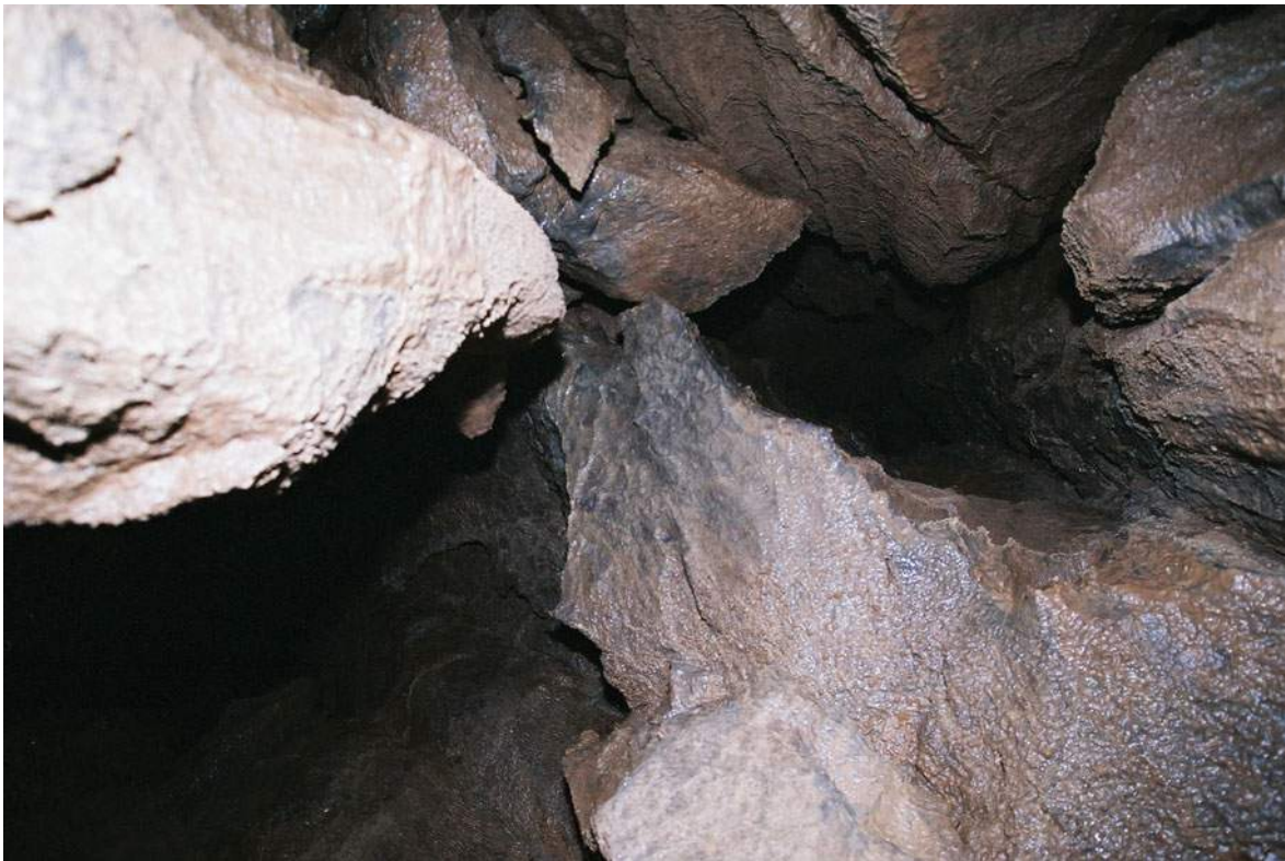
Fig. 6.31 Strong and intensive corrosion in Tuhobić Tunnel
