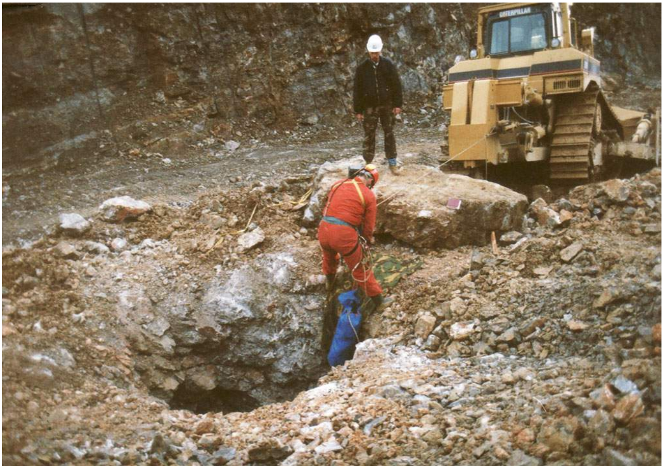
Fig. 8.28 Entrance to cavern at km 17 + 004 on Bosiljevo—Josipdol section
