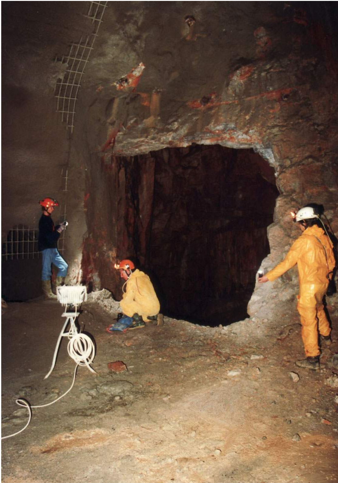
Fig. 6.55 Entrance of cavern at km 47 + 407 in Vršek Tunnel
