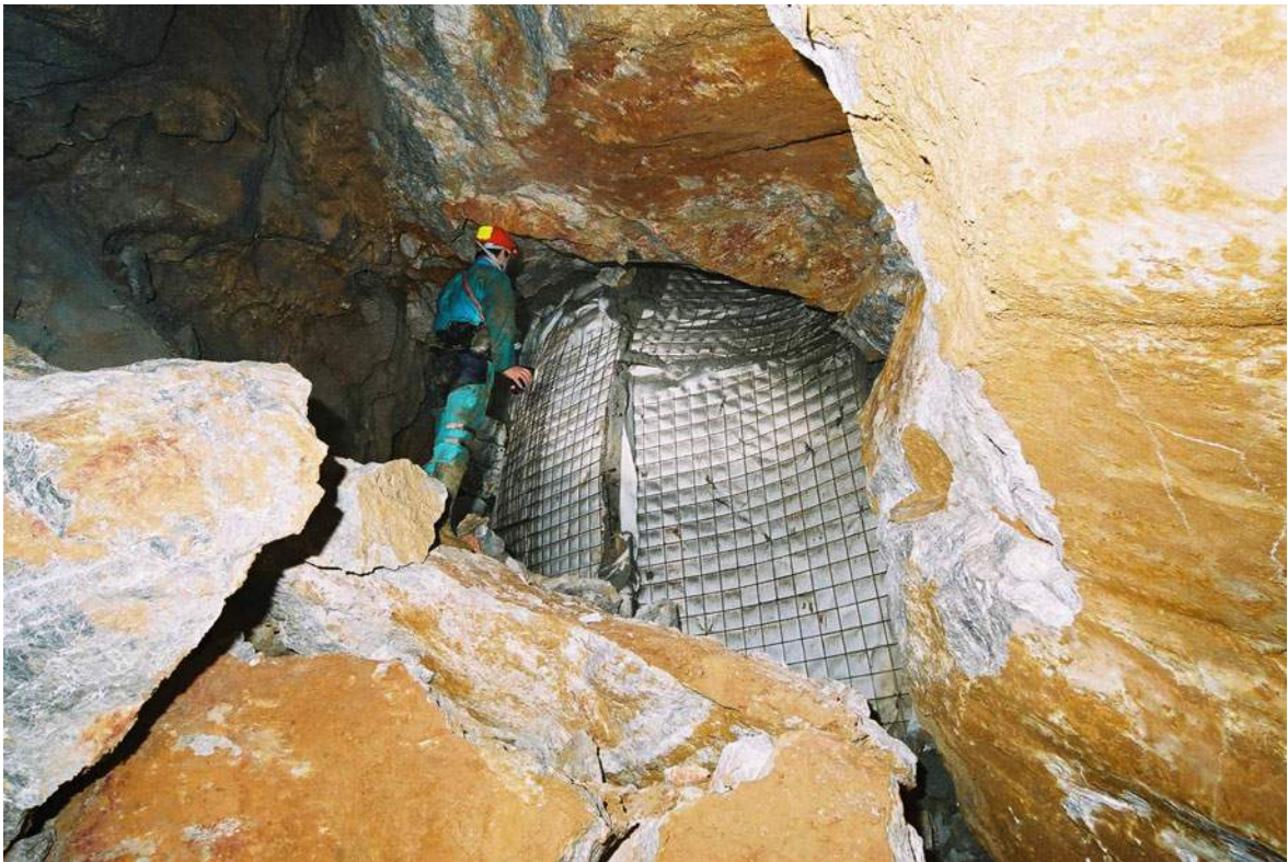
Fig. 7.62 View from Cavern at km 67 + 368 to Rožman Brdo Tunnel
