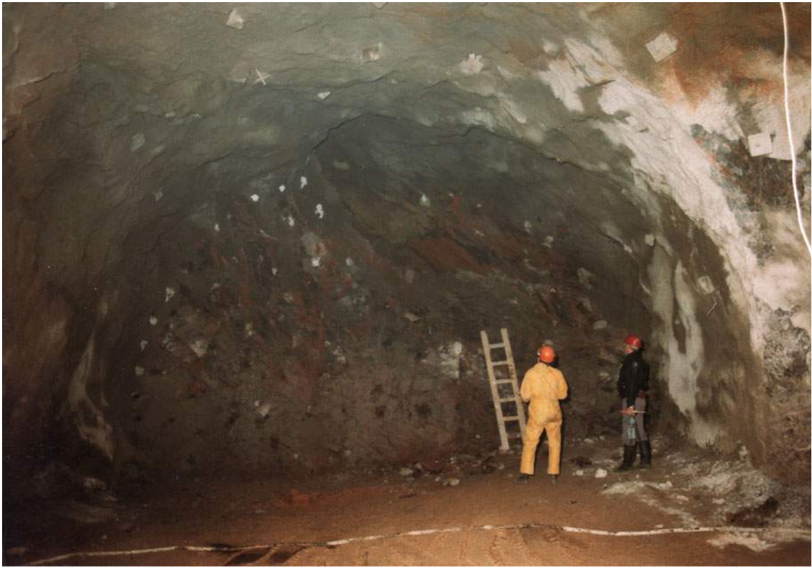
Fig. 6.20 Cavern at km 24 + 707 in Tuhobić Tunnel
