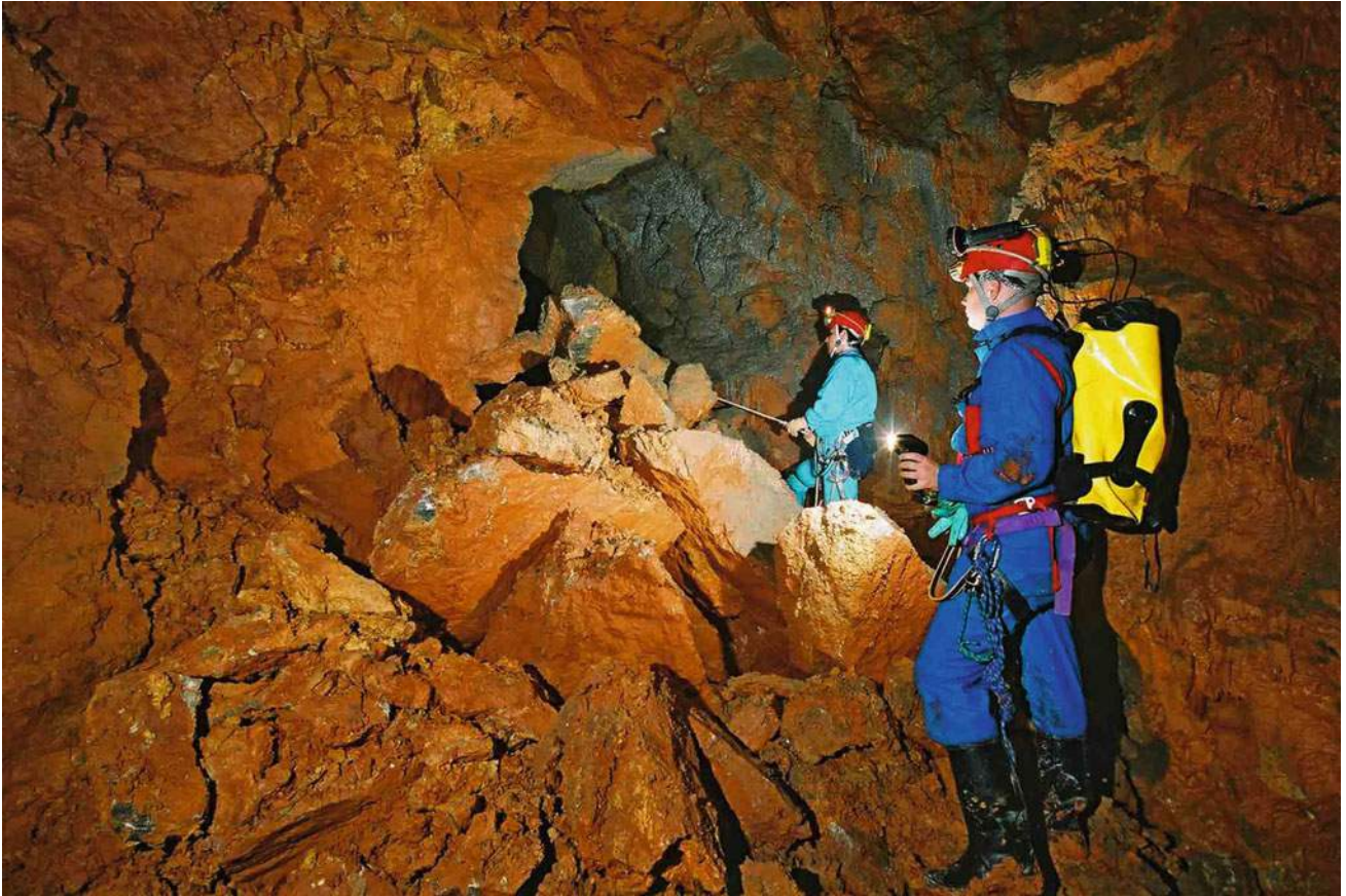
Fig. 6.77 Clay in cavern at km 59 + 166 in Čardak Tunnel
