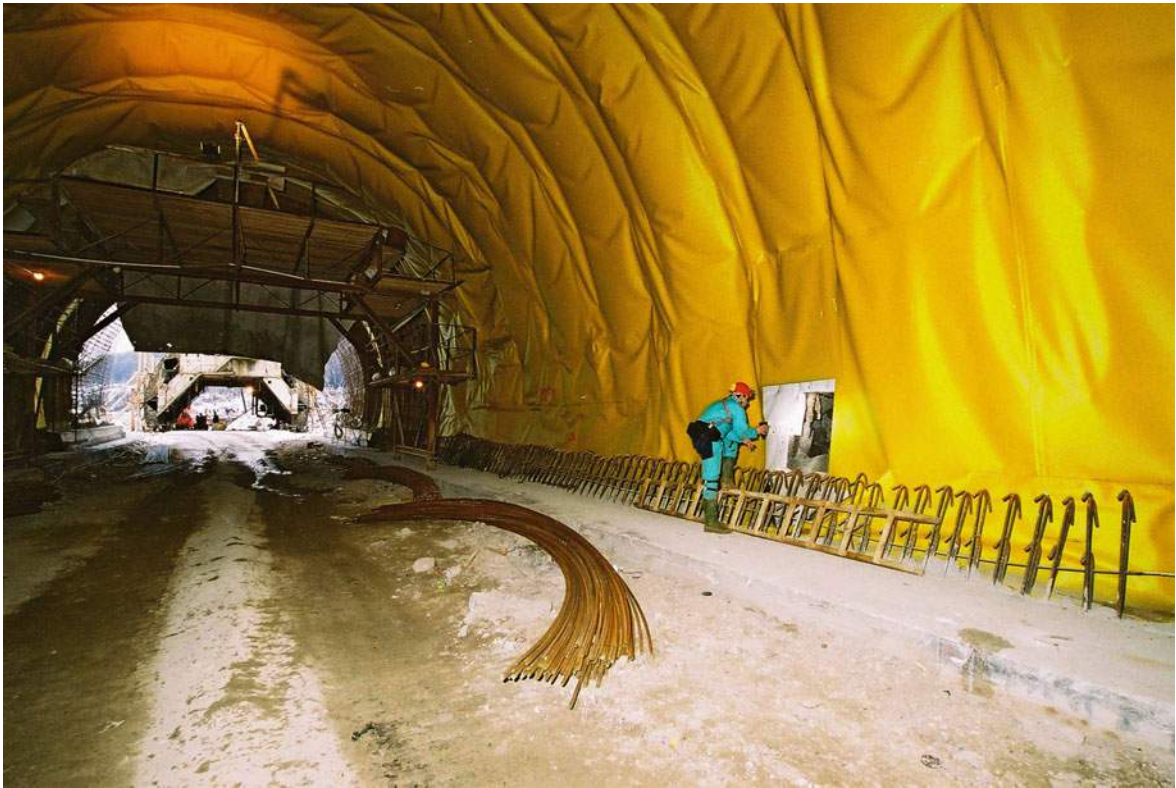
Fig. 7.61 Entrance from tunnel to cavern at km 67 + 368 in Rožman Brdo Tunnel
