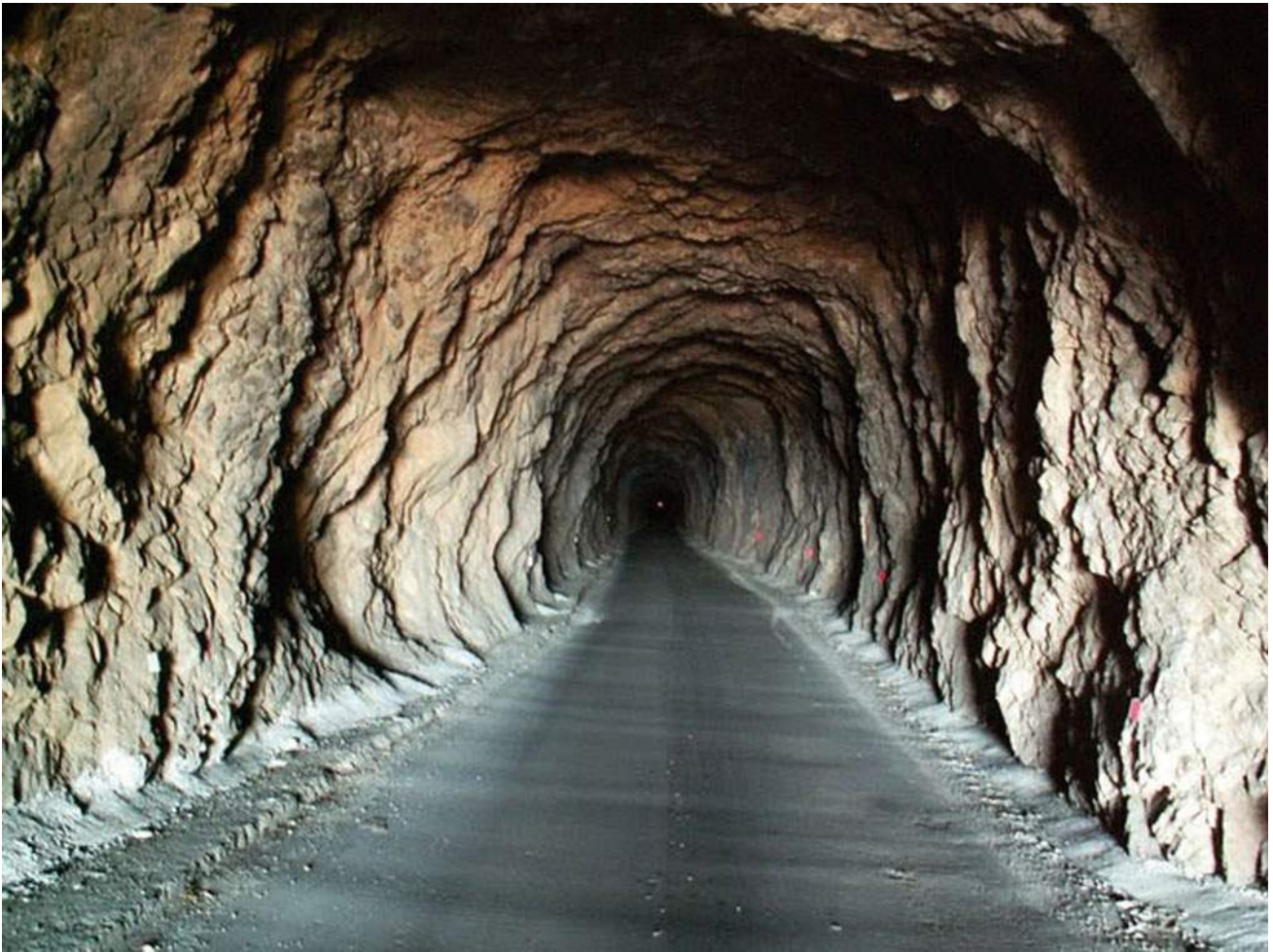
Fig. 6.1 In Pitve—Zavala tunnel, 16 smaller caverns were found in 1969
