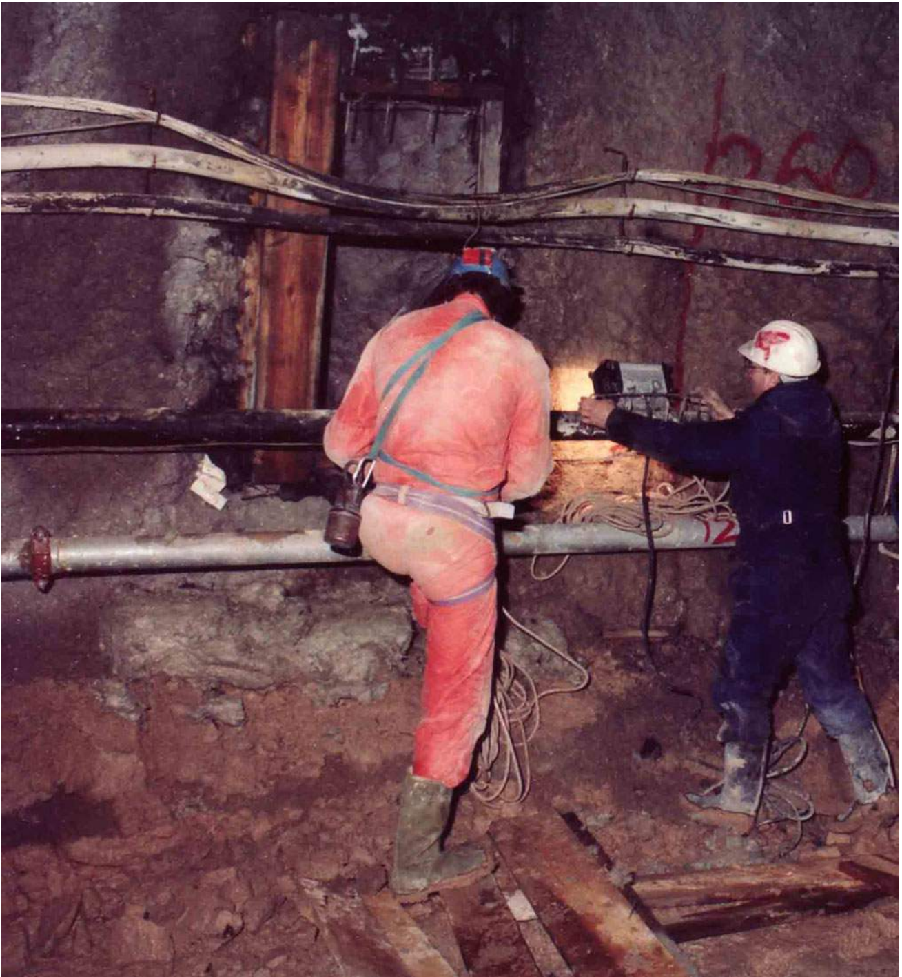
Fig. 6.26 Cavern at km 25 + 257 in Tuhobić Tunnel
