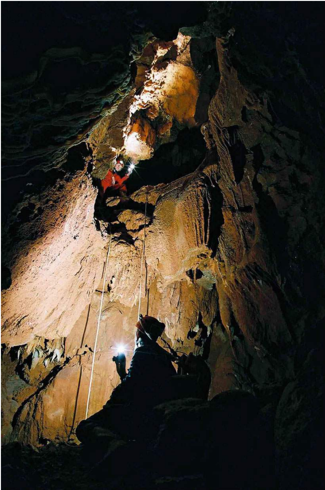
Fig. 7.34 Vertical part of cavern at km 207 + 425 in Bristovac Tunnel
