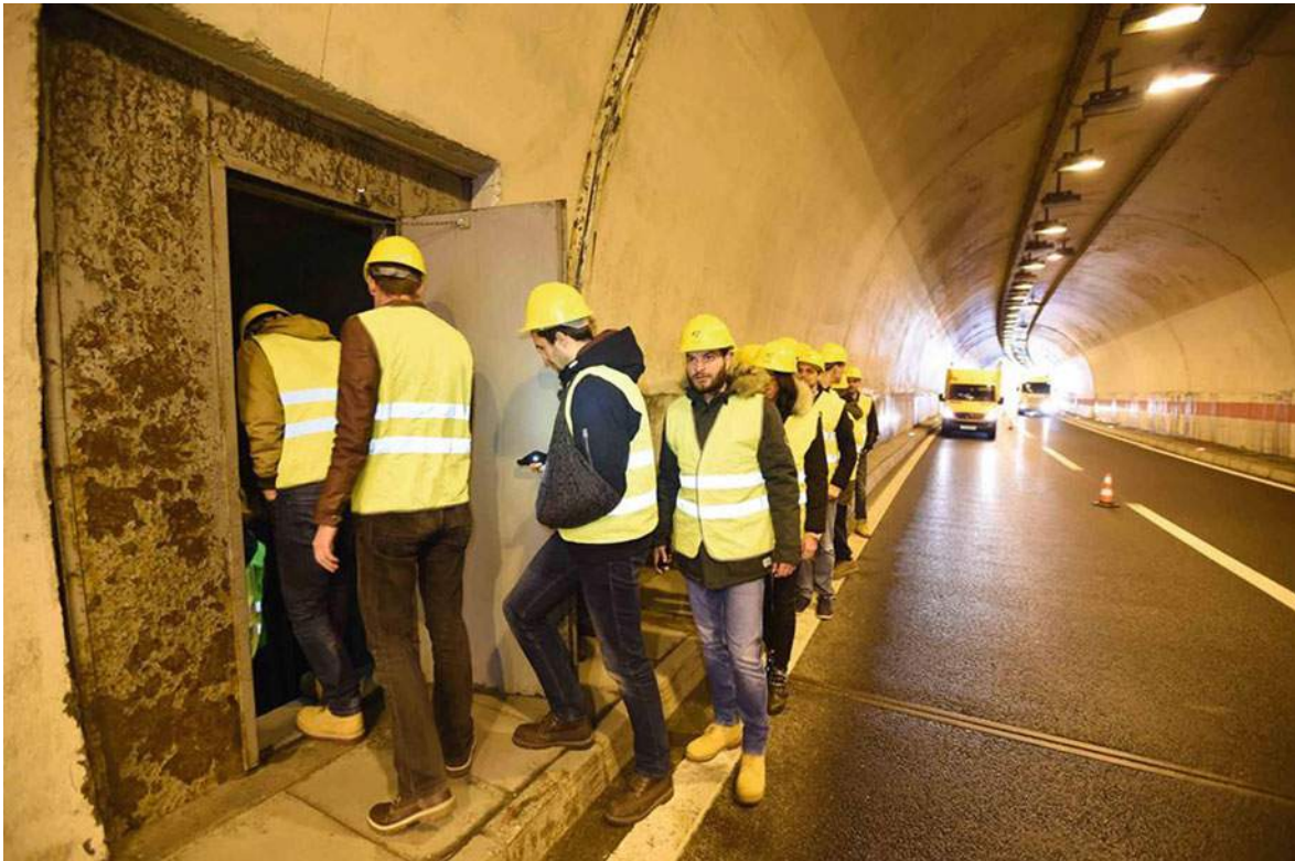
Fig. 6.69 Doors in the tunnel lining leading to the cavern
