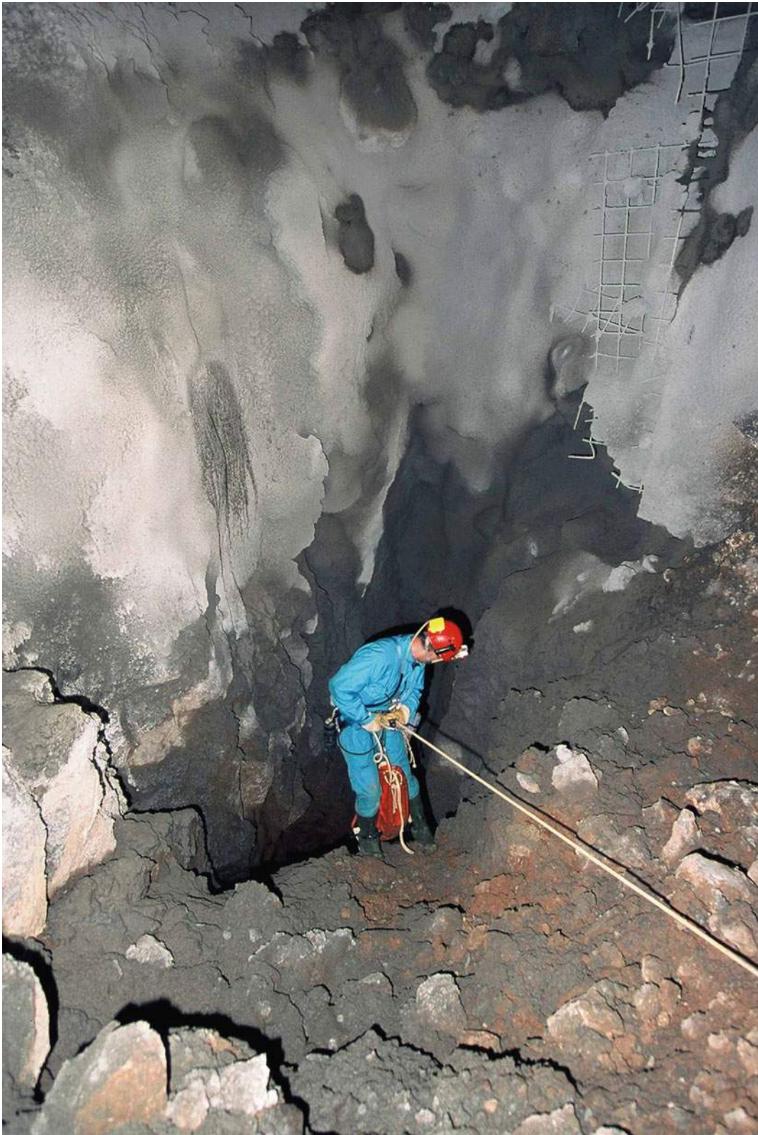
Fig. 7.40 Descending to cavern at km 0 + 634 in Grič Tunnel
