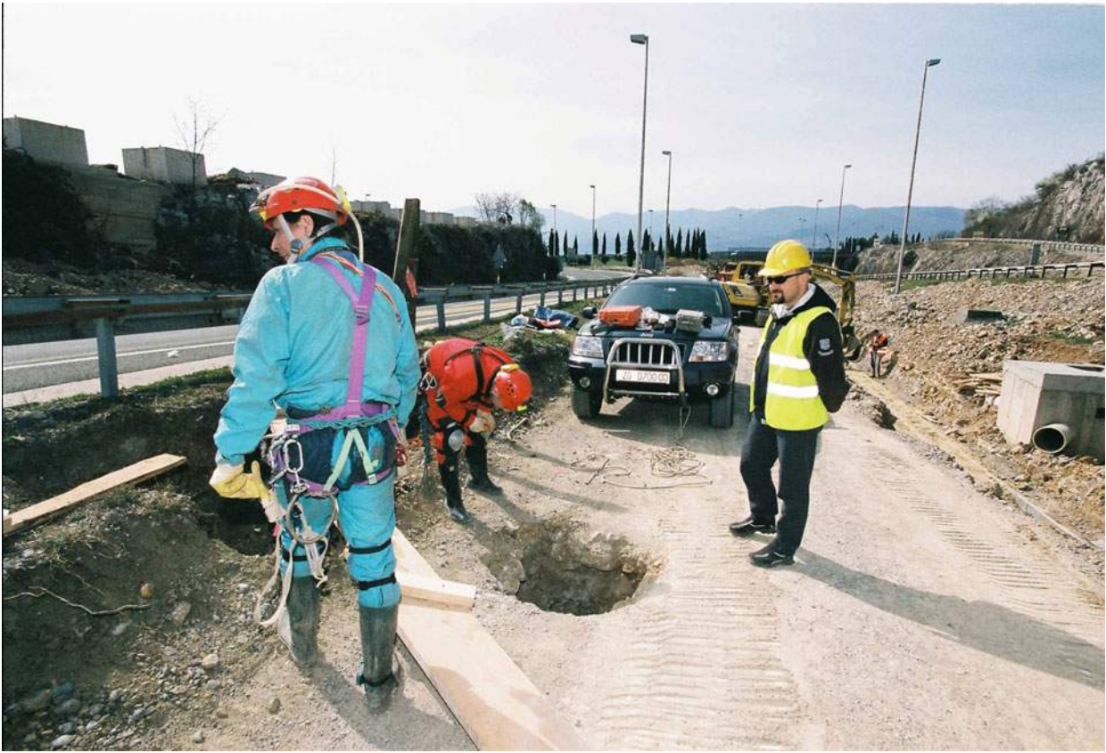
Fig. 8.47 Entrance to cavern at km 3 + 660 in Diračje road junction in Rijeka
