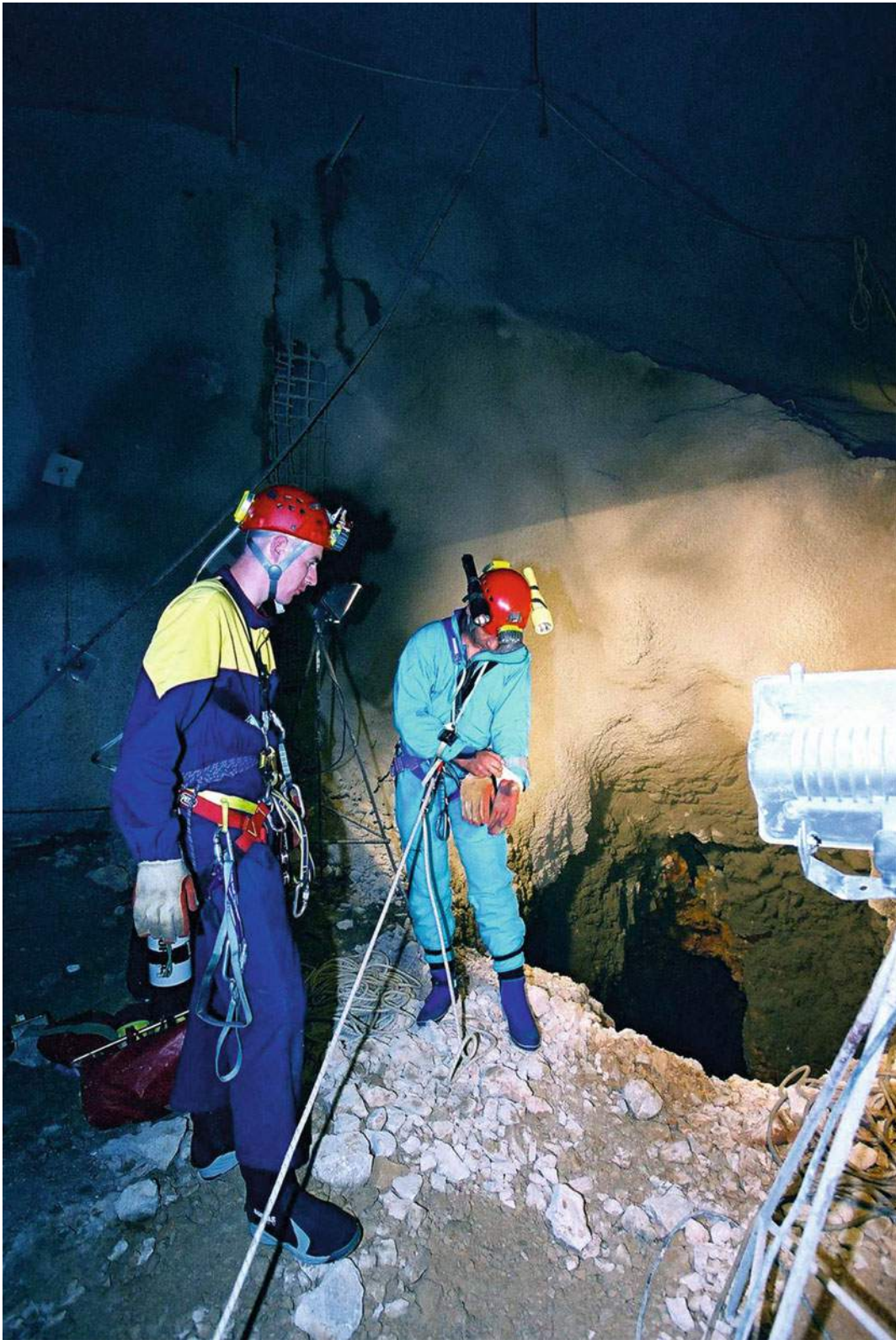
Fig. 7.55 Cavern at km 1 + 412 in Pećine Tunnel
