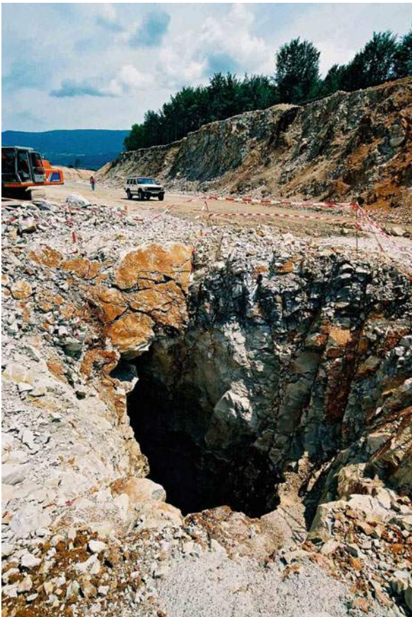
Fig. 8.59 Cavern at km 4 + 750 on A-1 highway, Mala Kapela—Žuta Lokva section
