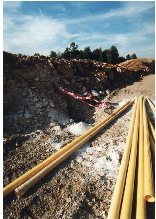
Fig. 8.25 Entrance to cavern at km 10 + 795 on Bosiljevo—Josipdol section
