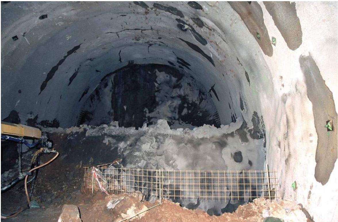
Fig. 7.39 Cavern at km 0 + 634 in Grič Tunnel
