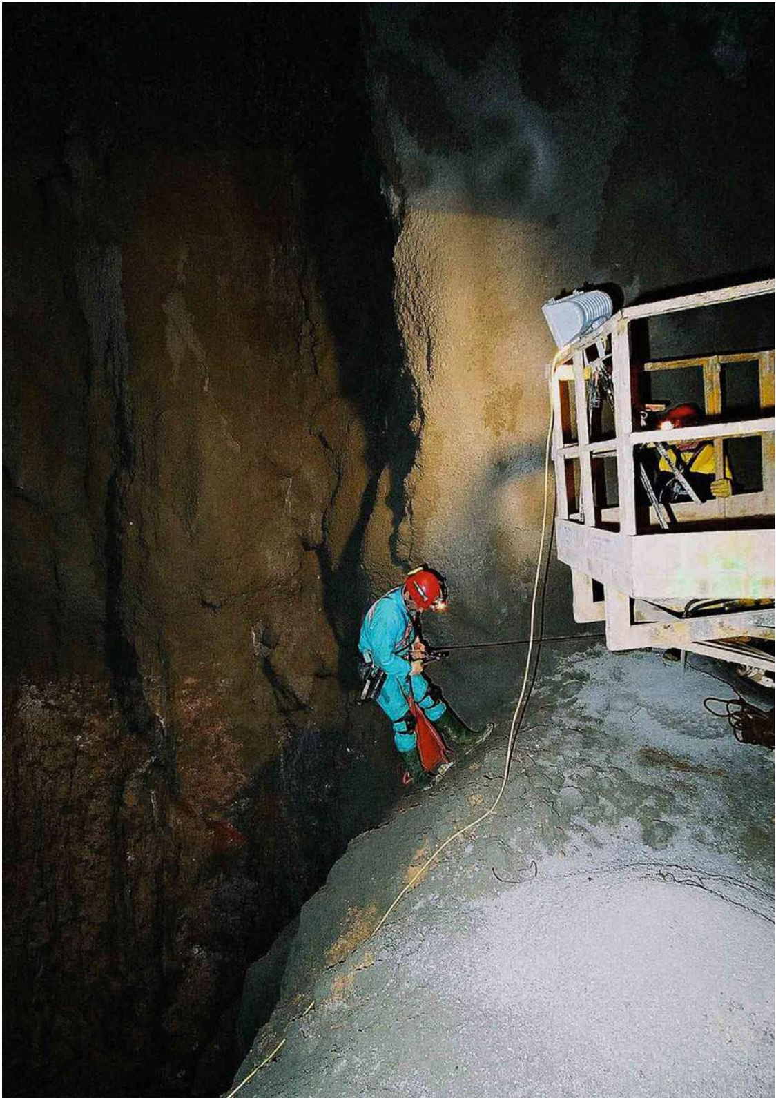
Fig. 7.43 Descending to cavern at km 14 + 027 in Brinje Tunnel
