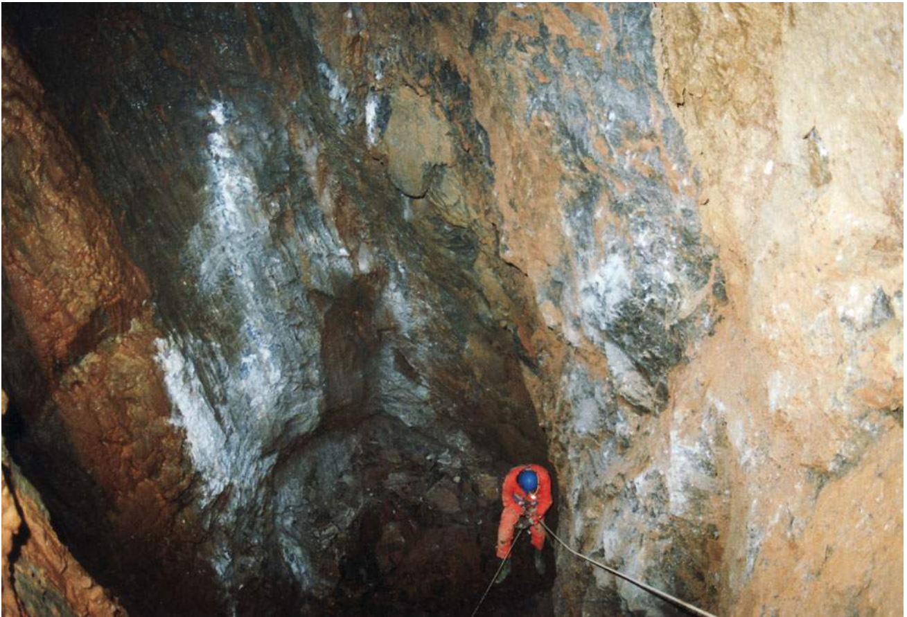
Fig. 6.37 Cavern at km 35 + 532 in Sleme Tunnel
