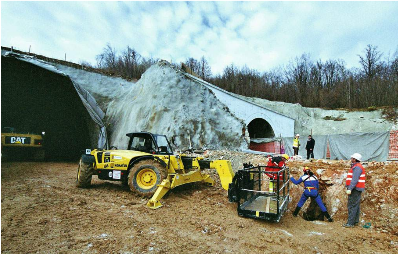
Fig. 6.80 Cavern in front of the portal of Hrasten Tunnel
