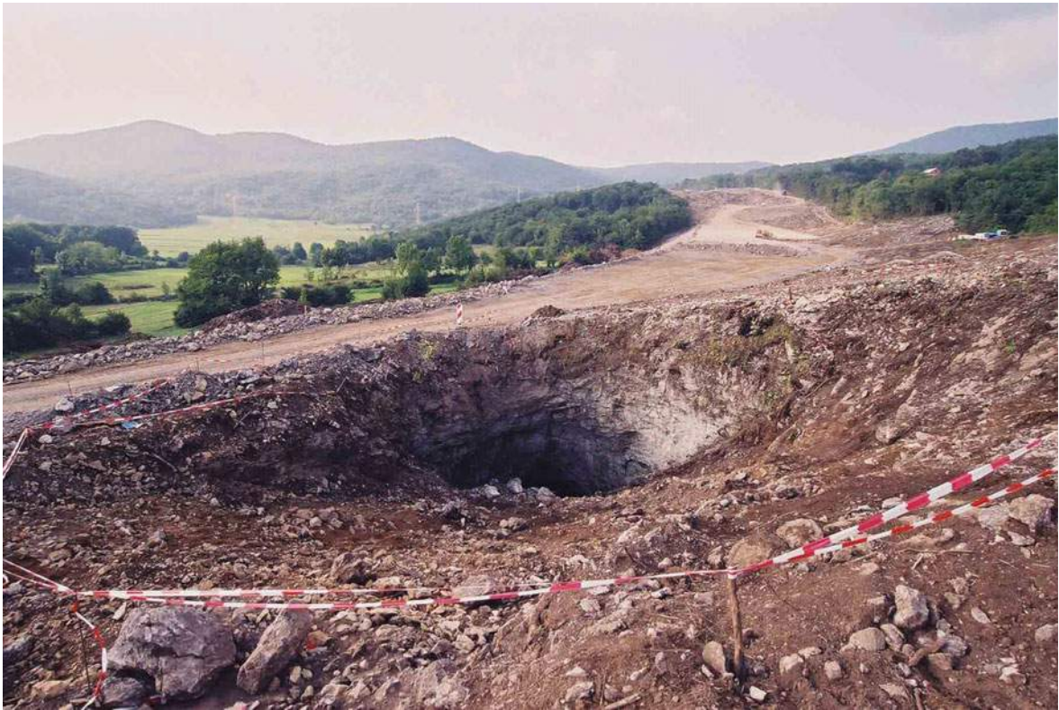
Fig. 8.56 Cavern at km 0 + 920 on A-1 highway, Mala Kapela—Žuta Lokva section
