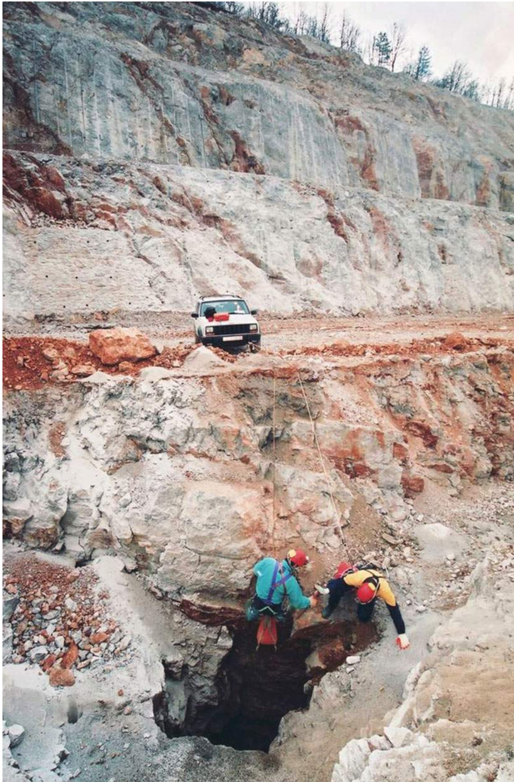
Fig. 8.63 Cavern at km 28 + 760 on A-1 highway, Ličko Lešće—Lički Osik section
