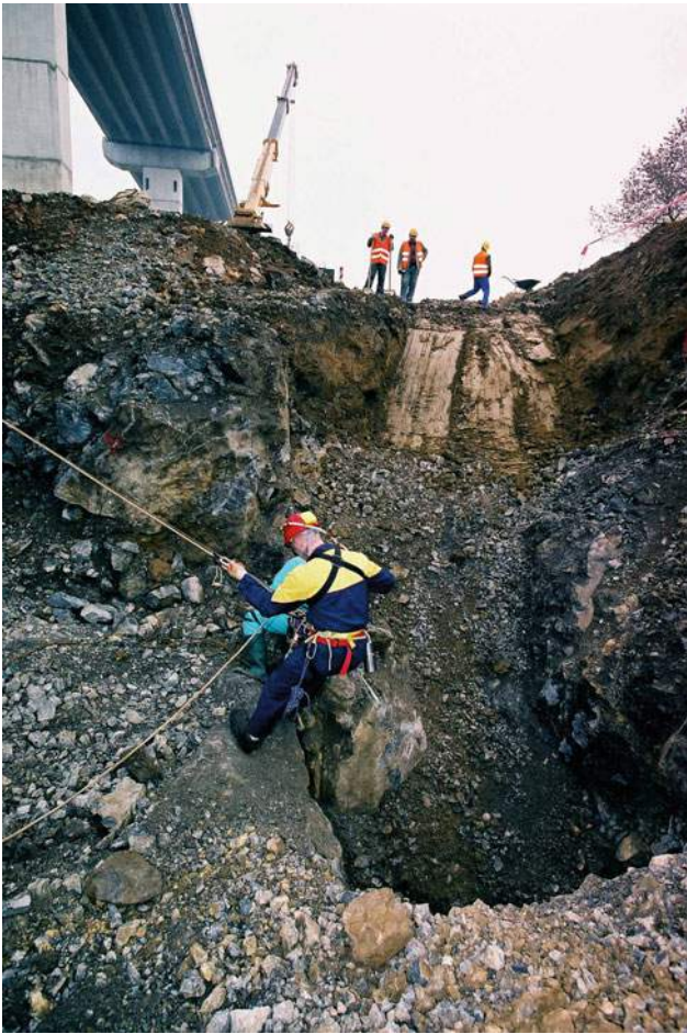
Fig. 8.5 Cavern at km 76 + 955 under pillar S-6, right of Osojnik Viaduct
