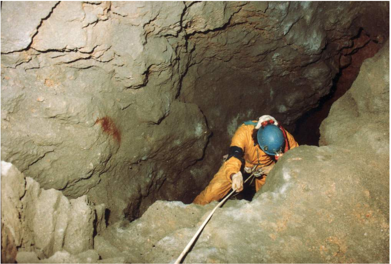
Fig. 6.49 Cavern at km 38 + 782 in Sopač Tunnel
