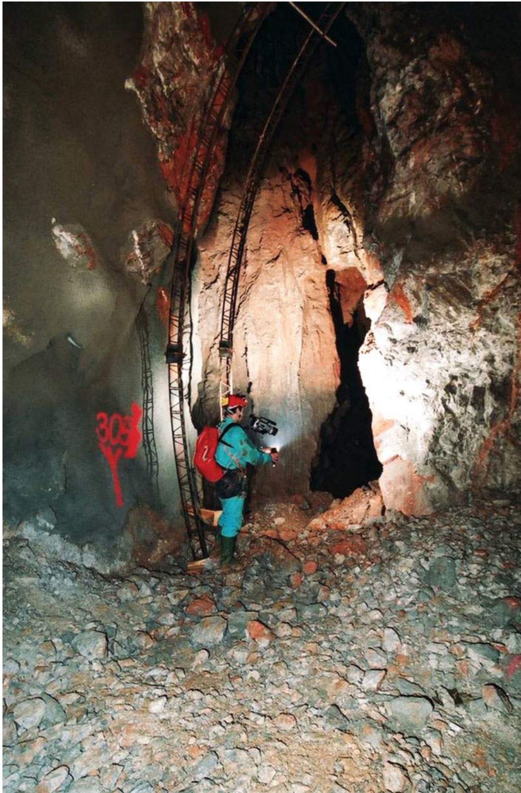
Fig. 7.36 Cavern at km 19 + 939 in Plasina Tunnel
