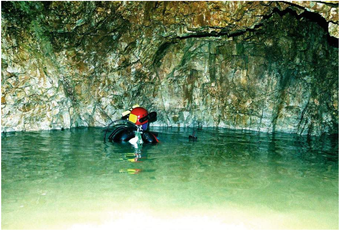
Fig. 7.58 Cave diving in lake in cavern at km 1 + 412 in Pećine Tunnel
