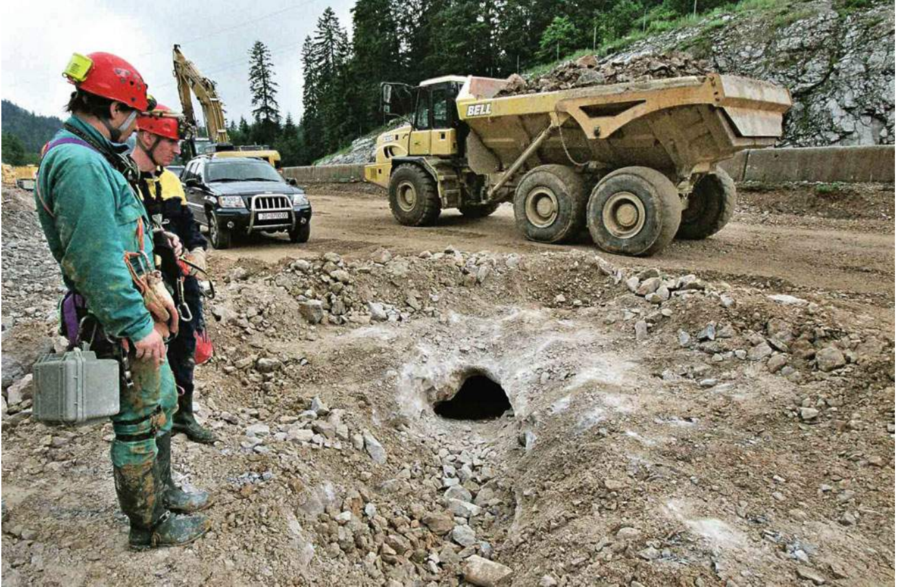
Fig. 6.82 Cavern at km 41 + 262 in front of the Lučice Tunnel
