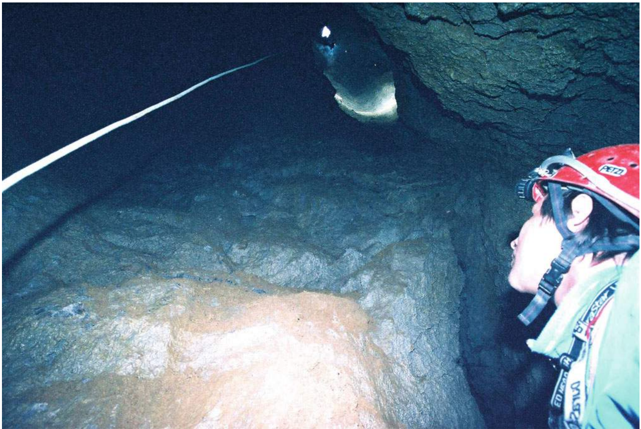
Fig. 8.4 Cavern at km 70 + 510 under pillar S-7 of Zečeve Drage Viaduct
