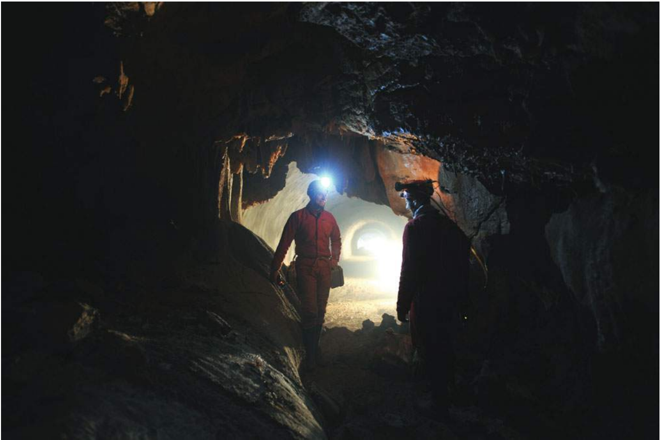
Fig. 7.67 Cavern at km 1 + 965 in Puljani Tunnel (view from cavern to tunnel)
