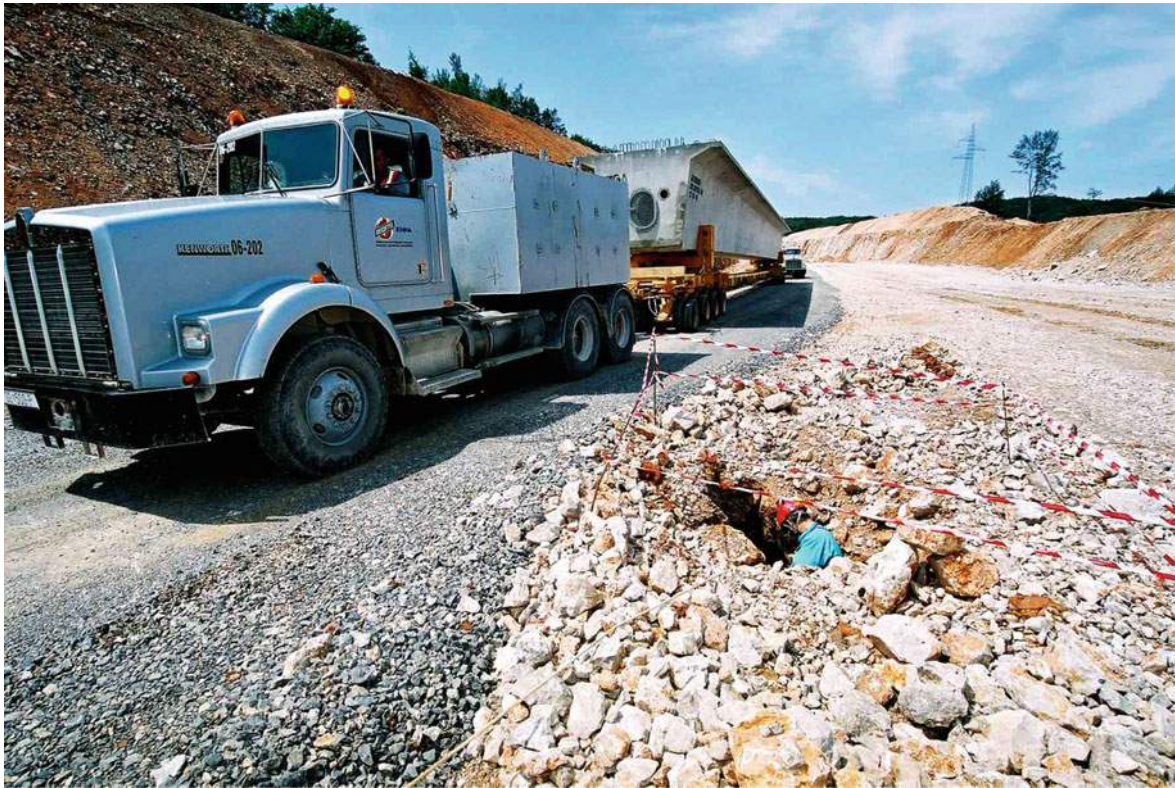
Fig. 8.58 Cavern at km 3 + 168 on A-1 highway, Mala Kapela—Žuta Lokva section
