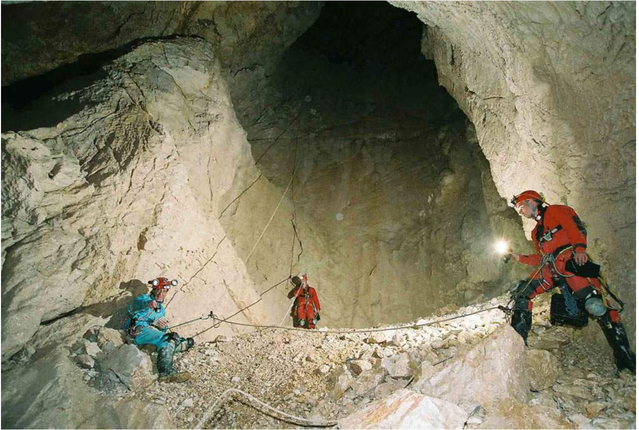
Fig. 7.53 Lower parts of cavern at km 1 + 637 in Sveti Ilija Tunnel
