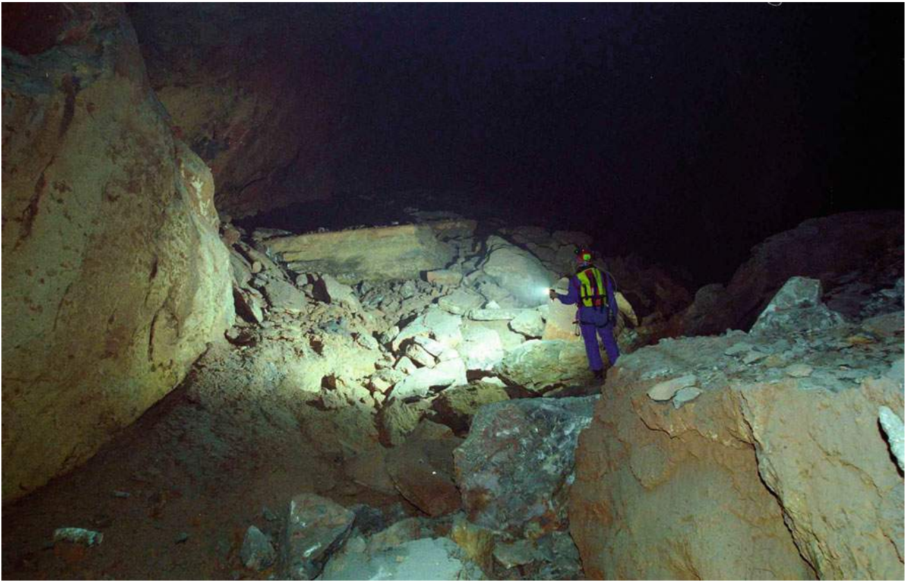
Fig. 7.19 Cavern at km 200 + 525 in Sveti Rok Tunnel
