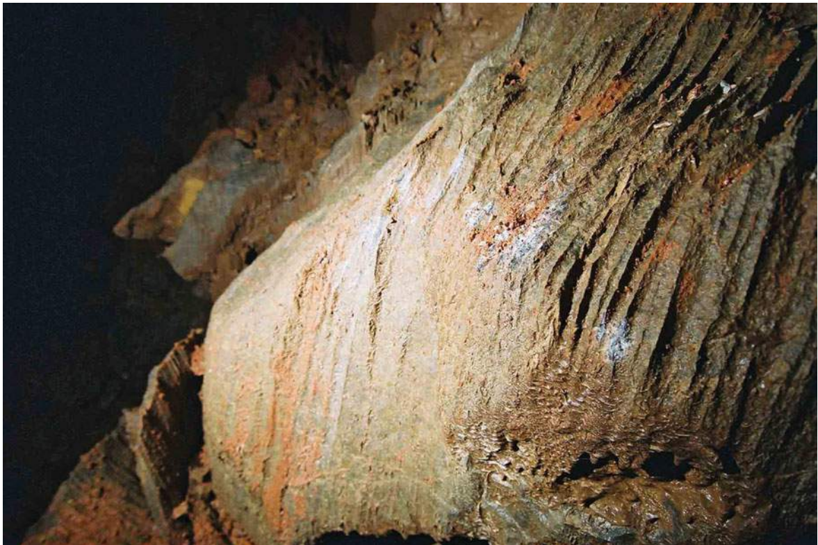
Fig. 7.59 Cave karren in cavern at km 66 + 926 in Rožman Brdo Tunnel
