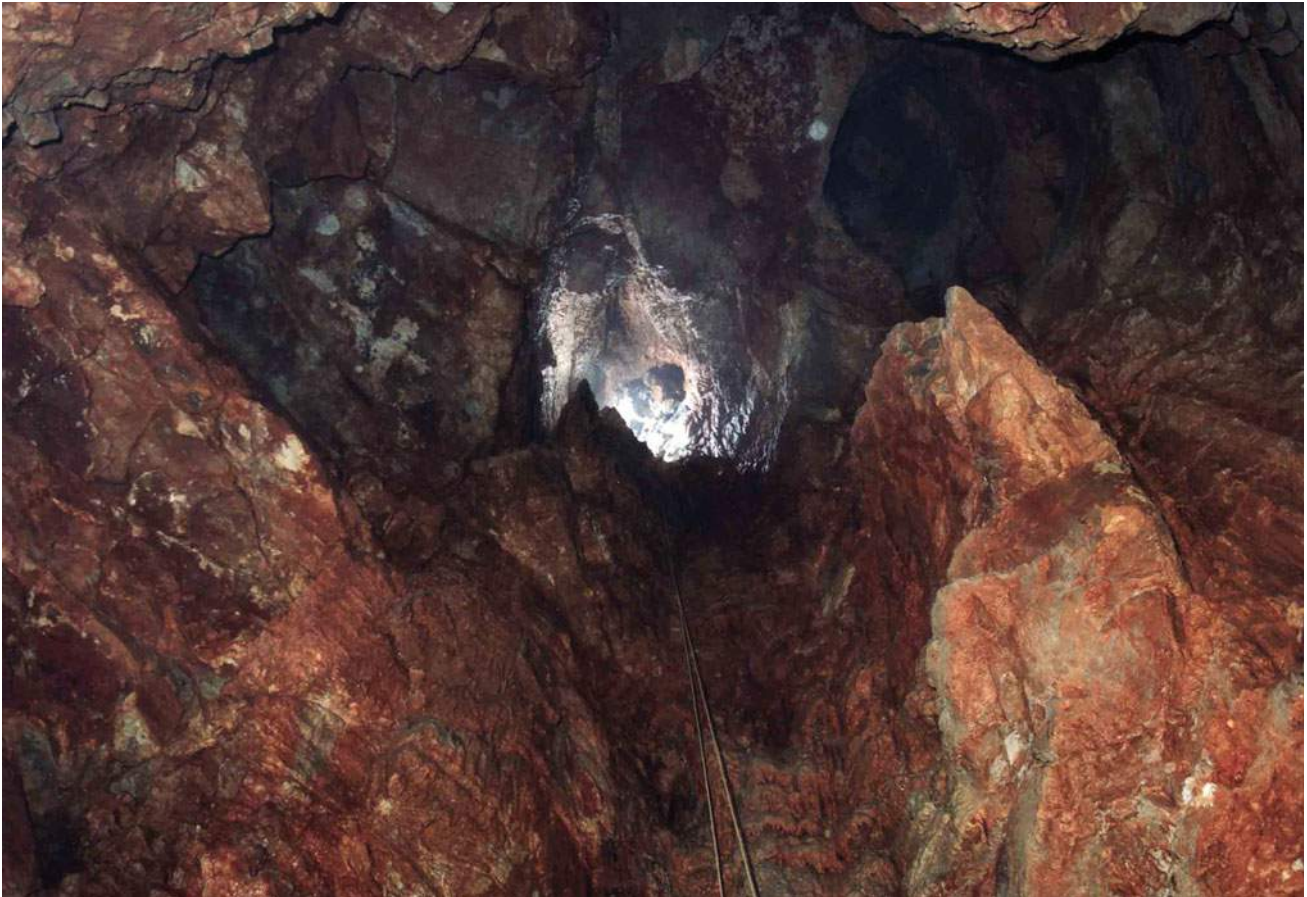
Fig. 6.57 Cavern at km 47 + 412 in Vršek Tunnel
