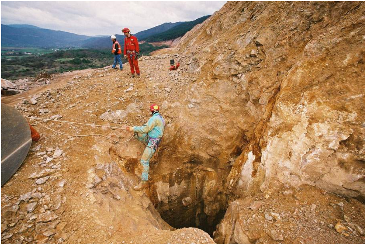
Fig. 8.61 Cavern at km 13 + 625 on A-1 highway, Žuta Lokva—Ličko Lešće section
