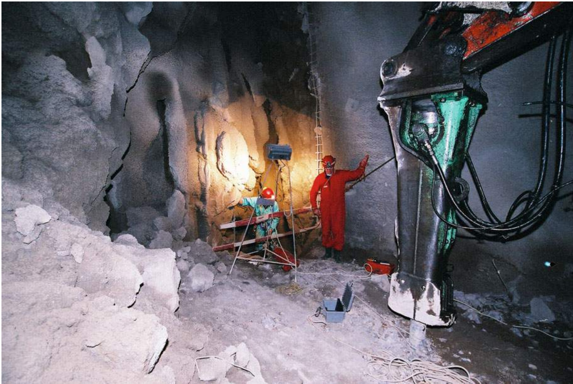
Fig. 6.30 Cavern entrance covered with sprayed concrete
