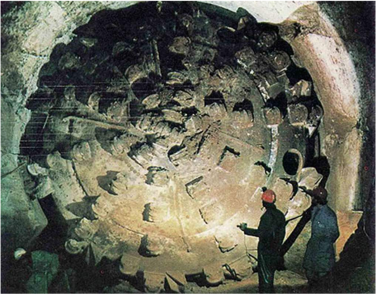
Fig. 5.21 Tunnel Boring Machine in one of the caverns in Zakučac tunnel
