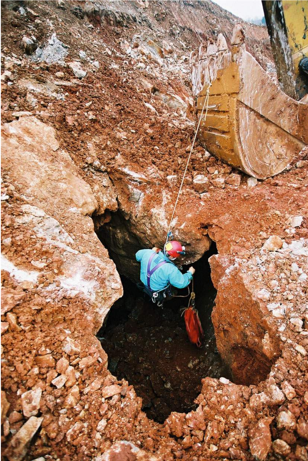
Fig. 8.62 Cavern at km 18 + 350 on A-1 highway, Žuta Lokva—Ličko Lešće section
