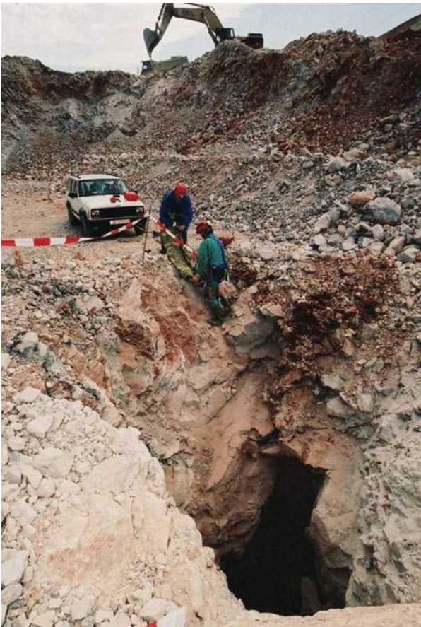
Fig. 8.57 Cavern at km 4 + 528 on A-1 highway, Mala Kapela—Žuta Lokva section
