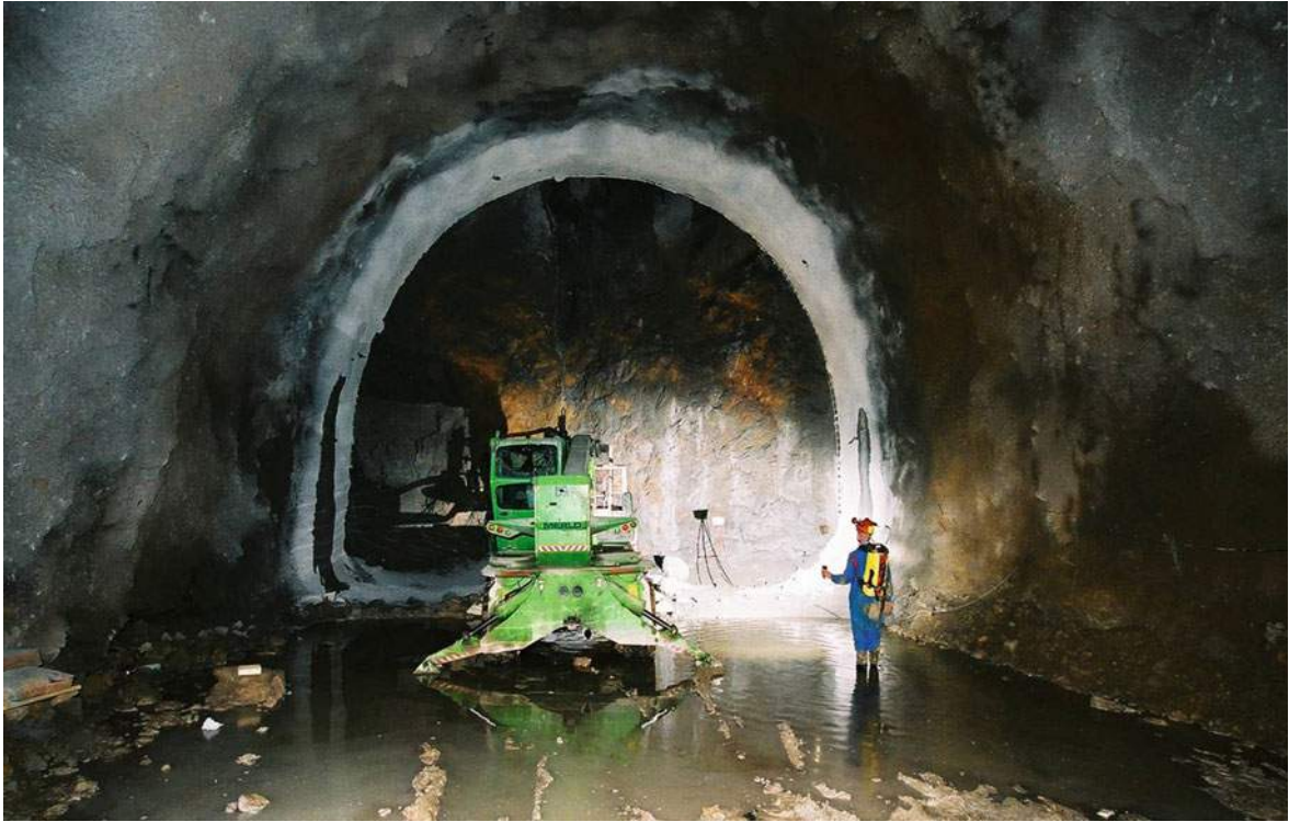
Fig. 6.71 Cavern in Veliki Gložac Tunnel
