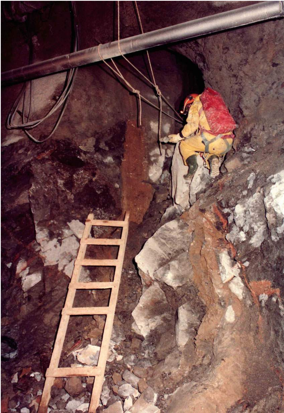
Fig. 6.27 Fault zone with clay material and cavern
