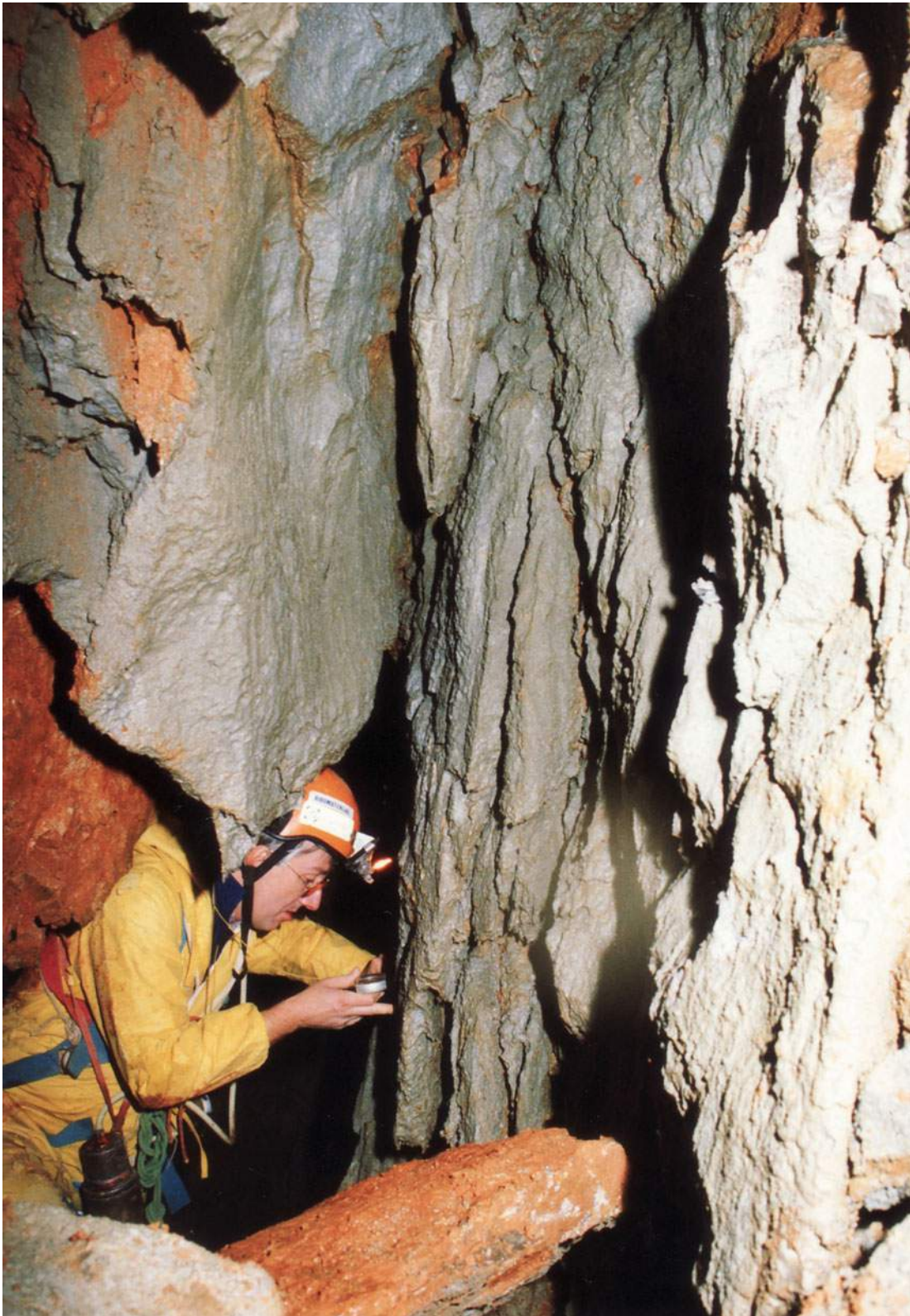
Fig. 6.17 Cavern at km 24 + 544 in Tuhobić Tunnel
