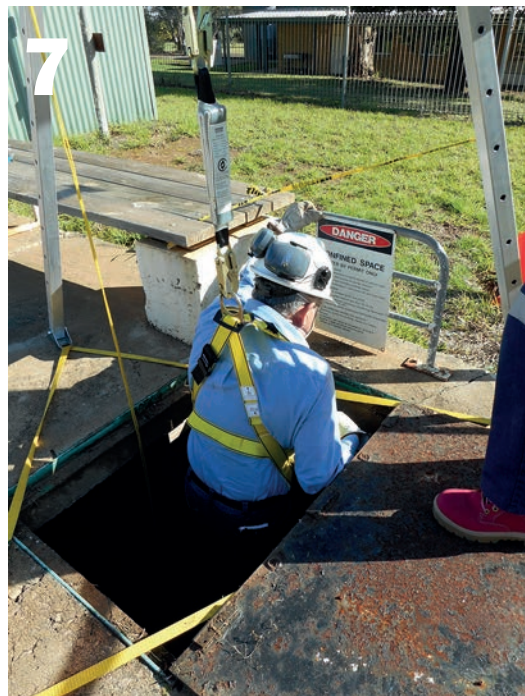
7 Worker or Standby Person lowering worker into vertical entry confined space.
