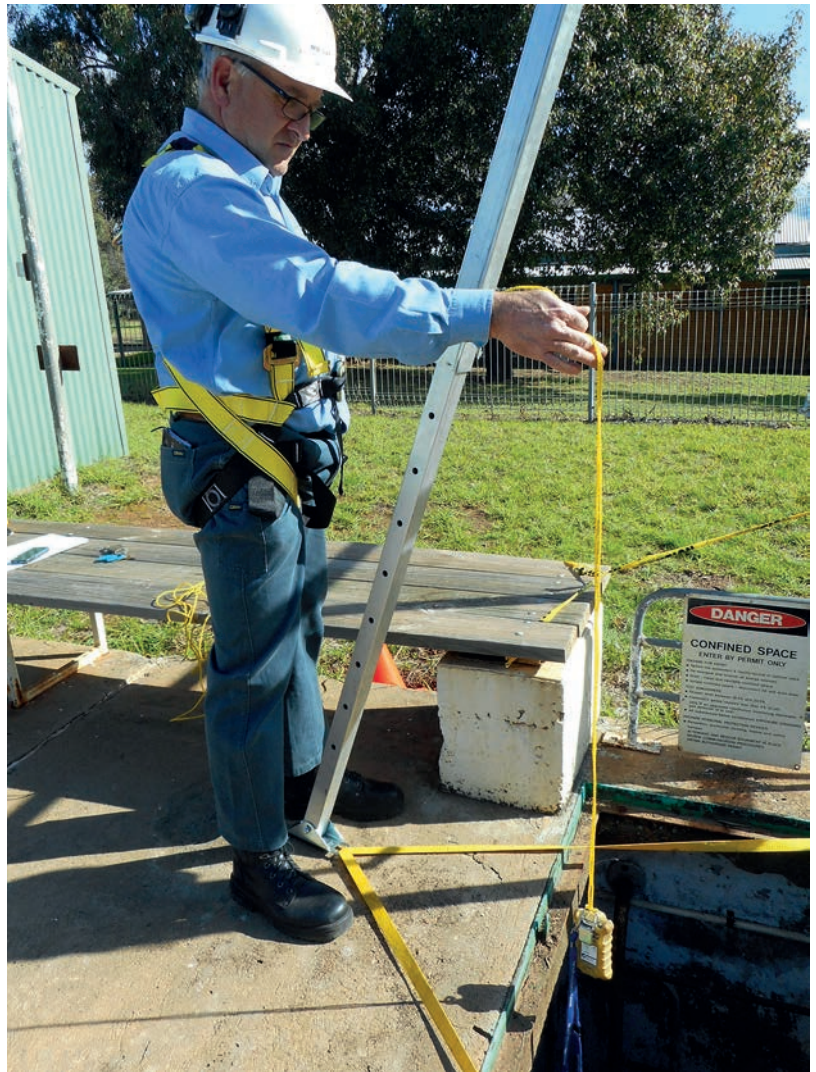
Example of gas testing a confined space with a vertical entry.
