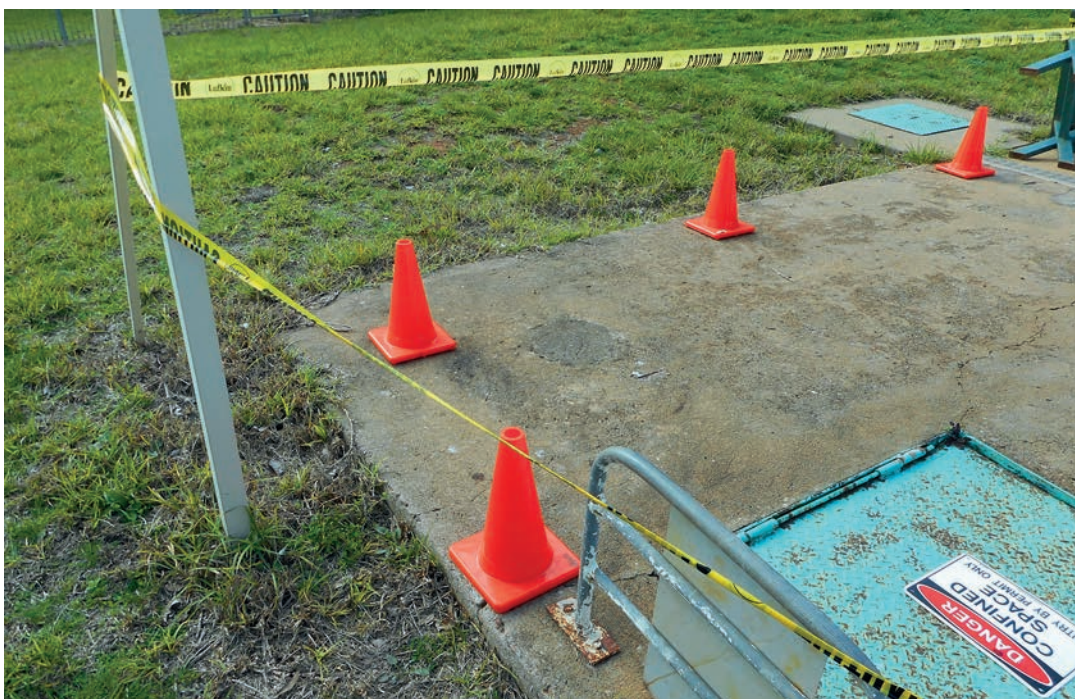
Using cones and barrier tape to secure the perimeter of a confined space.
