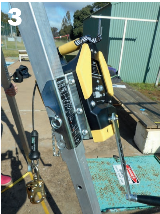
3 Attach personnel-rated hoist to the tripod.
