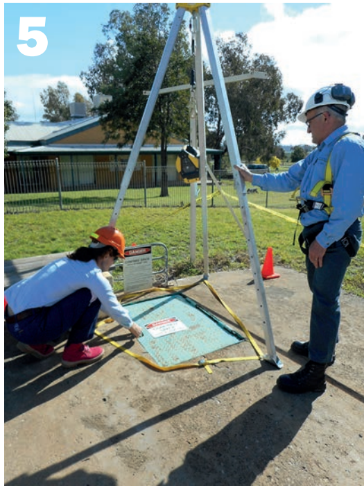
5 Position tripod over confined space entry point.
