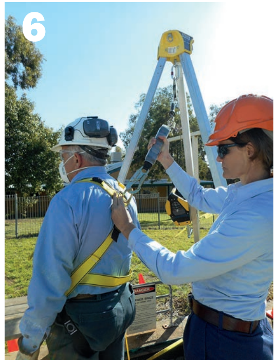
6 Attach a shock absorbing lanyard to worker's harness.
