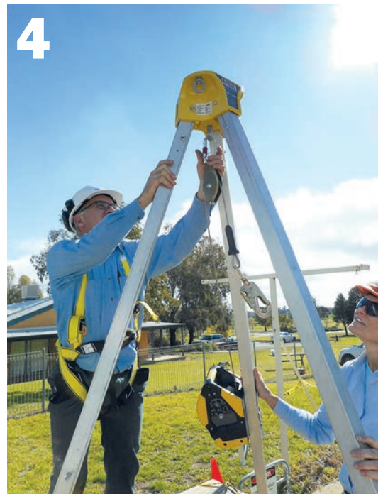
4 Attach hoist to connector on tripod and make any final adjustments to tripod height.
