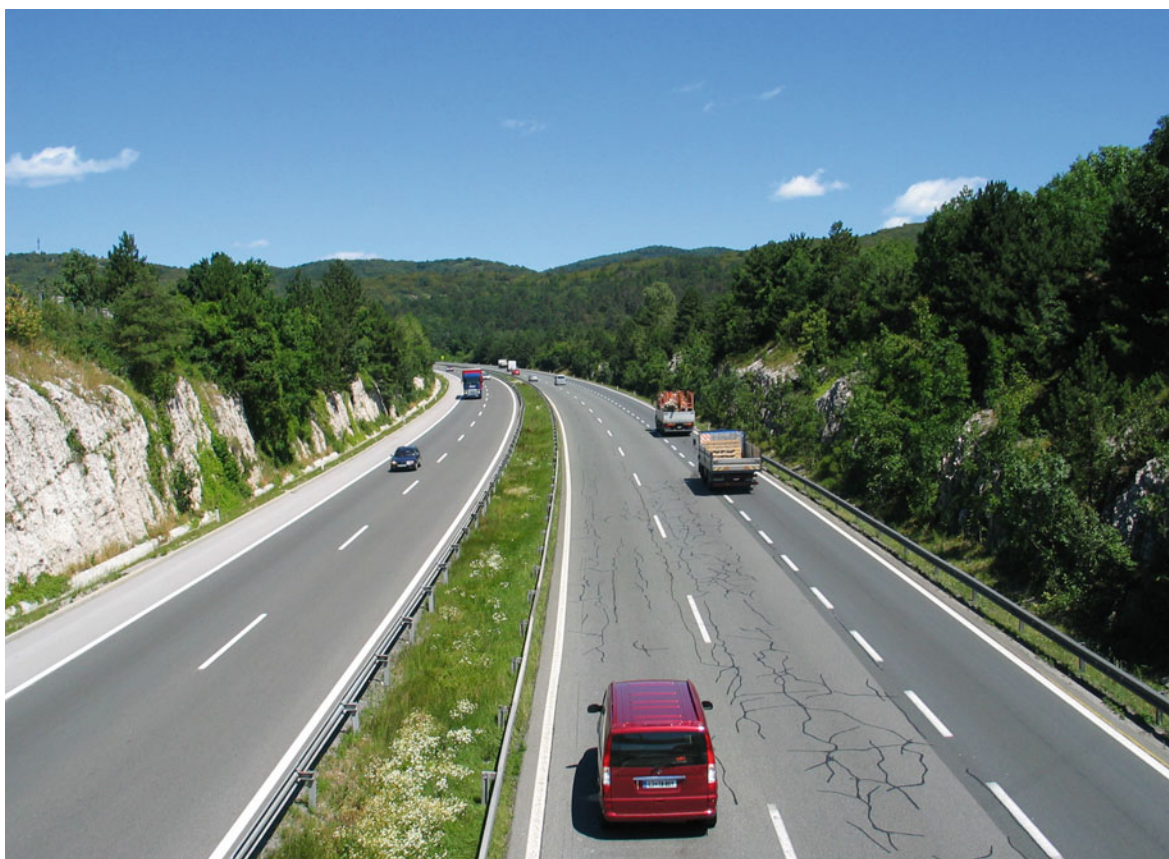
Fig. 27.2 Revealed karst rock in the roadcut of the motorway
