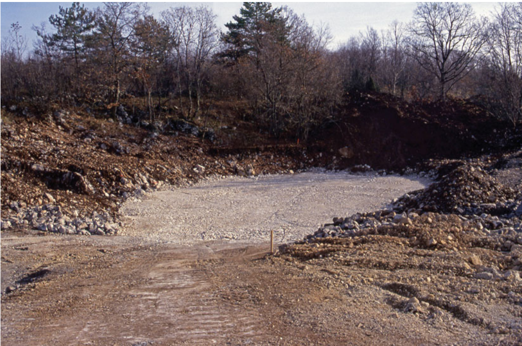
Fig. 1.6 Filling a doline (which now lies below the motorway) with rubble
