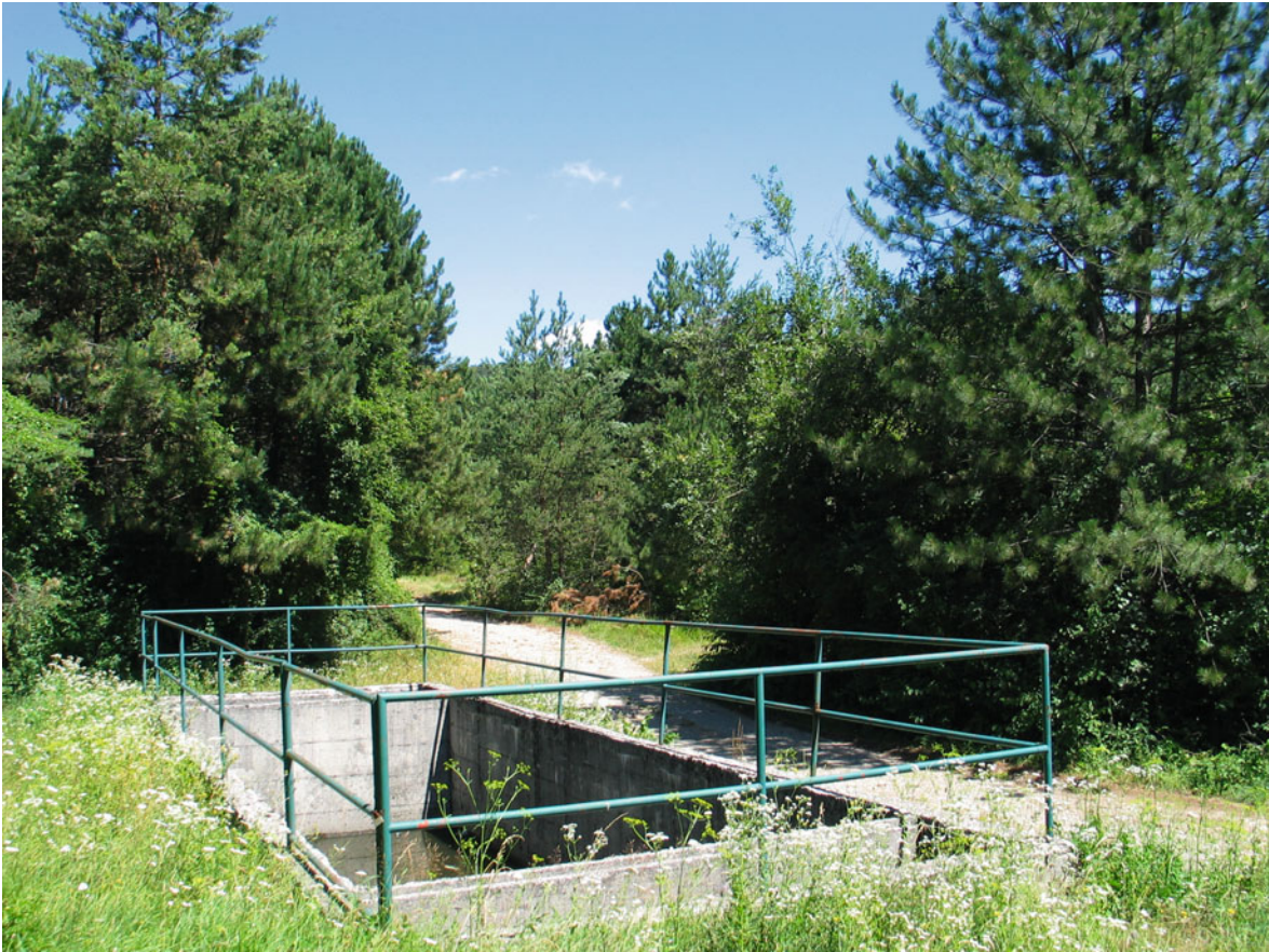
Fig. 28.3 Oil separator at the village of Stara vas
