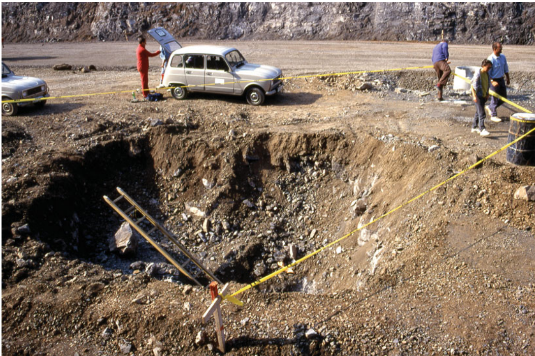
Fig. 6.16 A road collapse
