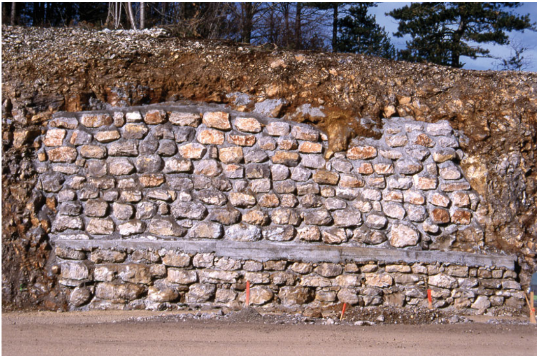
Fig. 1.14 Closing a cave in the embankment of a roadcut
