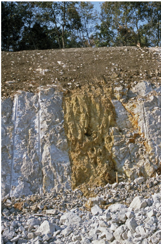
Fig. 2.10 An old shaft filled with fine-grained alluvium
