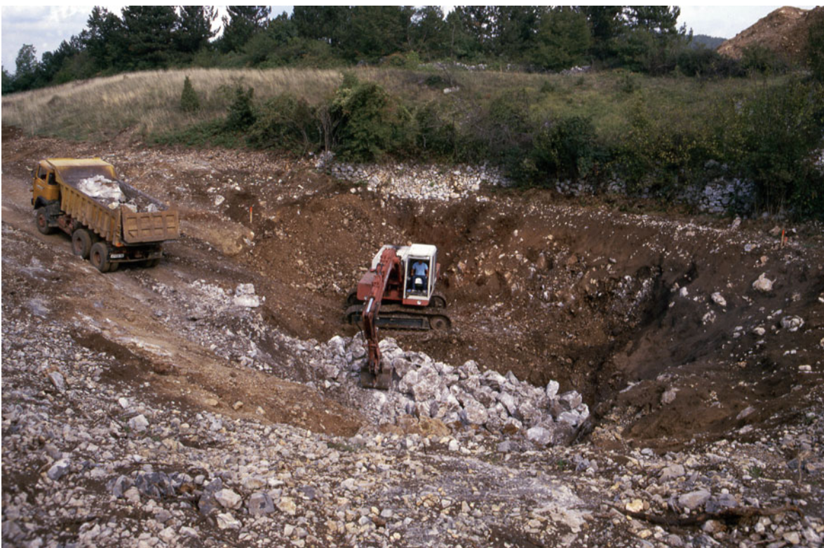
Fig. 6.1 Removing soil and sediments from a filled up doline
