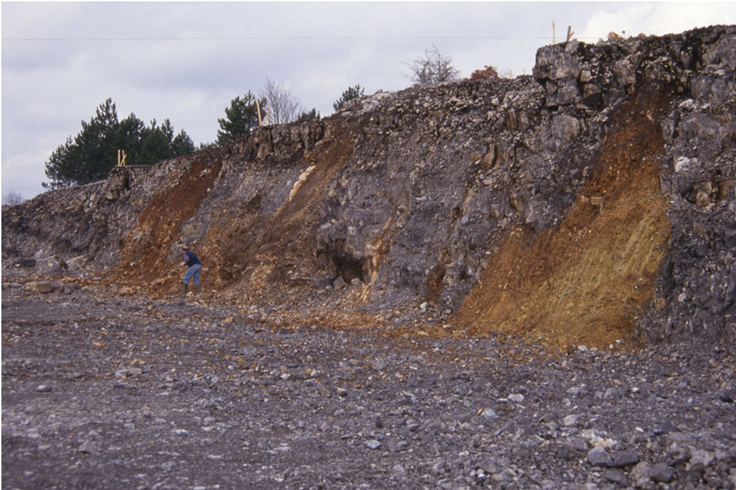
Fig. 6.8 Caves filled with alluvia in the embankment of a motorway roadcut
