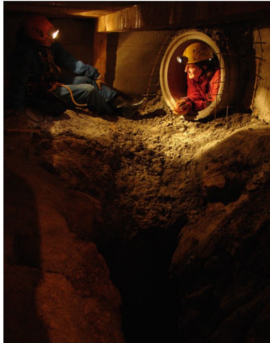
Fig. 16.10 A concrete tube connects the Igorjeva groza Cave to the motorway embankment
