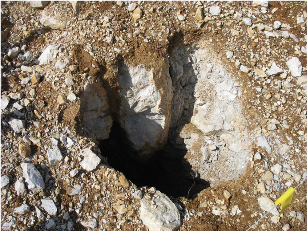
Fig. 18.5 The entrance to the shaft on the road route
