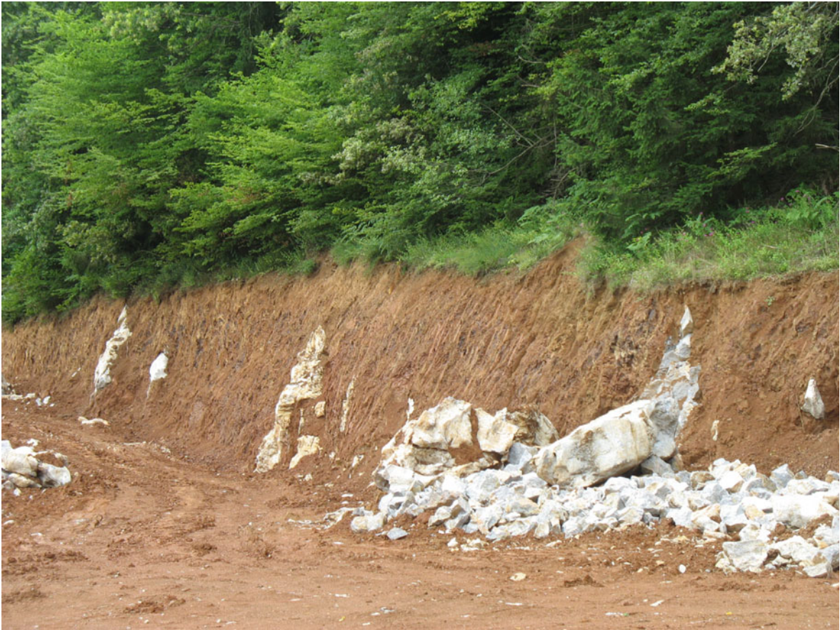
Fig. 18.3 Subsoil stone teeth within a thicker layer of soil and alluvium
