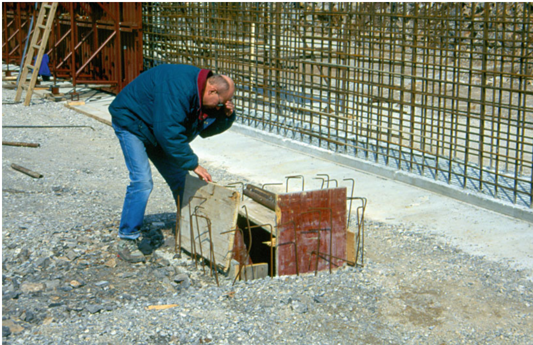
Fig. 1.16 Construction of a road-side artificial entrance
