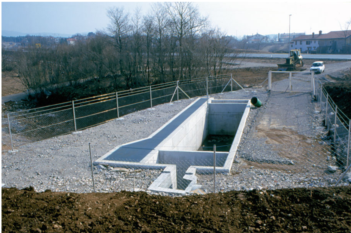
Fig. 1.19 Construction of an oil separator
