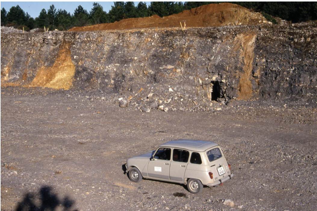
Fig. 6.9 Hollow and alluvium-filled caves uncovered during excavation works for the motorway roadcut
