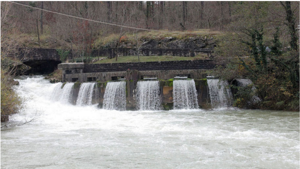
Fig. 27.4 The Spring of the Rižana River, captured in order to provide the coastal population with drinking water
