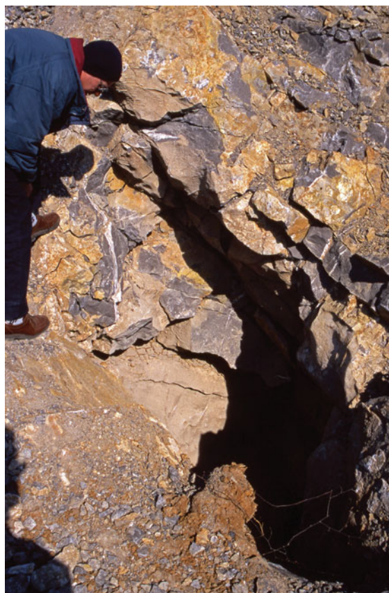
Fig. 23.6 A shaft which opened during excavation works for the roadcut
