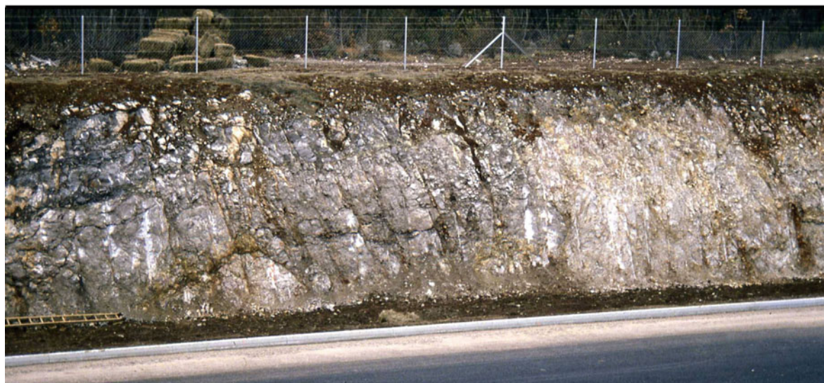
Fig. 14.1 The profile along the Divača-Kozina motorway section. Legend 1 limestones of the Lipica Formation (Upper Santonian); 2 bottom red horizon; 3 upper red horizon, direct base of the paleokarst surface; 4 series of horizontal centimetre-to decimetre-scale cavities, filled with brown silt; 5 paleokarst surface, contact area between the altered limestones of the Lipica Formation and the weathered zone; 6
