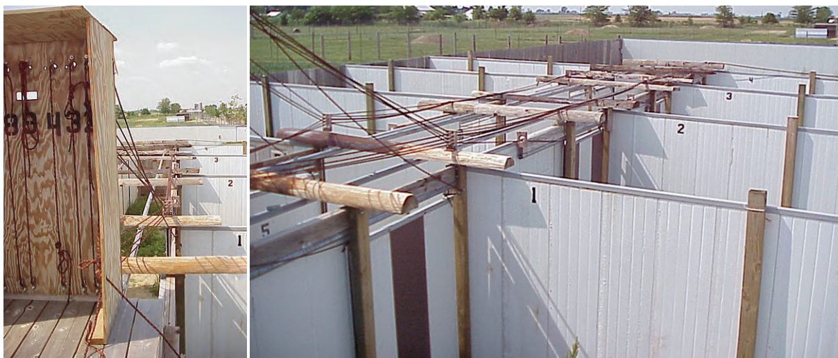
• Fig. 1.10 Deer-holding working facilities with individual stalls with solid walls and automatic doors.
