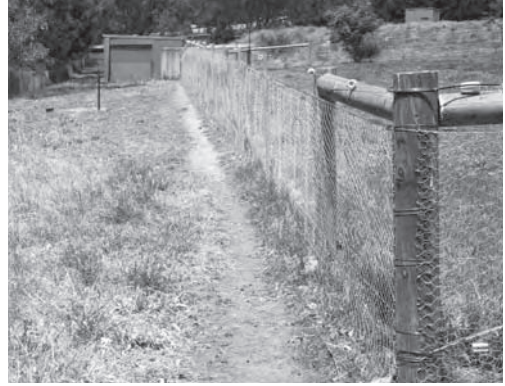
Rabbit proof netting fence with electric top wire, treated pine corner assembly.
