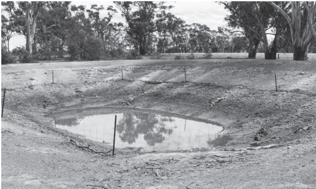
Fence off and check unsafe dams.
