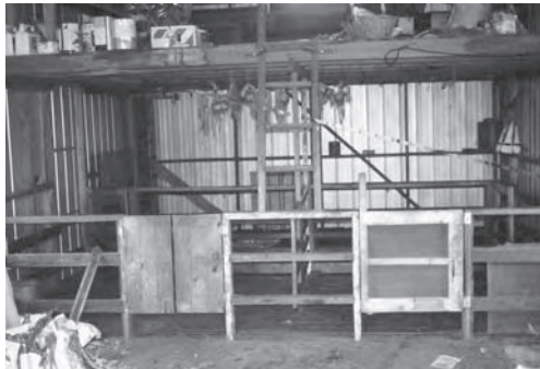
Multipurpose shed – shearing plant attaches to central bracket, catching pen (right), count-out pen (left).
