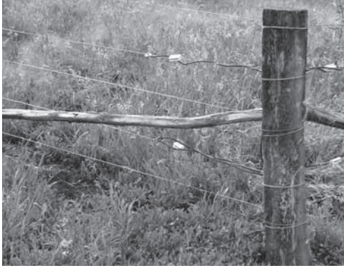
Electric fence – alternating earth and hot wire, hardwood posts.
