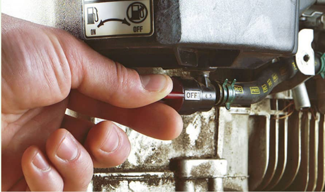
Fuel line problems—For more information, shown here
