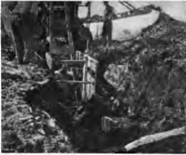
FIG. 91.—Movable Sheet piling Fastened to Traction Ditcher.
