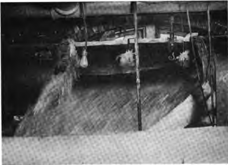
FIG. 45.—Overflow Weir in Action.
