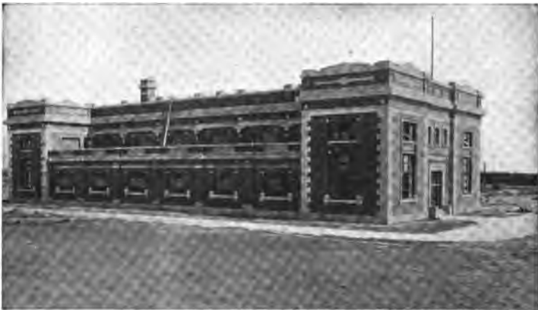
FIG. 49.—Calumet Sewage Pumping Station, Chicago, Illinois.
