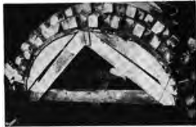
FIG. 127.—Centering for Brick Sewer.
