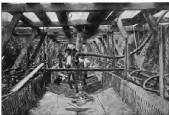
FIG. 100.—Well Points Pumped by Nye Steam Vacuum Pump.
