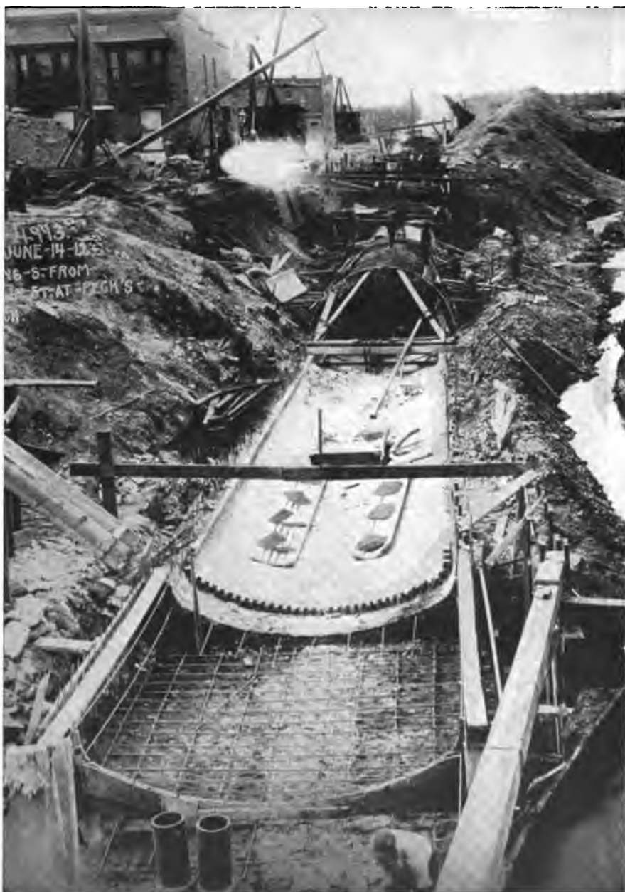
FIG. 1.—Construction of Peck's Run Sewer, Baltimore, Maryland.
