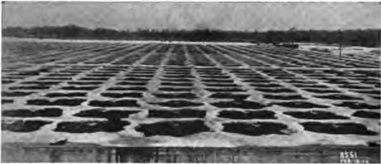
FIG. 167.—Sprinkling Filter in Operation in Winter at Baltimore.
