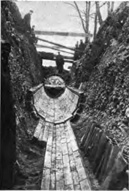
FIG. 128.—Segmental Block Sewer at Clinton, Iowa.
