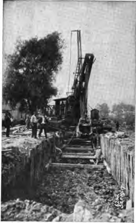
FIG. 93.—Steam Shovel at Work on Sewer Trench for North Shore Intercepting Sewer, Evanston, Illinois.
