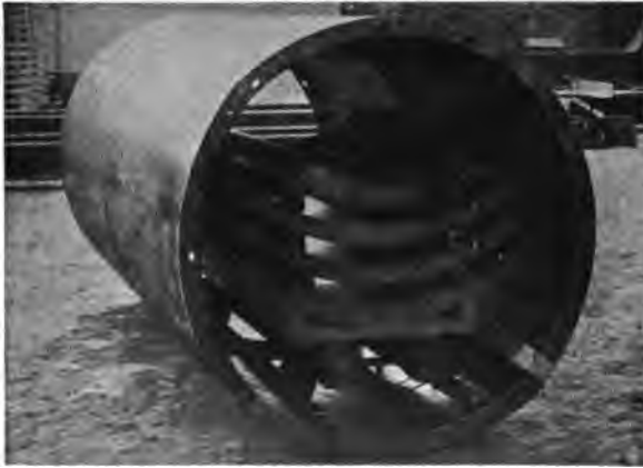
FIG. 138.—Blaw Standard Full Round Telescopic Sewer Forms, Showing Knocked-Down Sections Loaded on a Truck.
