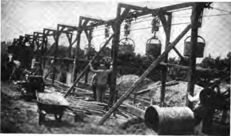
FIG. 92.—Carson Excavating Machine on Trench Excavation in South Milwaukee.
