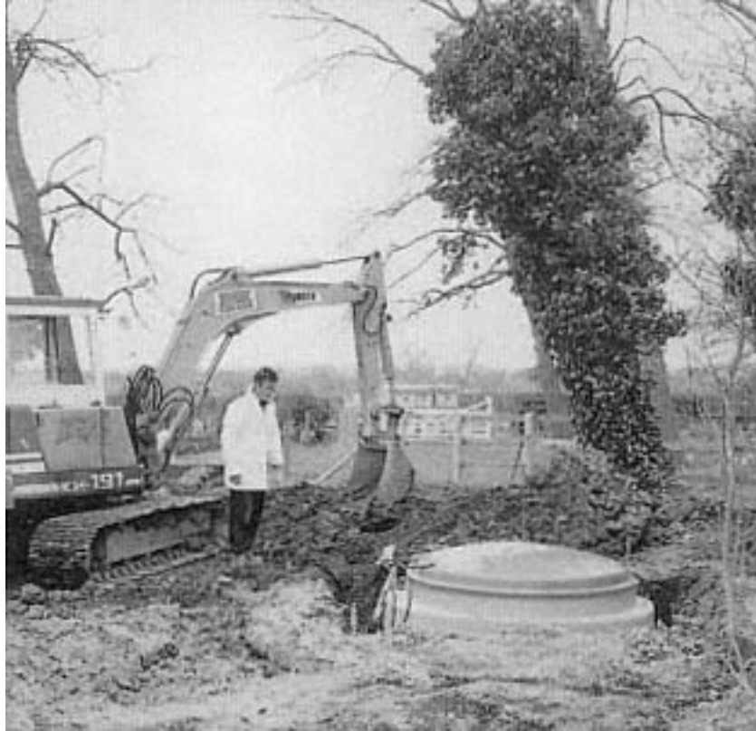
Figure 6.2 A 5 pe rbc being installed.
