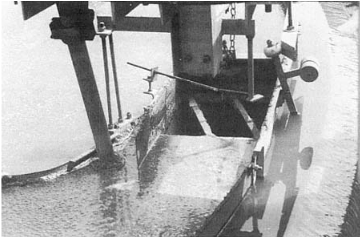
Figure 2.8 Scum box mechanism.
