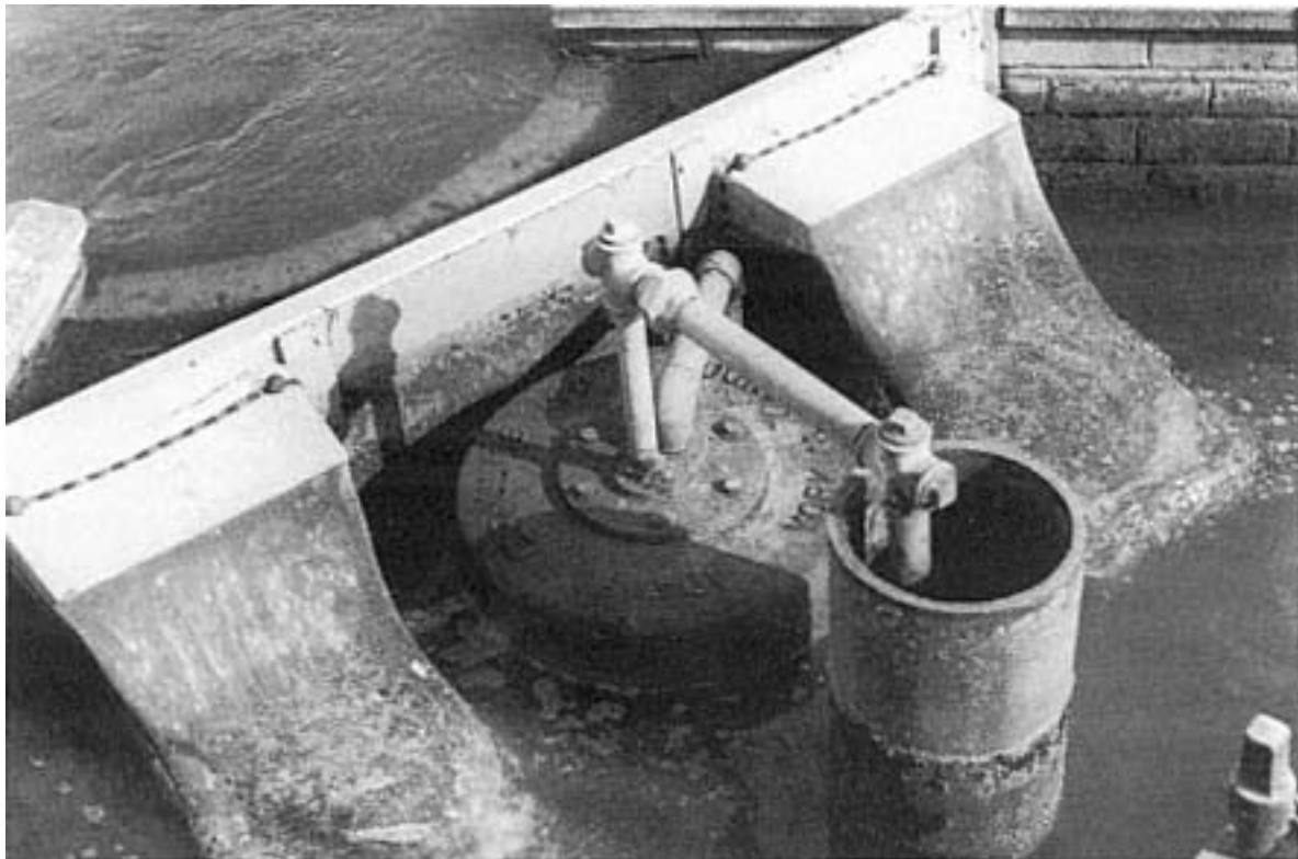
Figure 1.1 Copa sack installation on a weir.
