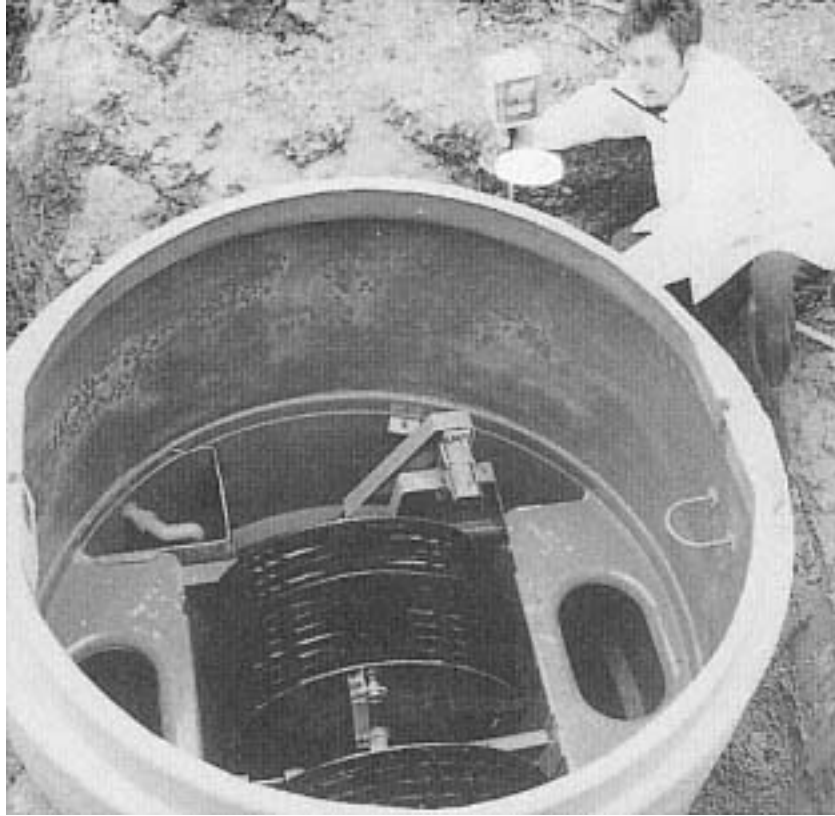
Figure 6.7 Small biodisc or rbc plant.
