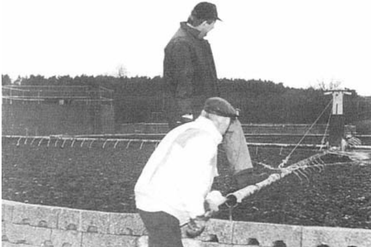
Figure 4.4 Rodding out a filter arm.
