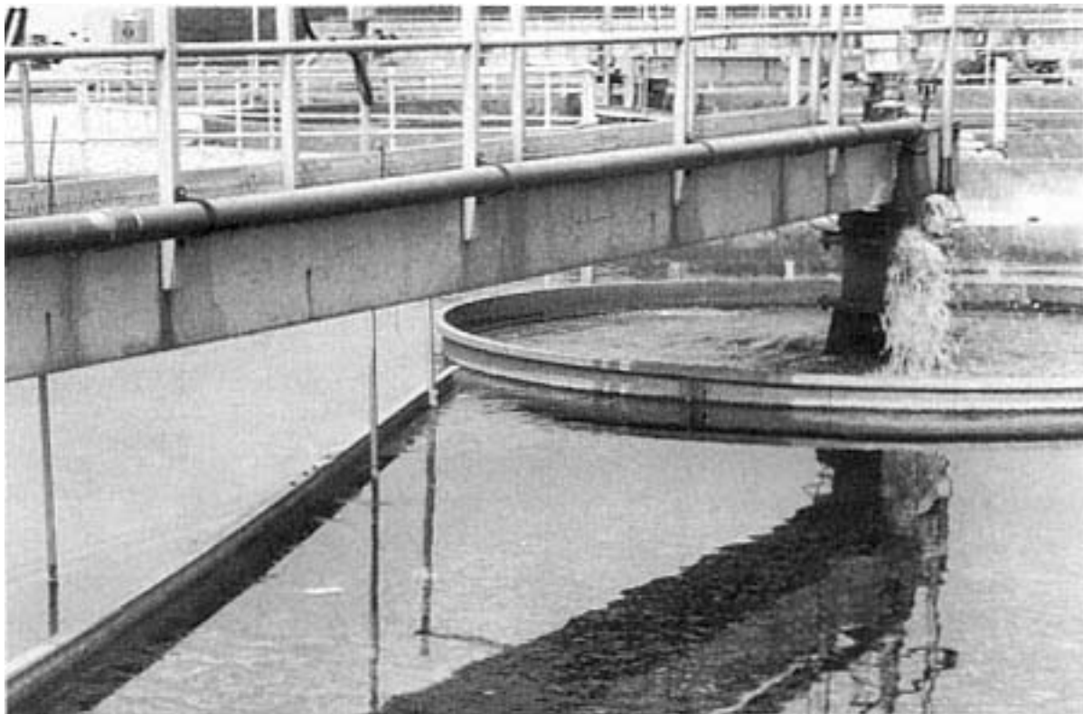
Figure 1.2 Surface pump and plastics skimming trap.
