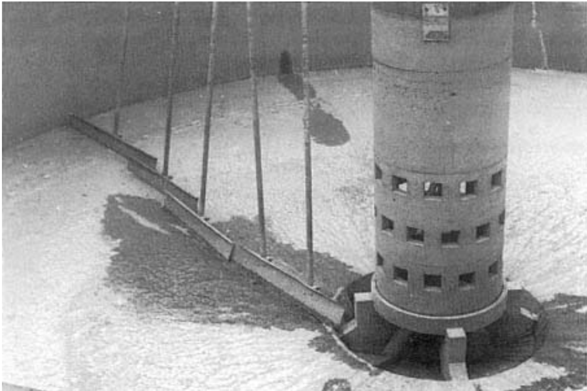
Figure 2.6 Continuous scraper blades sedimentation tank.
