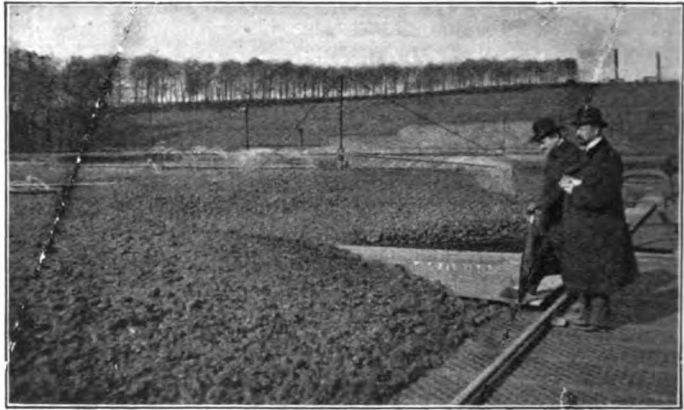
FIG. 101.—Whittaker and Bryant Sprinkler at Accrington.
