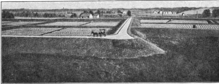
FIG. 83.—Furrows on the Surface of Filters.
