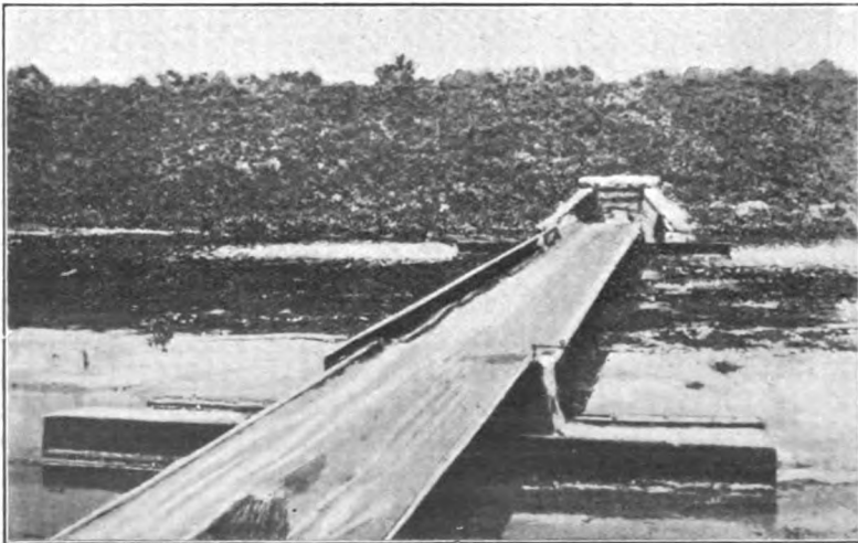
FIG. 82.—Distribution of Sewage in Filters.
