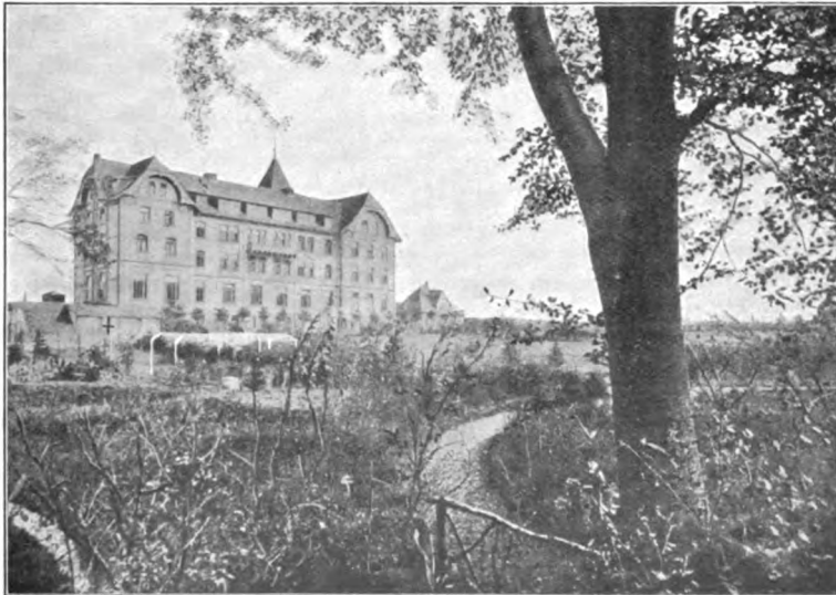
FIG. 136.—General View, showing Comparative Size of Biological Sewage Works for a Sanatorium.
