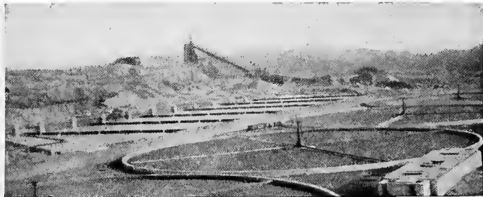
FIG. 124.—Revolving distribution on trickling filters at Pontiac, Mich.
