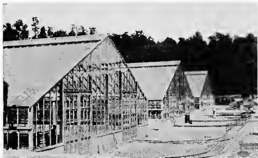
FIG. 200.—Glass-covered sludge-drying beds at North Toronto plant, Toronto, Ont.
