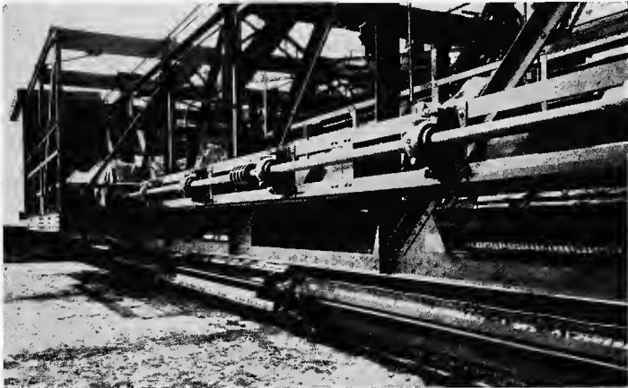
FIG. 205.—Longitudinal type of sludge-stripping machine at West Side works, Chicago.
