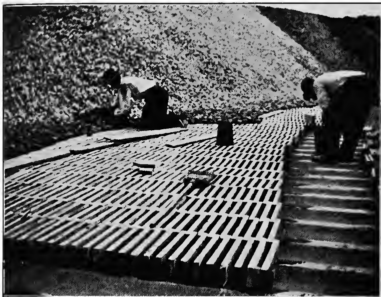
FIG. 146.—Constructing trickling-filter floor, Fitchburg, Mass.
