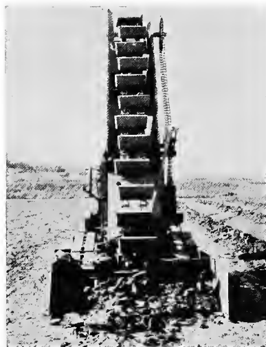
FIG. 204.—Machine used in stripping sludge from drying beds at Worcester, Mass.
