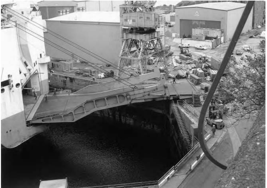
Car carrier – Vehicle Ramp. Angled vehicle ramp seen deployed from the Grimaldi Car Carrier, 'Republic Di Genova'. The scene is shown in Falmouth Dry Dock, where the vessel was booked in for routine maintenance.
