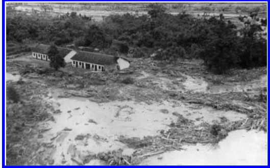
Figure 5. Destruction in the dock area and Packing House of English Farm after the debris flow of March 1967.
