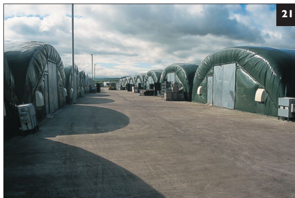
21 Plastic covered insulated tunnels, the cheapest form of structure for producing the crop.
