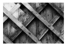
Figure 10.22. Mould growth on untreated larch wood panels and battens.
