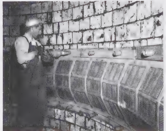
FIGURE 8-6. Strainer being installed in a brick-lined digester (Esco).
