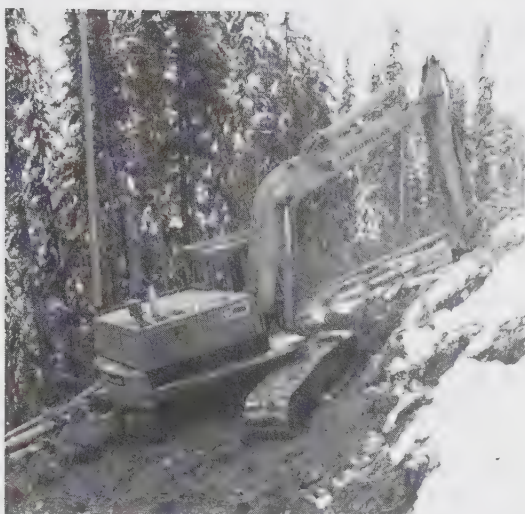
FIGURE 3-8. Clearing for a logging road in the Northwest (photo by Finning).
