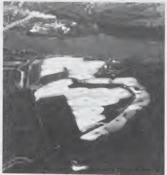
FIGURE 26-10. This aeration stabilization basin utilizes 27 40-hp aeration units, and provides five days of retention (Aqua Aerobic System).
