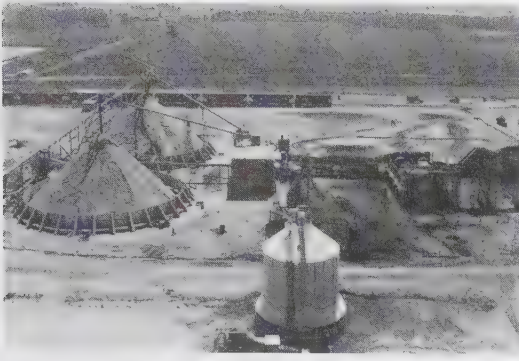
FIGURE 3-34. Part of a woodyard showing two open-type chip storage and reclaim systems. A closed bark bin is shown in the foreground (Atlas Systems).
