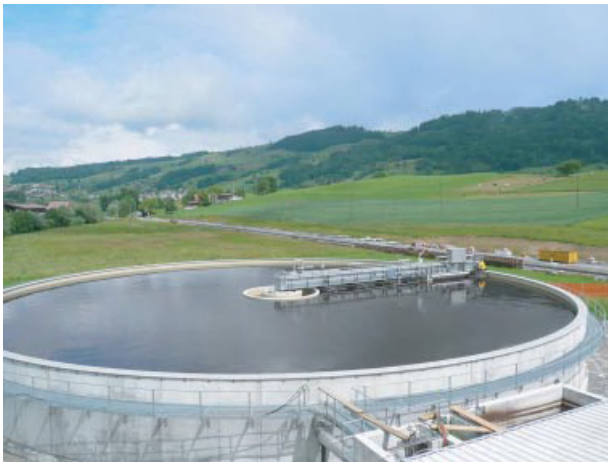
Figure 9.37 Circular sedimentation clarifier.
