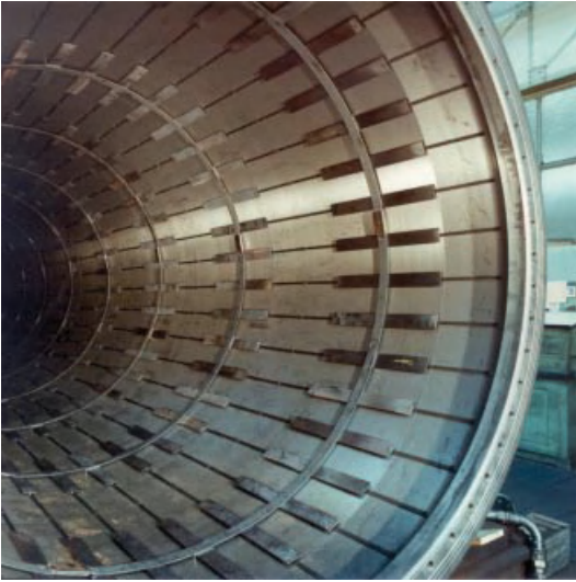
Figure 16.5 View inside a drying cylinder equipped with spoiler bars. (Source: Voith.)
