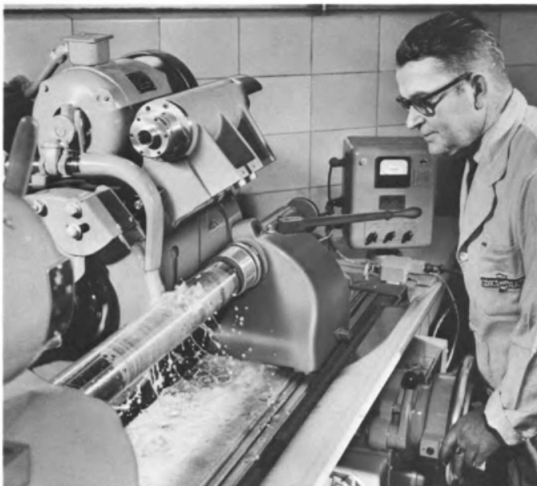
Fig. 1-6. Principle of cylindrical grinding, "traverse" method.
