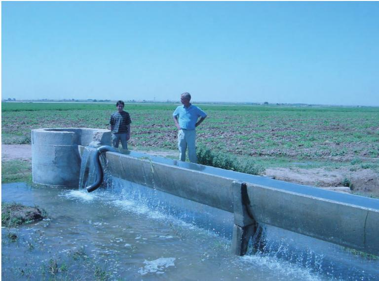
**Fig. 5.5** In the distribution system the misdistribution of water usually exceeds seepage
