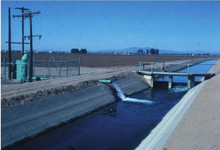
**Fig. 5.10** Pumping groundwater into the (downstream) part of the conveyance systems improves the operational flexibility and control of the groundwater table
