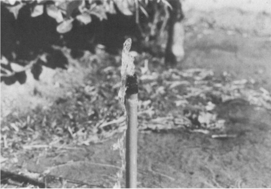
Fig. 1.1.8 Bubbler system with a small basin around each tree to contain the high water application rate.
