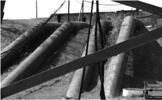
FIGURE 6 Repression pipes (Floating pumping station) [3].
