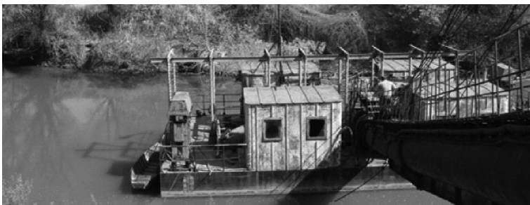
FIGURE 5 Ship of floating pumping station on Mures River [3].
