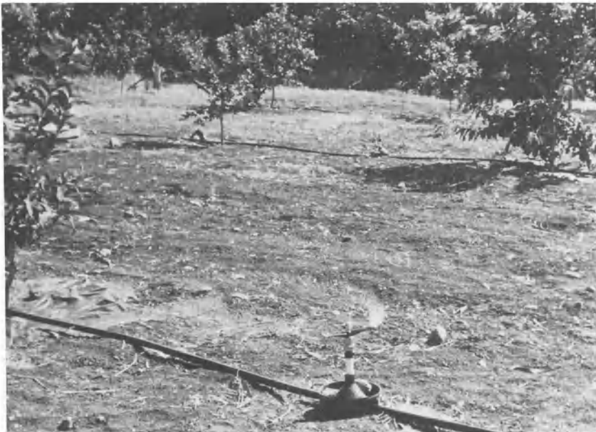
B. Orchard Sprinkler on Hose-pulled Skid
