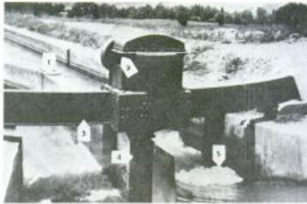
FIGURE 4-12. - Flow divisor (Neyrpic), Oned Fodda network, Algeria. 1. Flap hinge. 2. Control gear. 3. Flap positioning. 4. Movable flap. 5. Hydraulic jump. (69)
