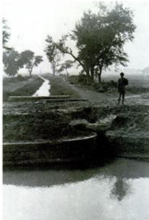
FIGURE 5-19. - General view of an AOSM outlet to a farm watercourse (Haryana, India).
