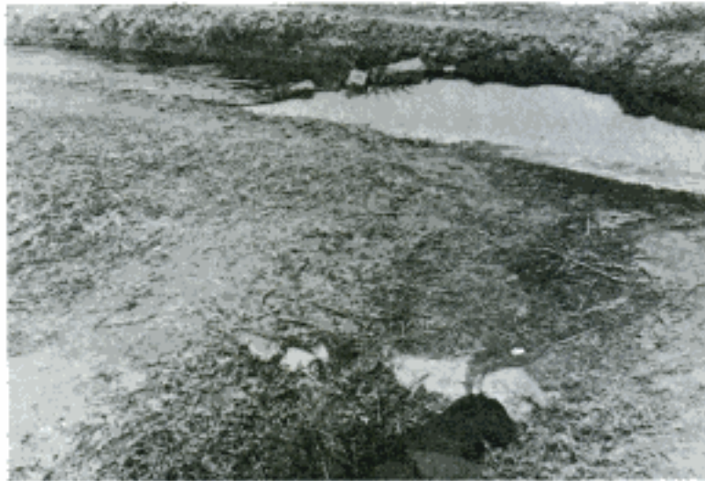
FIGURE 2-4. - Example of tampering. Brush and stone dam built by farmers across a minor irrigation canal to increase flow through a pipe outlet.
