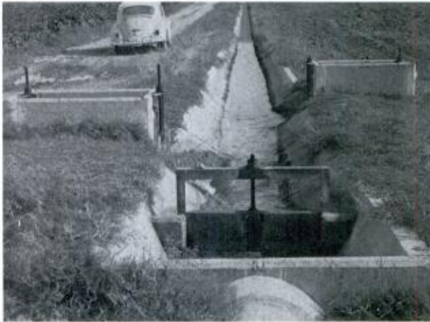
FIGURE 3-7. - Constant-head orifice farm turnouts with check-gate in foreground - East Ghor Canal Project, Jordan.
