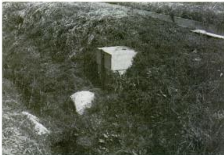
FIGURE 5-50. - Prefabricated gated outlet (Ferrara type).
