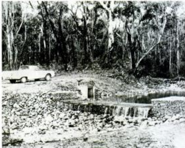
FIGURE 3-32. - General view of the stone mesh weir and inlet box. (Almost all the flow - 12 \text{ ft}^3/\text{s} - is being diverted.)
