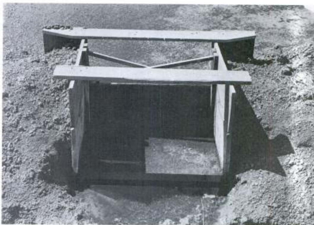
FIGURE 5-60. - Wooden outlet for basin or border irrigation.
