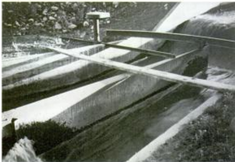
FIGURE 4-8. - Flow divisor with adjustable splitter, Argentina.
