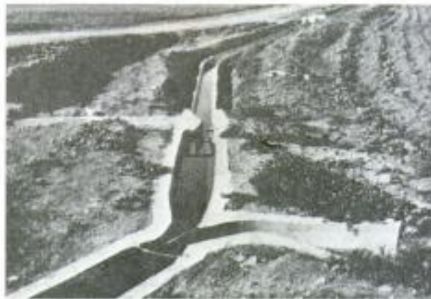
FIGURE 4-13. - Three-way distribution by means of two consecutive flow divisors. (69)
