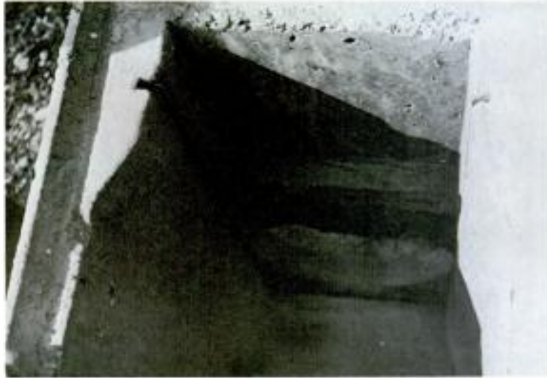
FIGURE 5-52. - Prefabricated gated outlet (Ferrara type).
