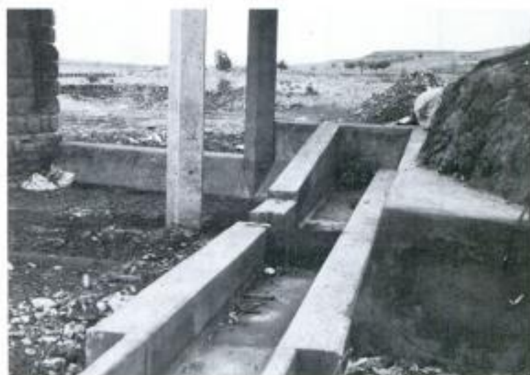
FIGURE 3-39. - Photograph of groyne intake structure (Cyprus).
