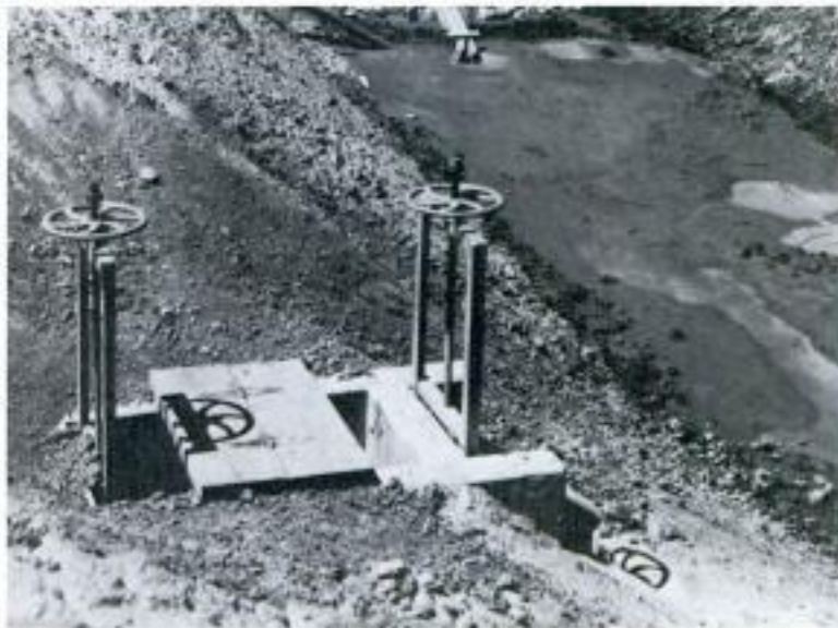
FIGURE 3-8. - A single-barrel constant-head orifice turnout.
