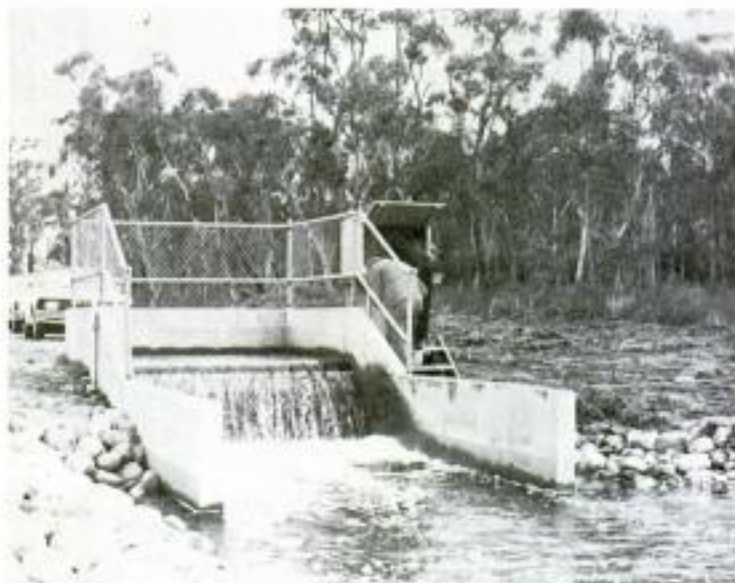
FIGURE 3-35. - Dissipation structure and measuring weir at the pipe outlet. (Discharge 10 \text{ ft}^3/\text{s} .)
