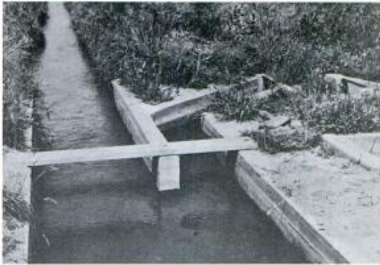
FIGURE 4-2. - Simple fixed proportional flow divisor of low accuracy.
