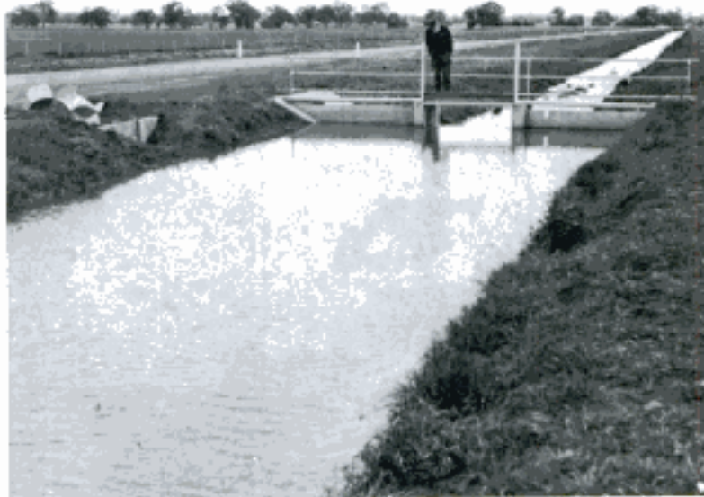
FIGURE 5-6. - Typical setting of Dethridge meter just upstream of a regulator. The supply level of the canal is indicated by the bottom of the slot in the wall on the right hand side of the regulator.
