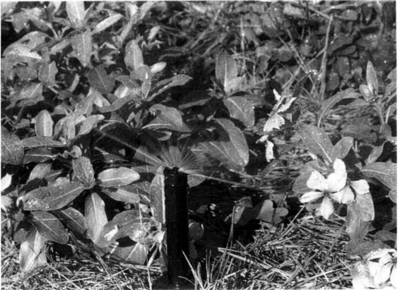
FIGURE 30.6B Micro-spray adapter and nozzle cap attached to 570 body.
