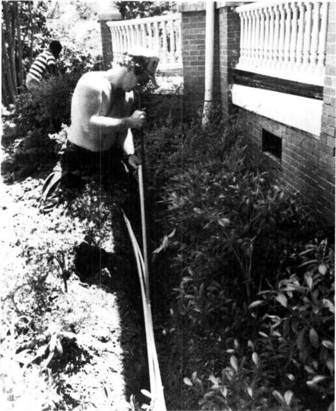
FIGURE 7.1 C Trench in a shrub bed dug by hand.
