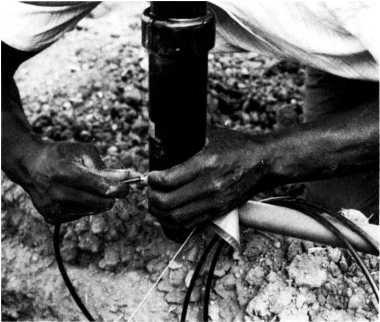
FIGURE 15. 1 Hydraulic tubing being connected to a valvein-head sprinkler.
