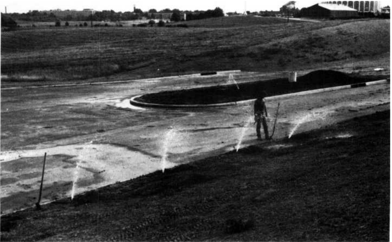
FIGURE 7.4 Flushing pipe lines.
