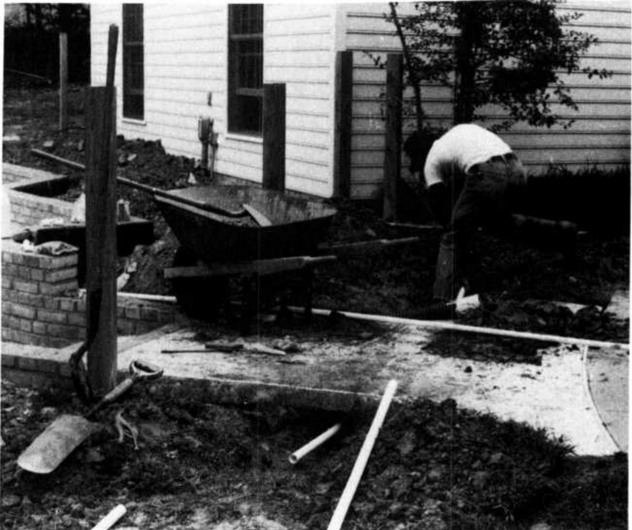
FIGURE 17. 1 Schedule 40 pipe sleeve beneath walk.
