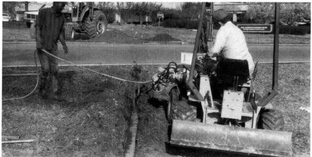
FIGURE 7.19 Boring beneath roadways.
