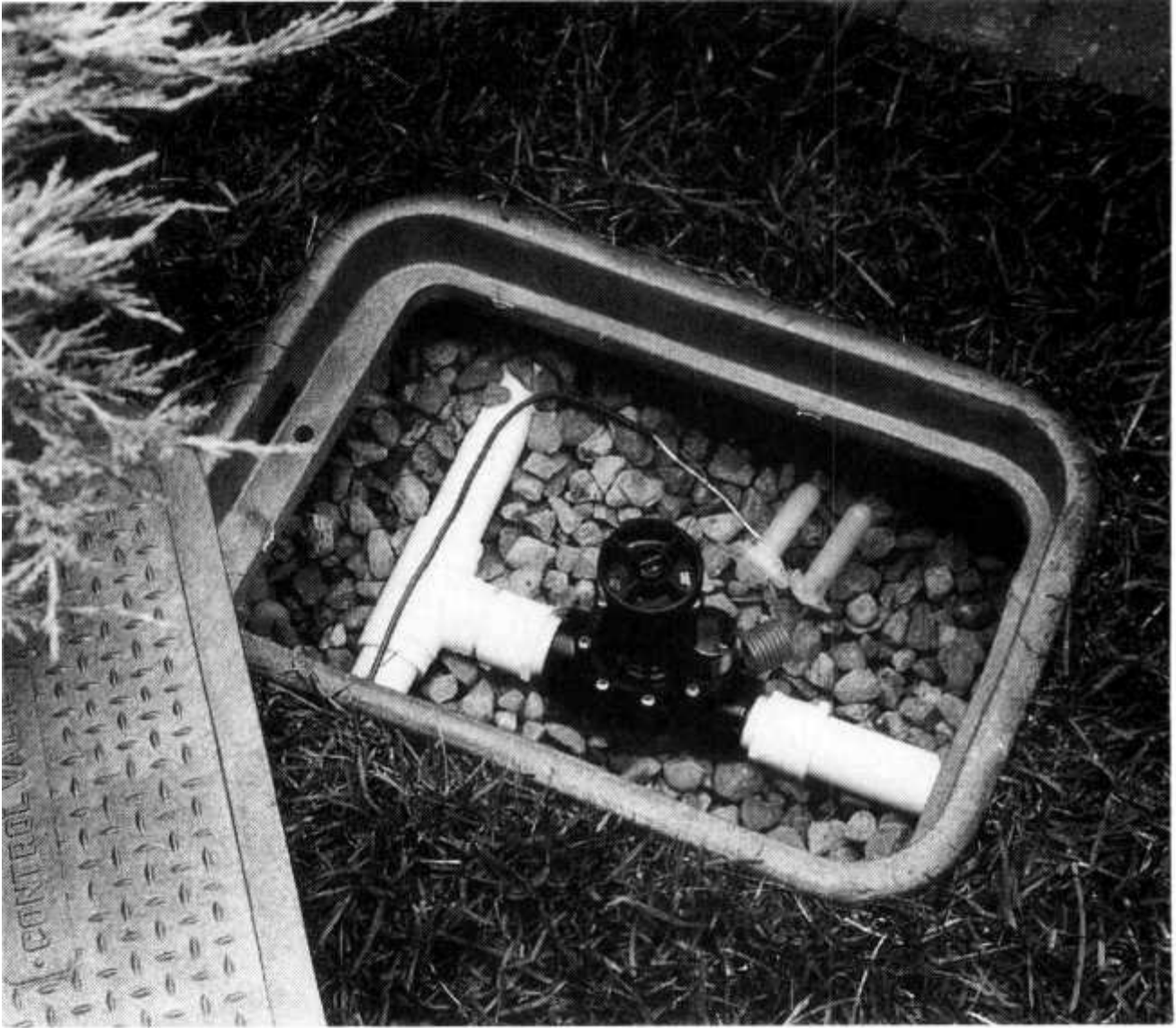
FIGURE 12.2 Valve with solenoid and wire splice caps. (Source: The Toro Company. Used with permission.)
