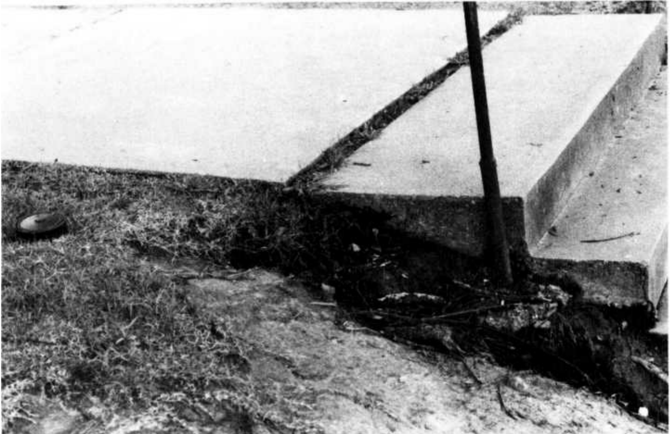
FIGURE 9.11 Low head drainage.
