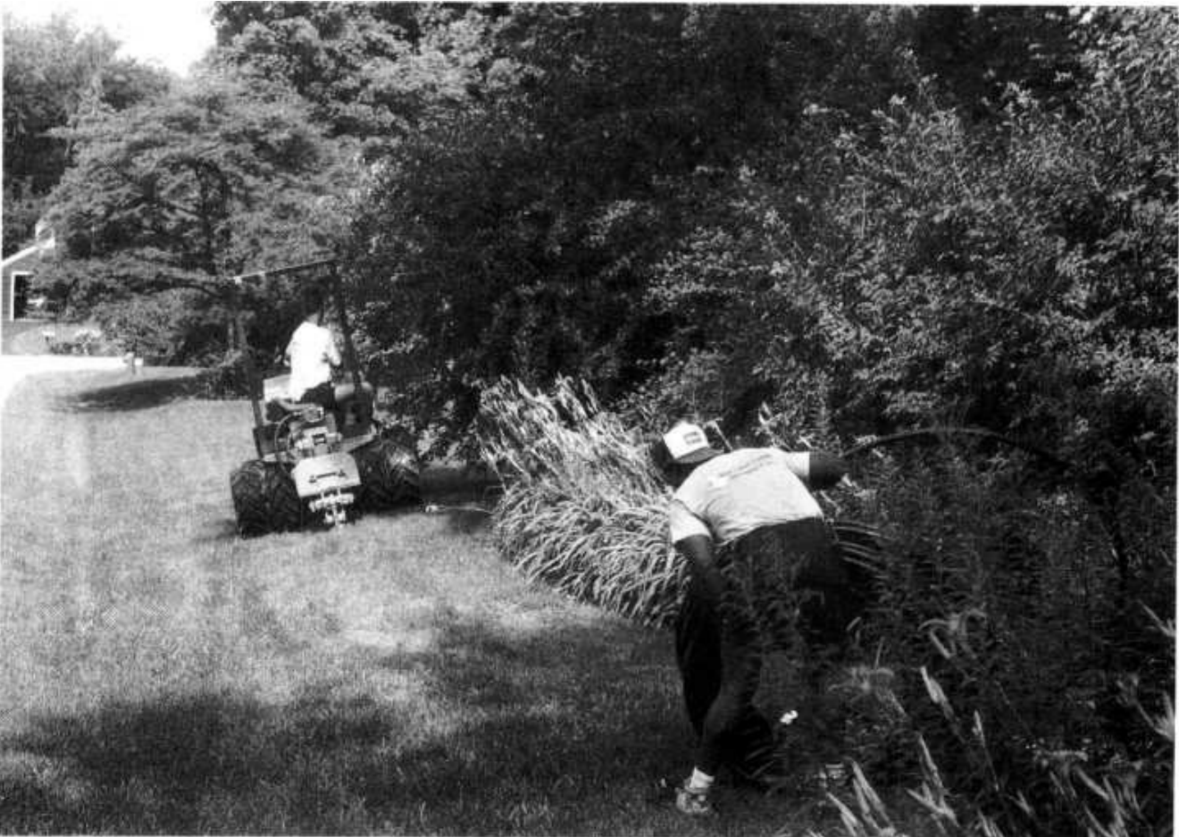
FIGURE 7.6C Attaching PE pipe to plow.
