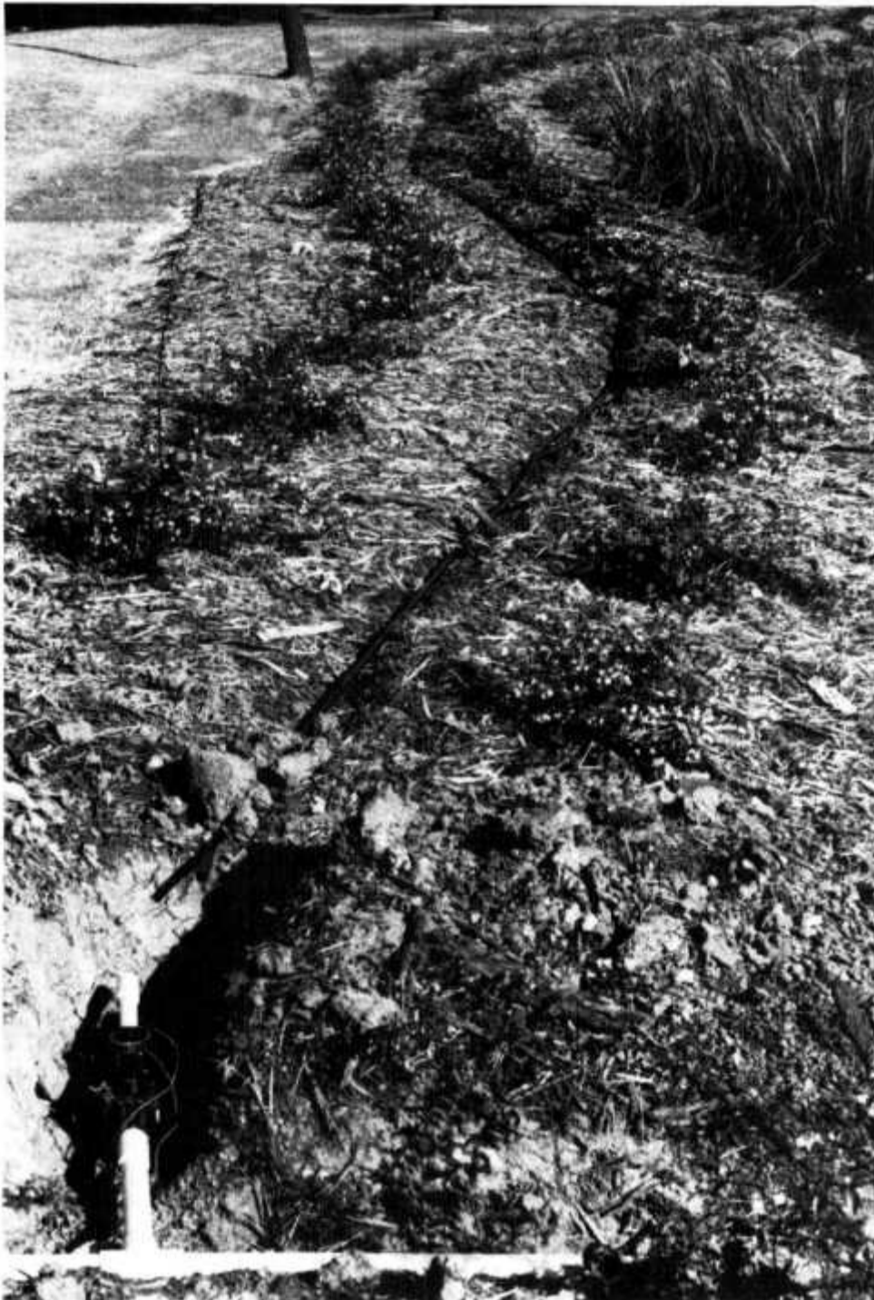
FIGURE 33.8 Drip tubing running parallel with slope.
