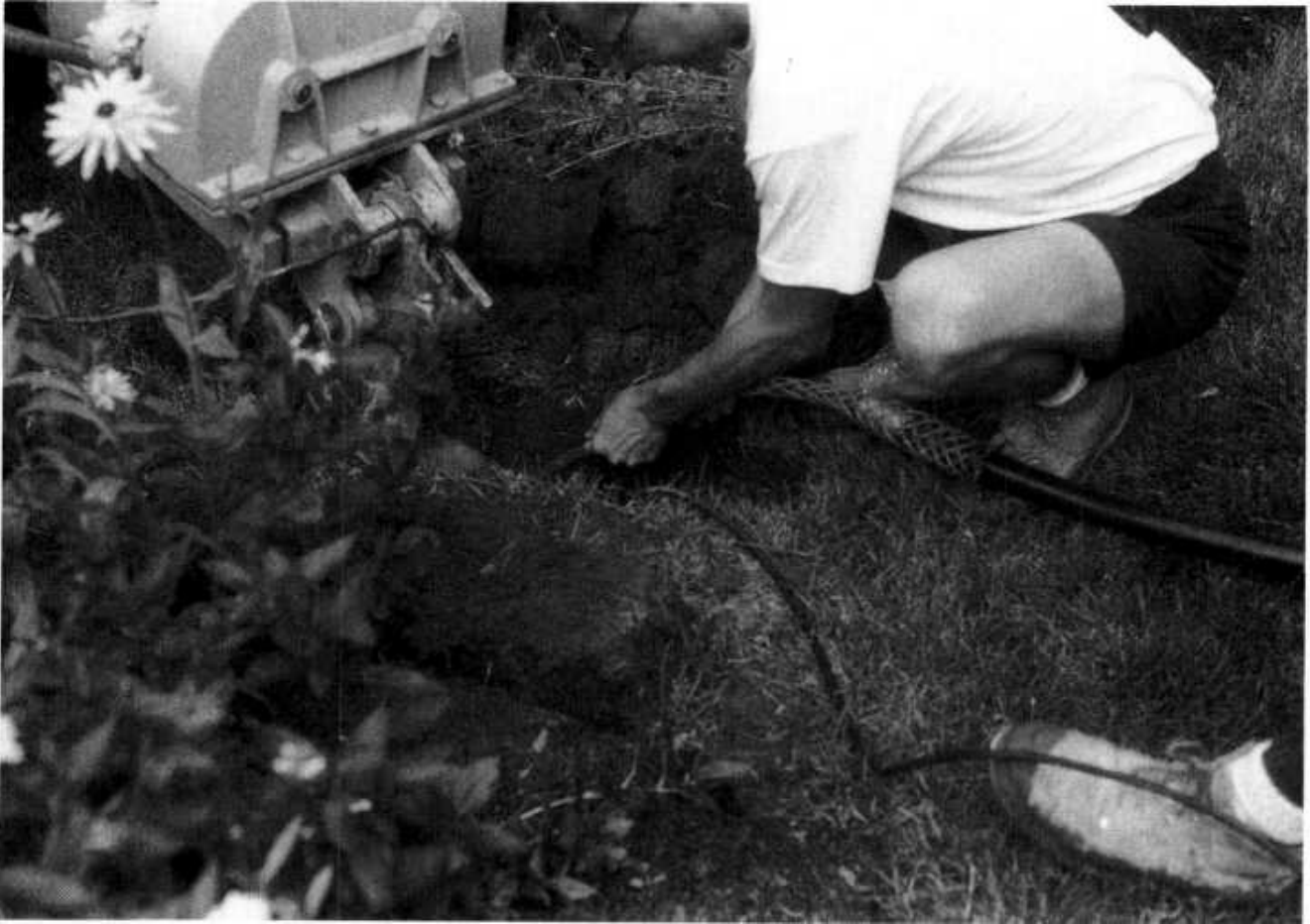
FIGURE 7.6C Attaching PE pipe to plow.
