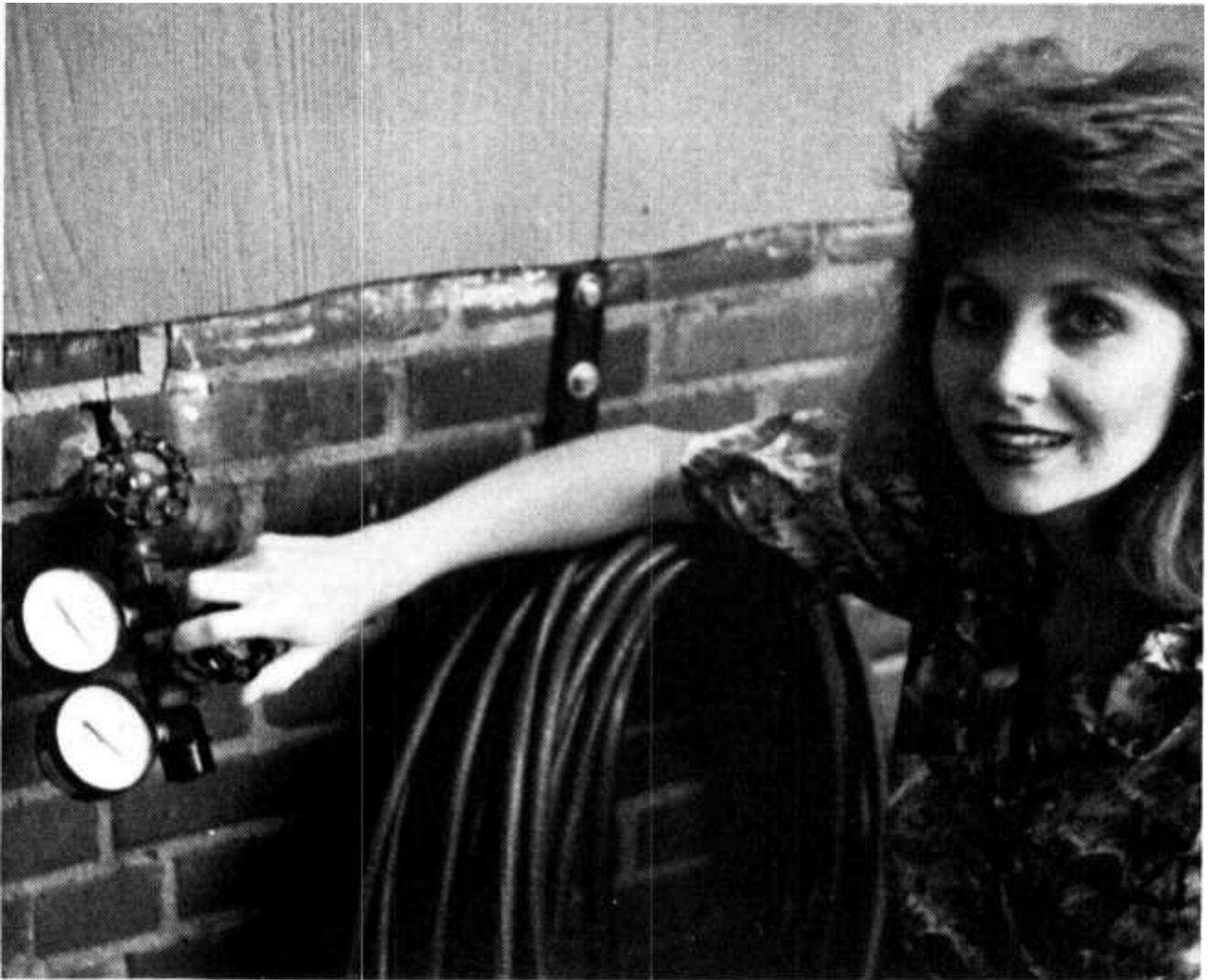
FIGURE 33.2 Reading water pressure at hose bib.
