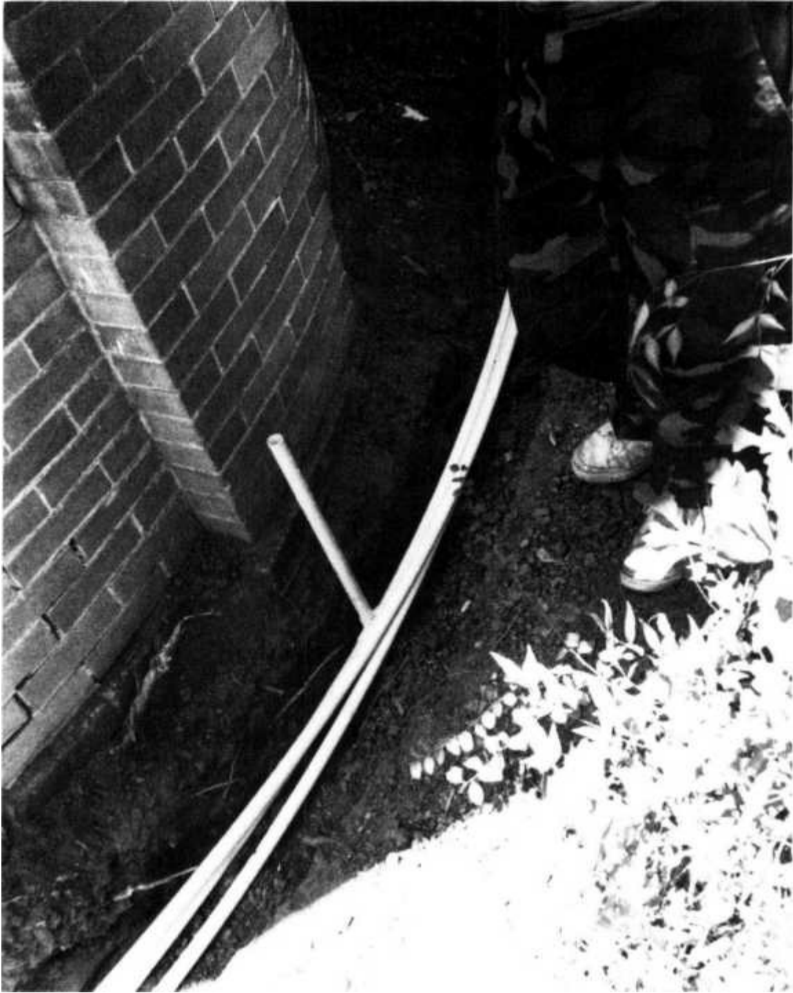
FIGURE 7.1 A Trench dug by hand next to a building.
