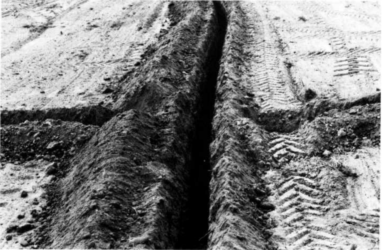
FIGURE 7.12 Cross-trenching.
