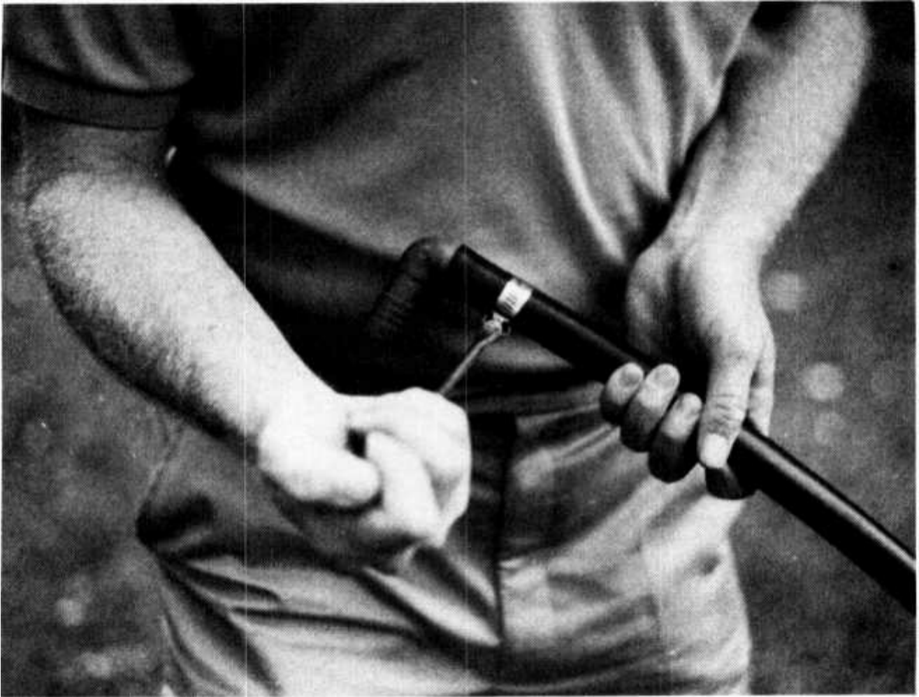
FIGURE 17.5 Attaching stainless steel clamp.
