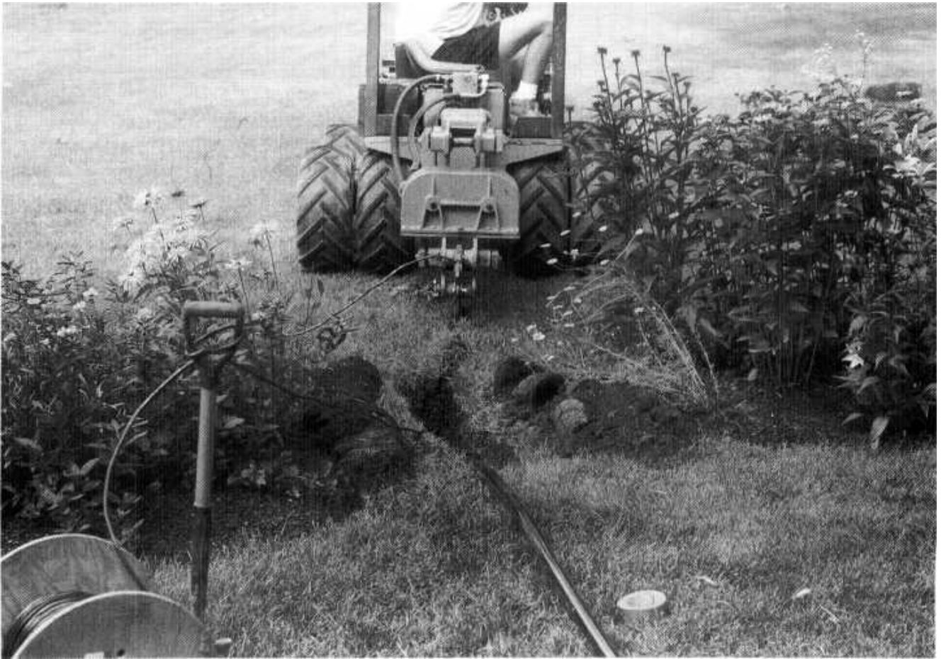
FIGURE 7.6B Tractor and vibratory plow pulling PE pipe.
