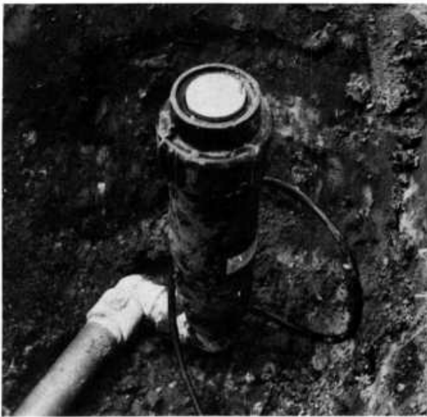
FIGURE 29.3 Valve-in-head sprinkler and swing joint.
