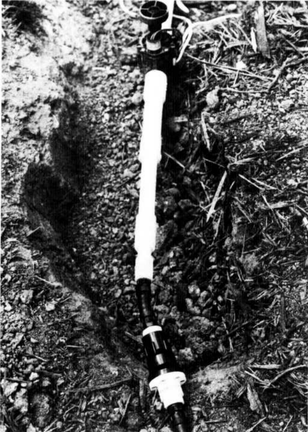
FIGURE 9. 10 Valve and pressure regulator.
