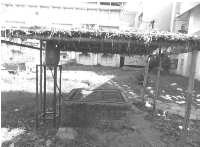
FIGURE 7.7 ZECC with micro-dripper system under gravity flow.
