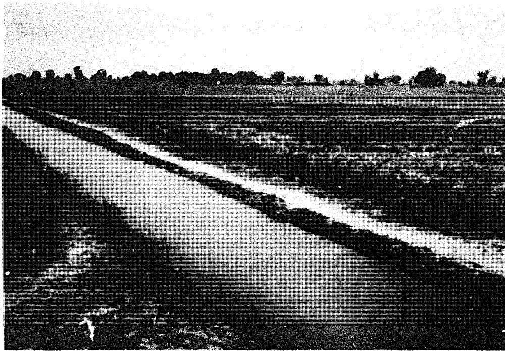
Irrigation supply channel.
